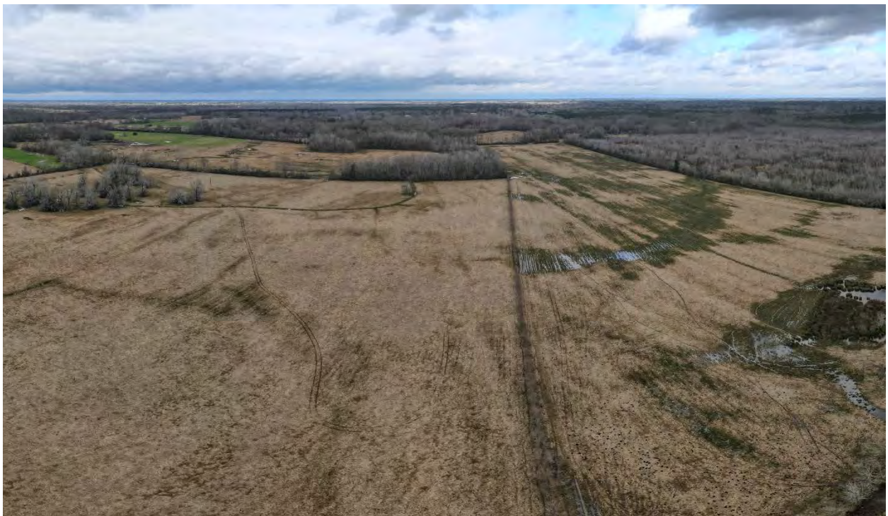
Photo 8: Overview of site from center of Phase 2, facing north.
