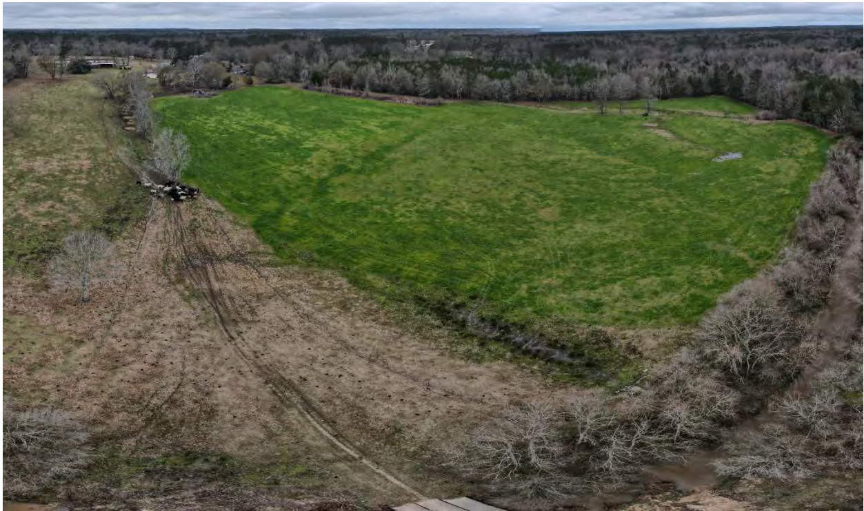
Photo 3: Overview of site from center, facing north.
