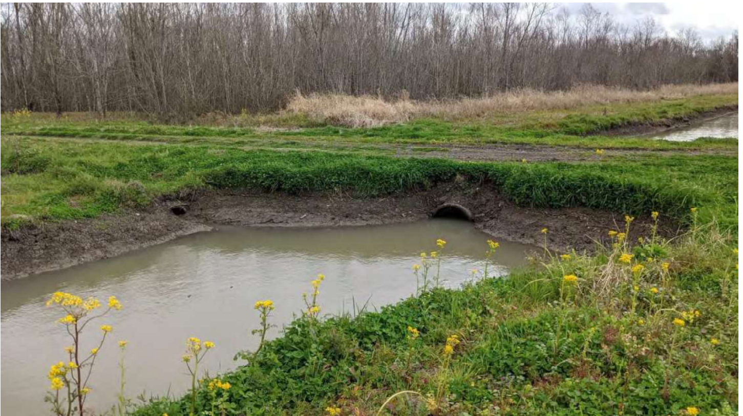
Figure 12: Typical Culvert and Elevated Dirt Road Found on Site
