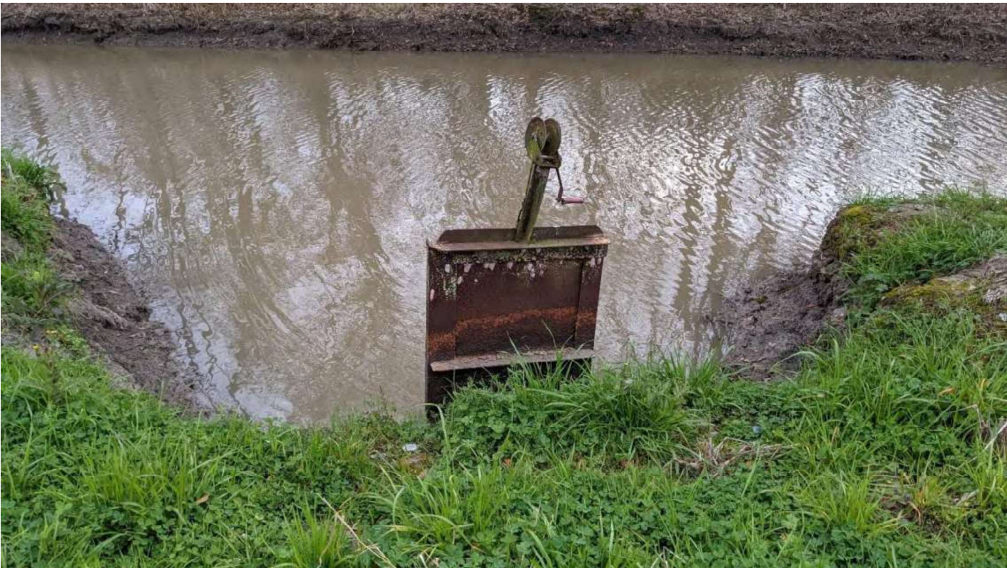
Figure 08: Typical Slide Gate Structure Located at the Intersection of the “Southern Slide Gate Canal” and “Unnamed Agricultural Canal”
