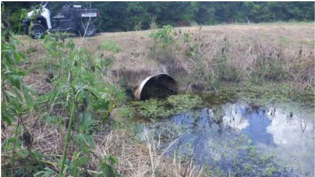
Typical drainage features currently used for water management (May 23, 2018)
