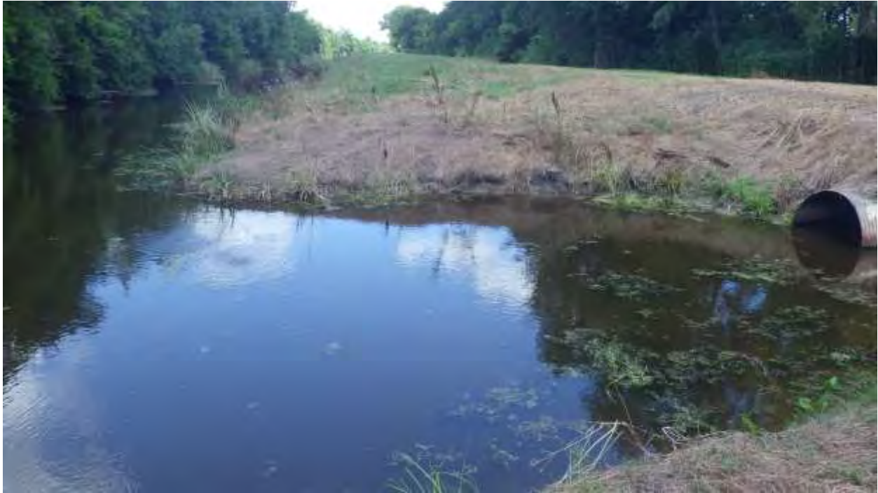
Typical drainage features currently used for water management (May 23, 2018)
