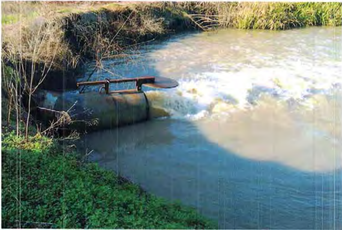
Pumping station gated discharge.
