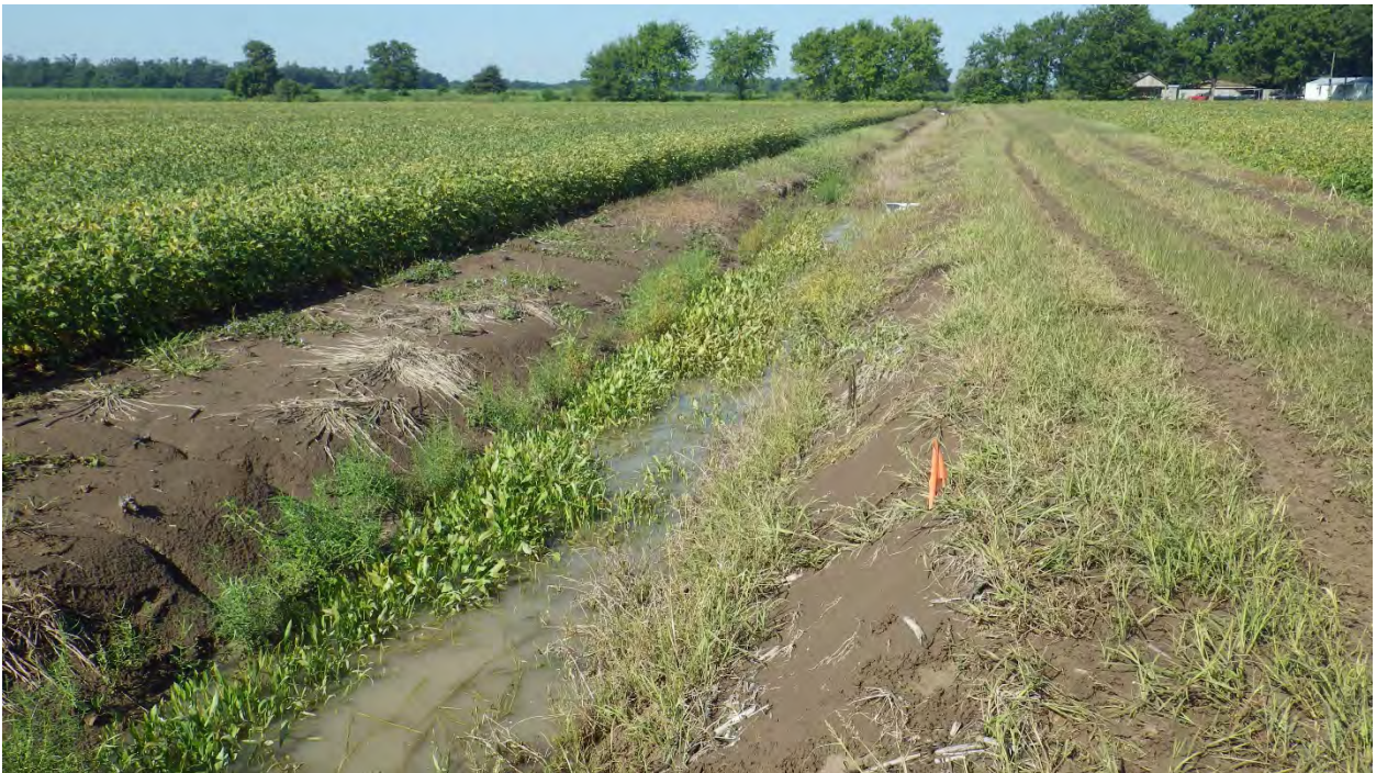
View of typical interior agriculture drain to be filled
