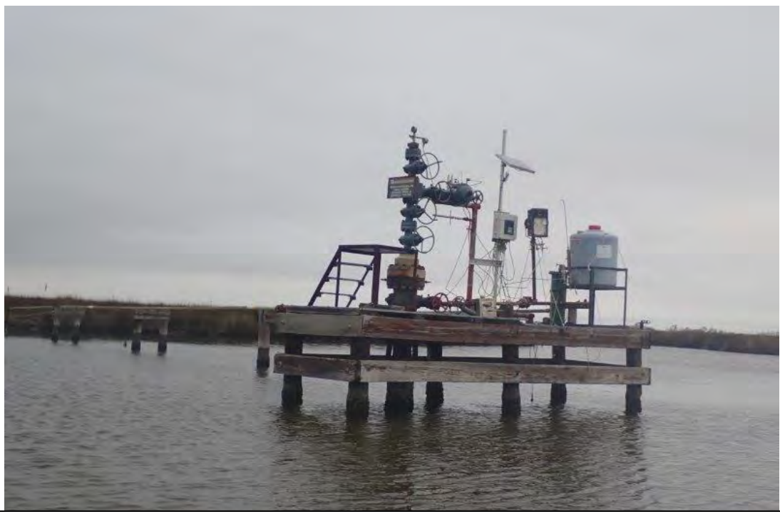
Photograph 145. Site 40: Well Platform (29°35'40.39"N, 90°1'37.96"W)
