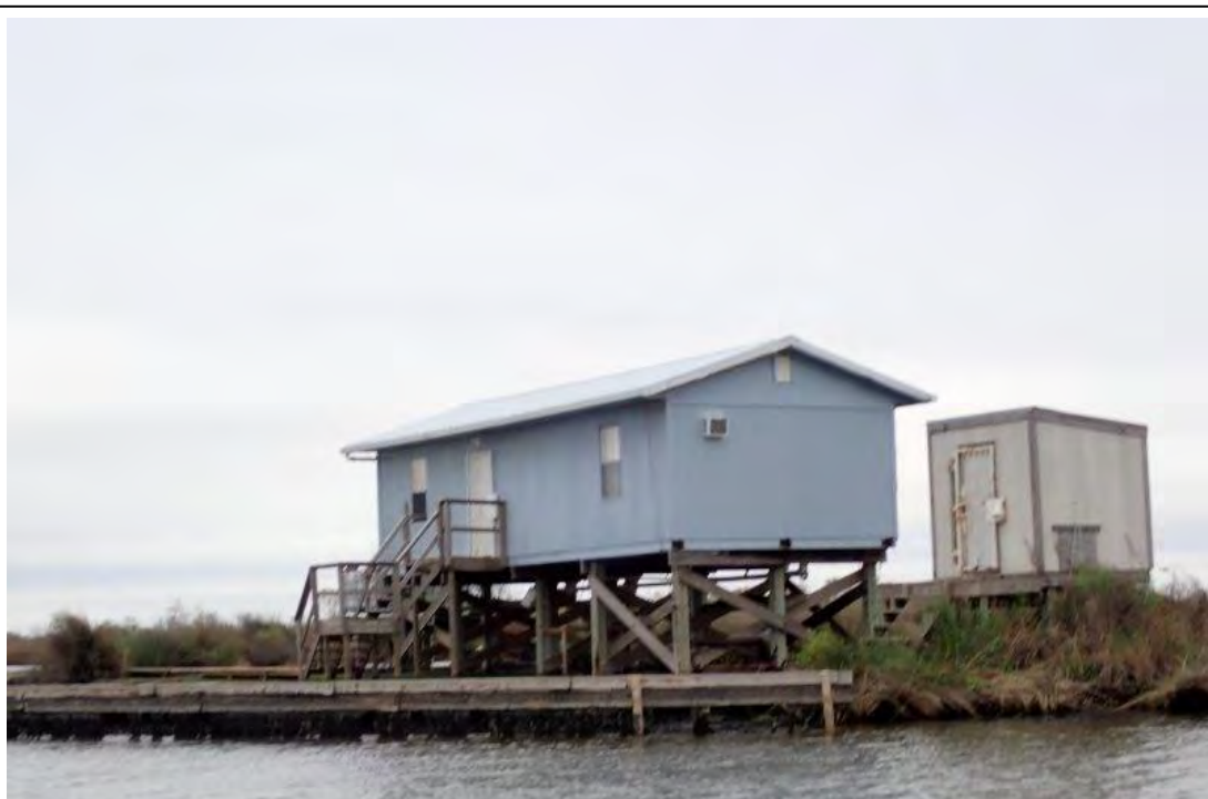
Photograph 130. Site 30: Camp Structure (29°33'49.25"N, 90°3'51.96"W)
