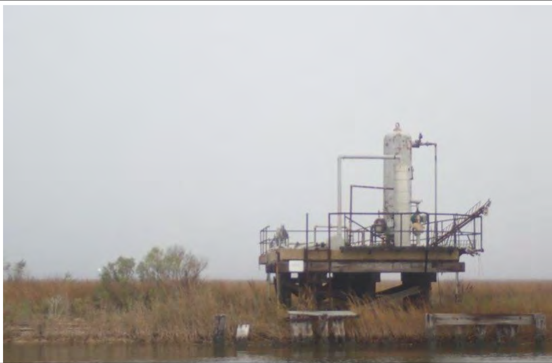
Photograph 109. Site 18: Oilfield Condensate Structure
