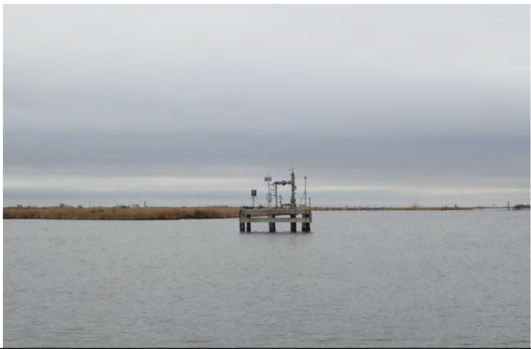
Photograph 135. Site 32: Oil Field Facility Structures
