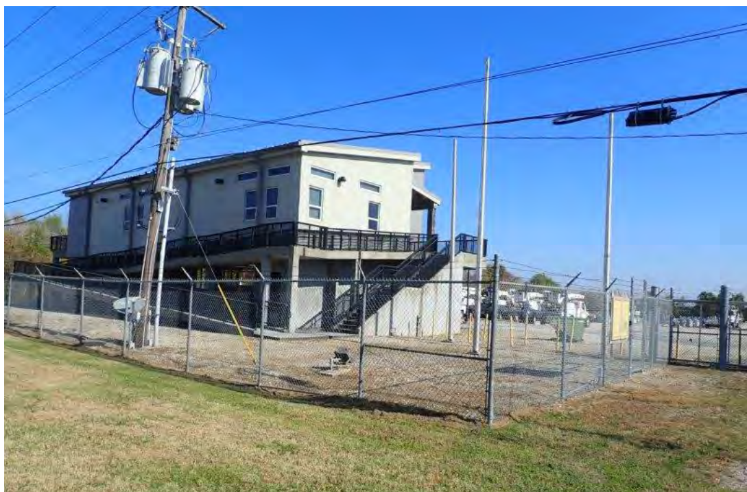
Photograph 78. Entergy Office and Yard (29°39'49.52"N, 89°58'30.50"W)
