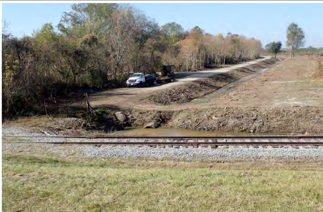
Photograph 8. Overview of Mississippi River Levee Area 2 Facing West
