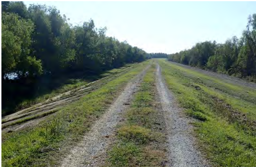
Photograph 7. Overview of Mississippi River Levee Area 2 Facing South
