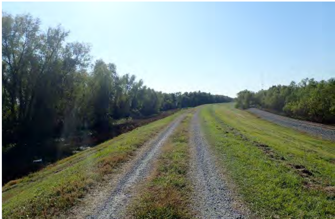
Photograph 3. Overview of Mississippi River Levee Area 1 Facing South
