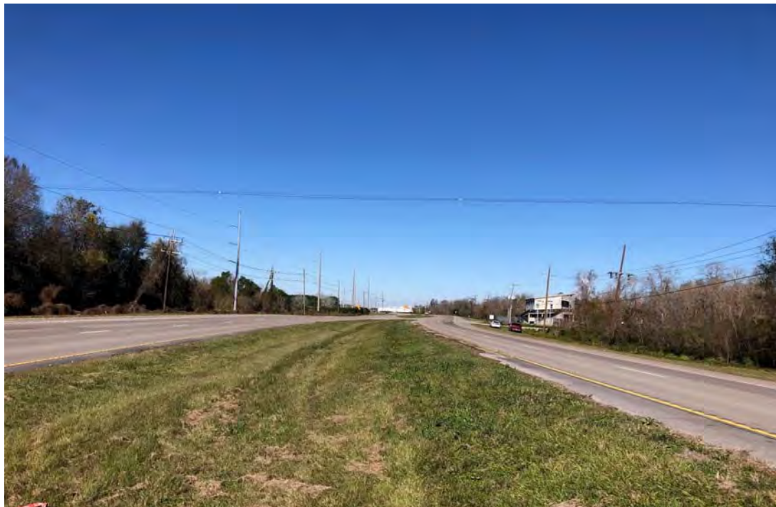
Photograph 33. Overview of Highway Area 3 Facing North (29°39'43.14"N, 89°58'31.14"W)
