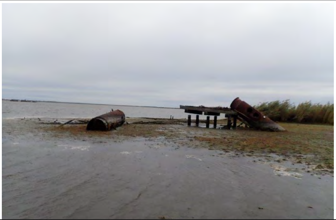
Photograph 89. Site 2: Damaged Oil Field Facility
