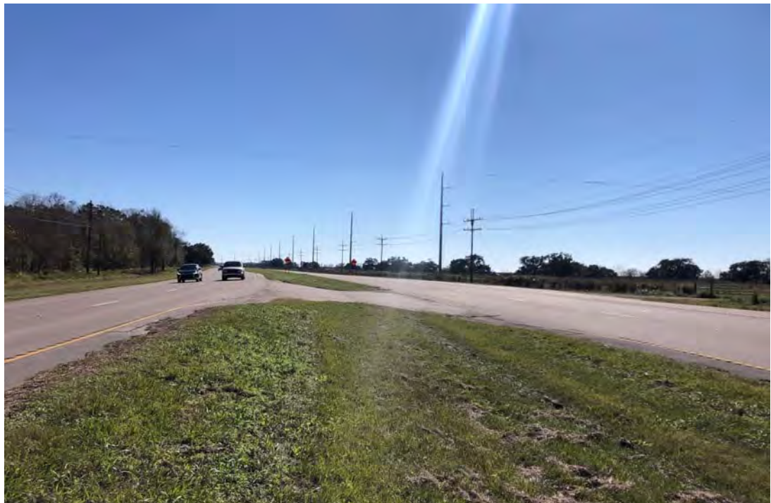
Photograph 35. Overview of Highway Area 3 Facing South
