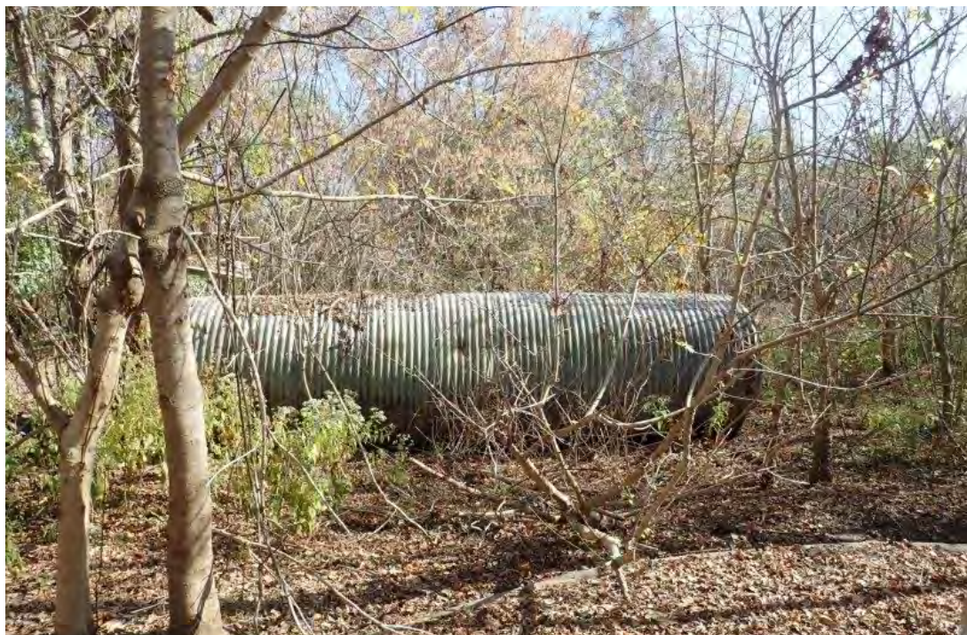
Photograph 70. Galvanized Pipe Adjacent to Silo Pad
