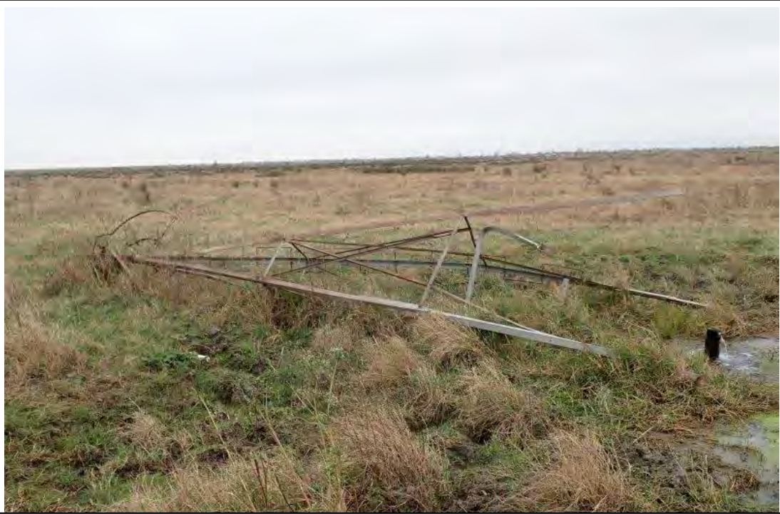
Photograph 81. Collapsed Windmill with Flowing Water Well (29°39'5.16"N, 89°58'32.10"W)
