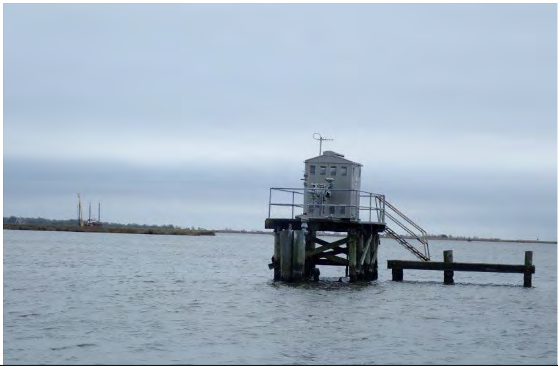
Photograph 125. Site 27: Oil Field / Pipeline Metering Platform (29°32'40.15"N, 90°3'36.20"W)
