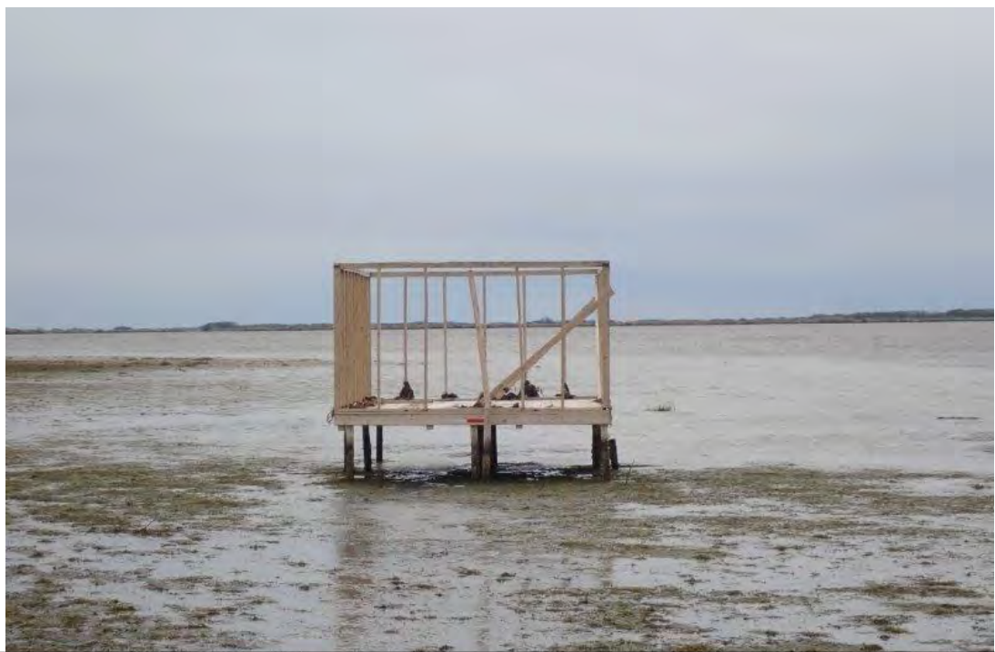
Photograph 83. Partially Constructed Camp (29°38'35.02"N, 90°0'6.35"W)
