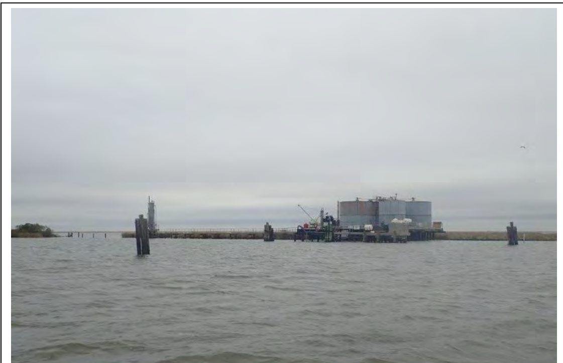
Photograph 122. Site 25: Oil Field Tank Battery with Flare Unit (29°32'21.78"N, 90°3'5.60"W)
