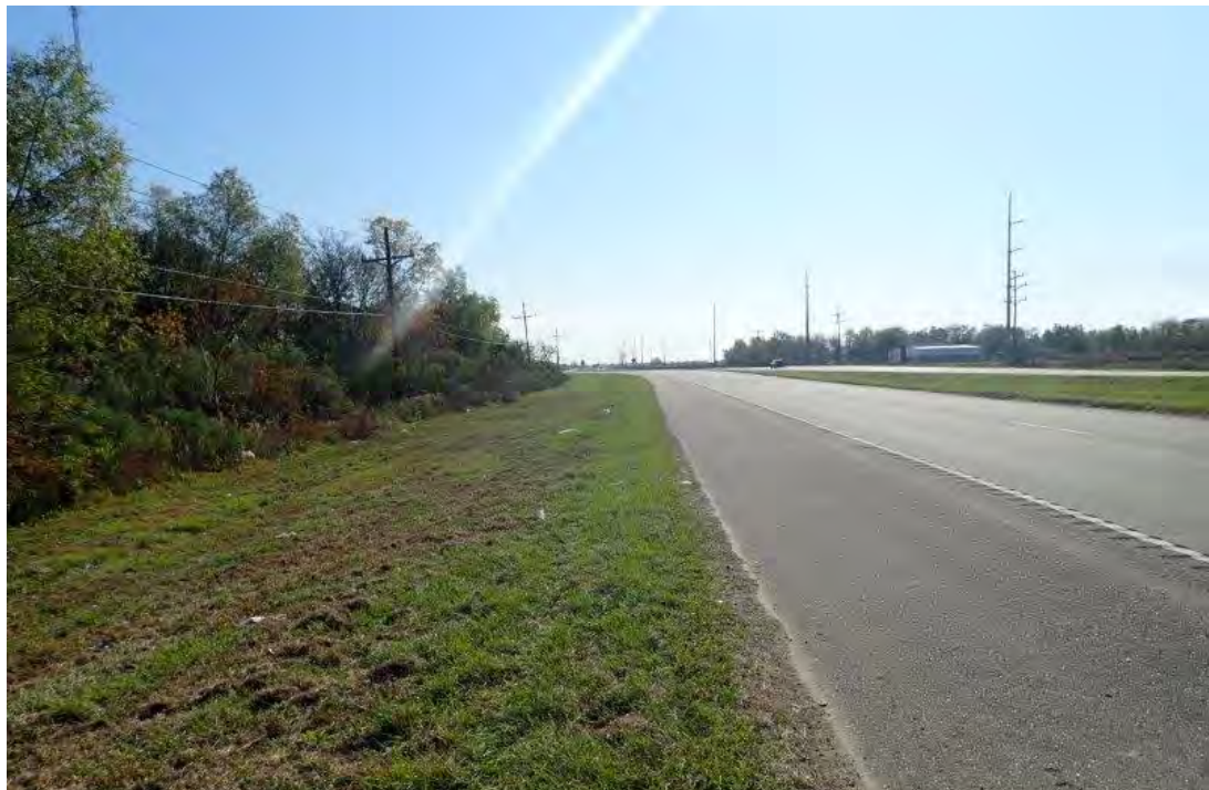
Photograph 27. Overview of Highway Area 1 Facing South
