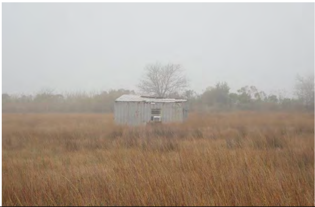
Photograph 105. Site 15: Displaced Camp Structure (29°31'44.24"N, 89°54'15.17"W)
