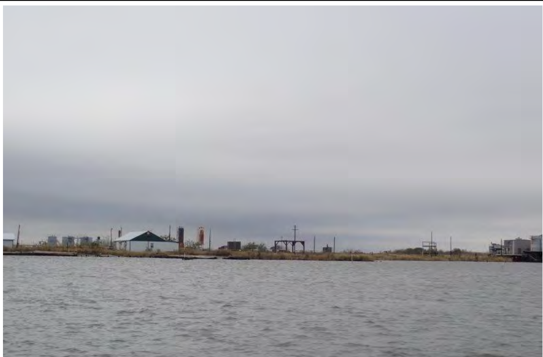
Photograph 136. Site 32: Oil Field Facility Structures
