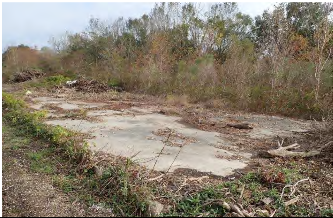
Photograph 75. Concrete Slab (29°39'48.70"N, 89°58'22.97"W)
