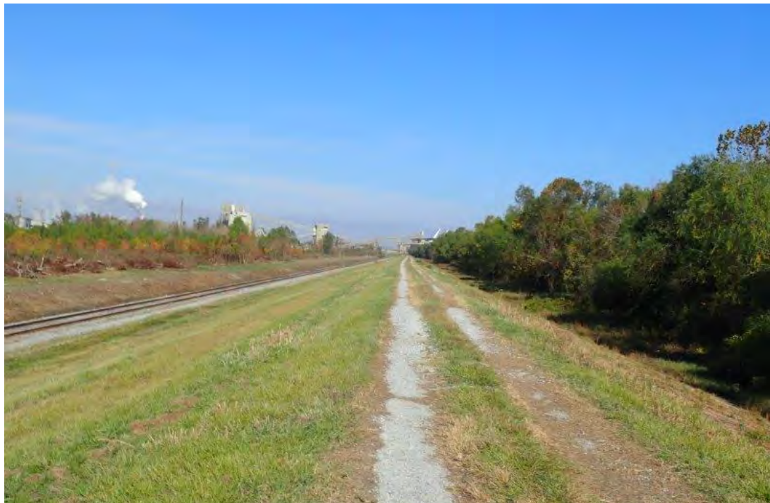
Photograph 5. Overview of Mississippi River Levee Area 2 Facing North (29°39'49.83"N, 89°57'48.43"W)
