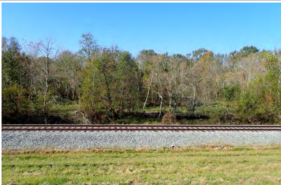
Photograph 4. Overview of Mississippi River Levee Area 1 Facing West
