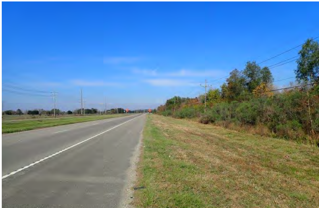
Photograph 25. Overview of Highway Area 1 Facing North (29°39'1.44"N, 89°58'5.58"W)
