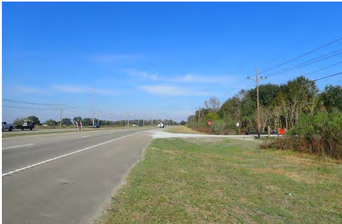
Photograph 29. Overview of Highway Area 2 Facing North (29°39'14.22"N, 89°58'15.60"W)
