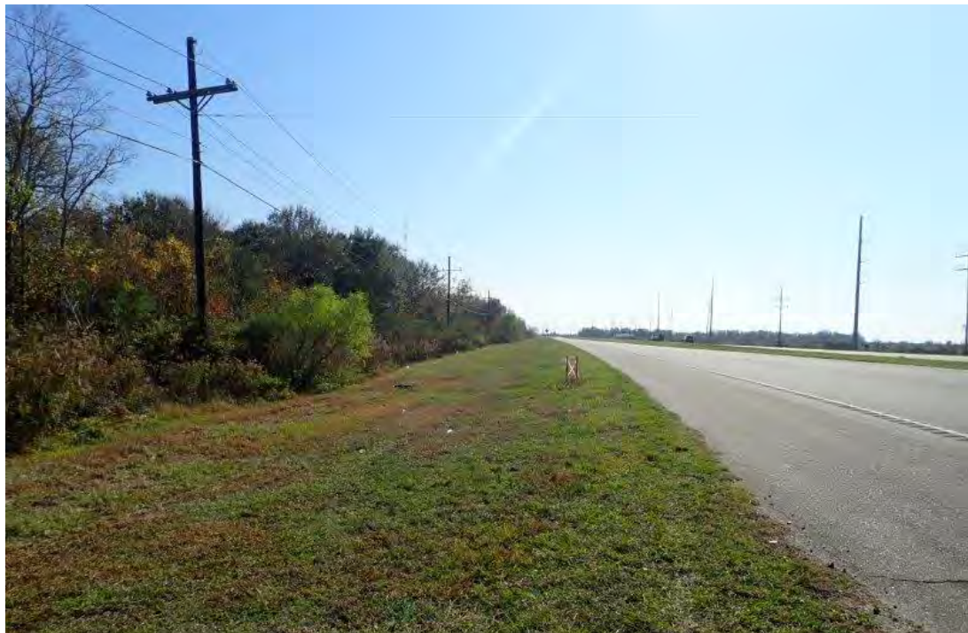
Photograph 31. Overview of Highway Area 2 Facing South
