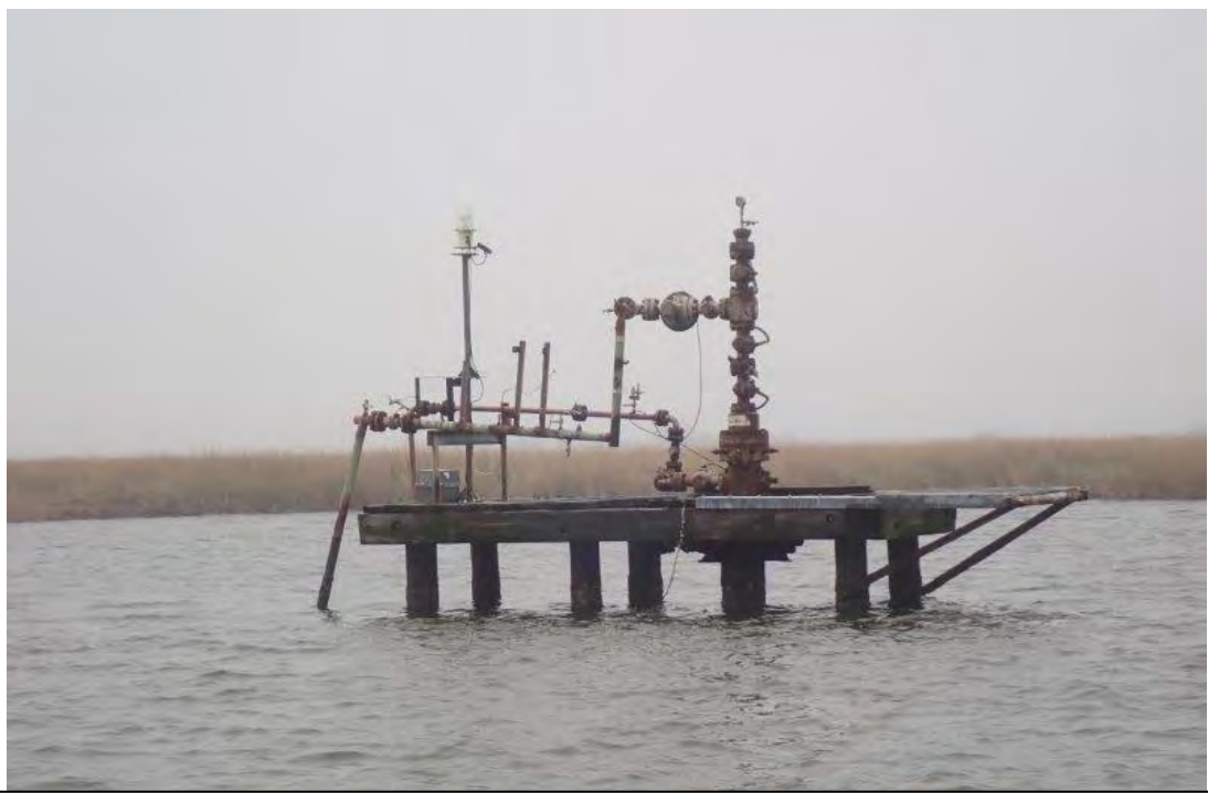
Photograph 107. Site 17: Well Platform (29°32'19.86"N, 89°54'22.60"W)
