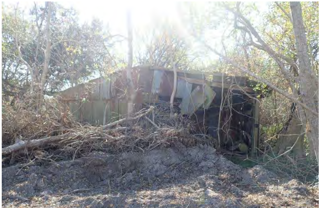
Photograph 63. Abandoned Shed (29°39'49.56"N, 89°57'55.61"W)
