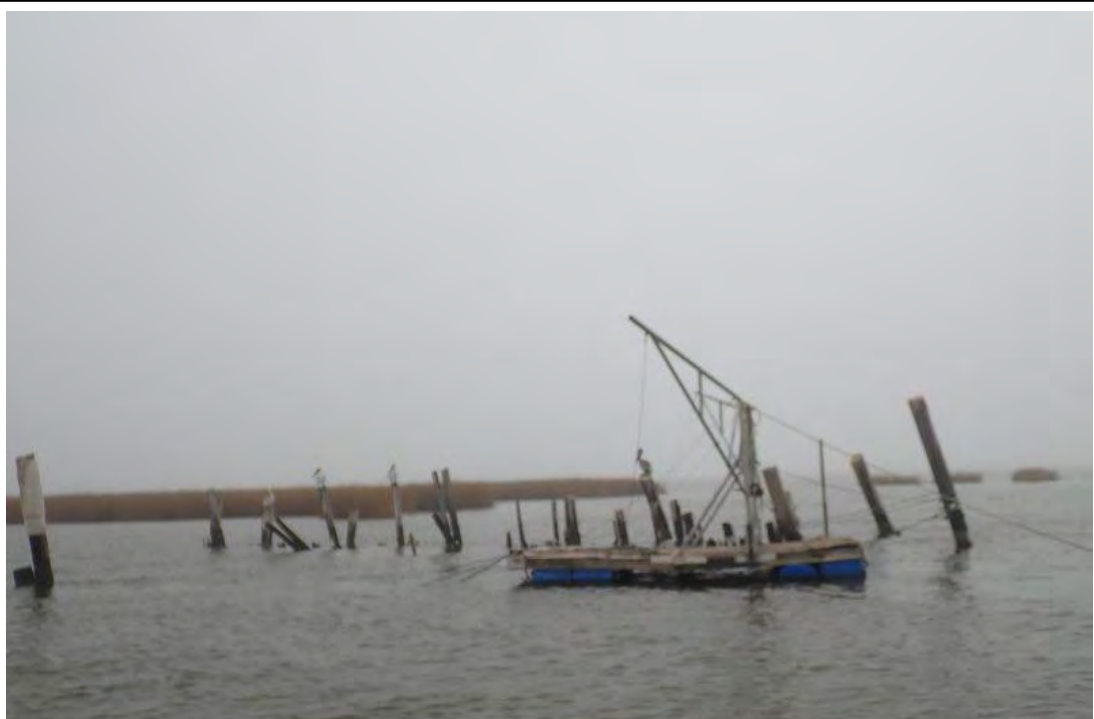
Photograph 106. Site 16: Shrimp Net Platform and Pilings (29°32'12.28"N, 89°54'9.78"W)
