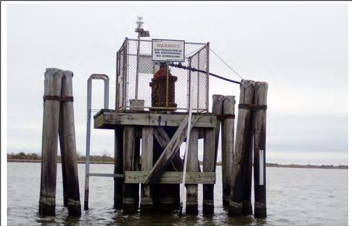
Photograph 137. Site 33: Pipeline Valve Platform (29°36'11.77"N, 90°4'28.50"W)
