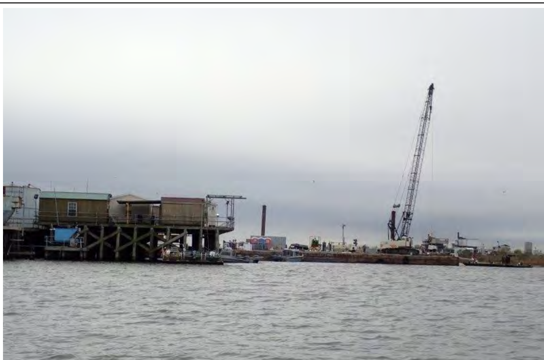
Photograph 134. Site 32: Oil Field Facility Structures
