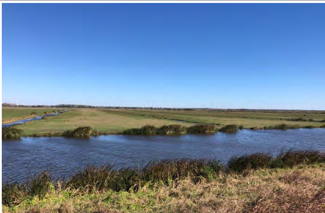
Photograph 46. Overview of Parish Levee Area Facing East
