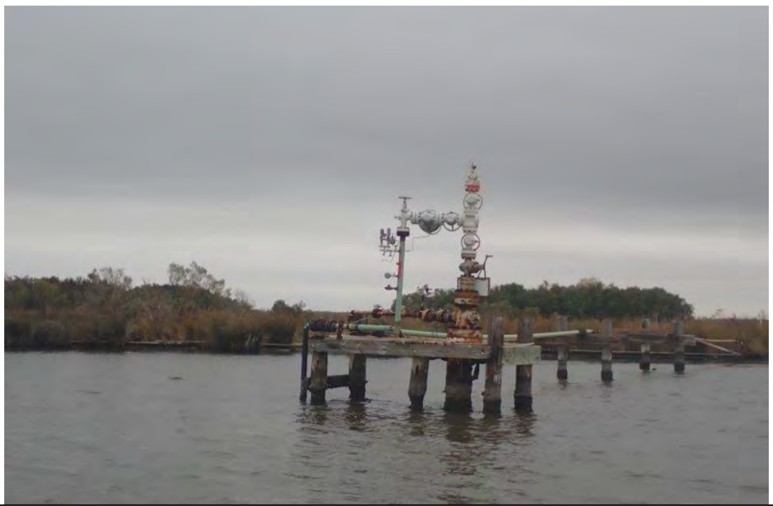
Photograph 147. Site 42: Well Platform (29°35'49.93"N, 90°1'43.70"W)
