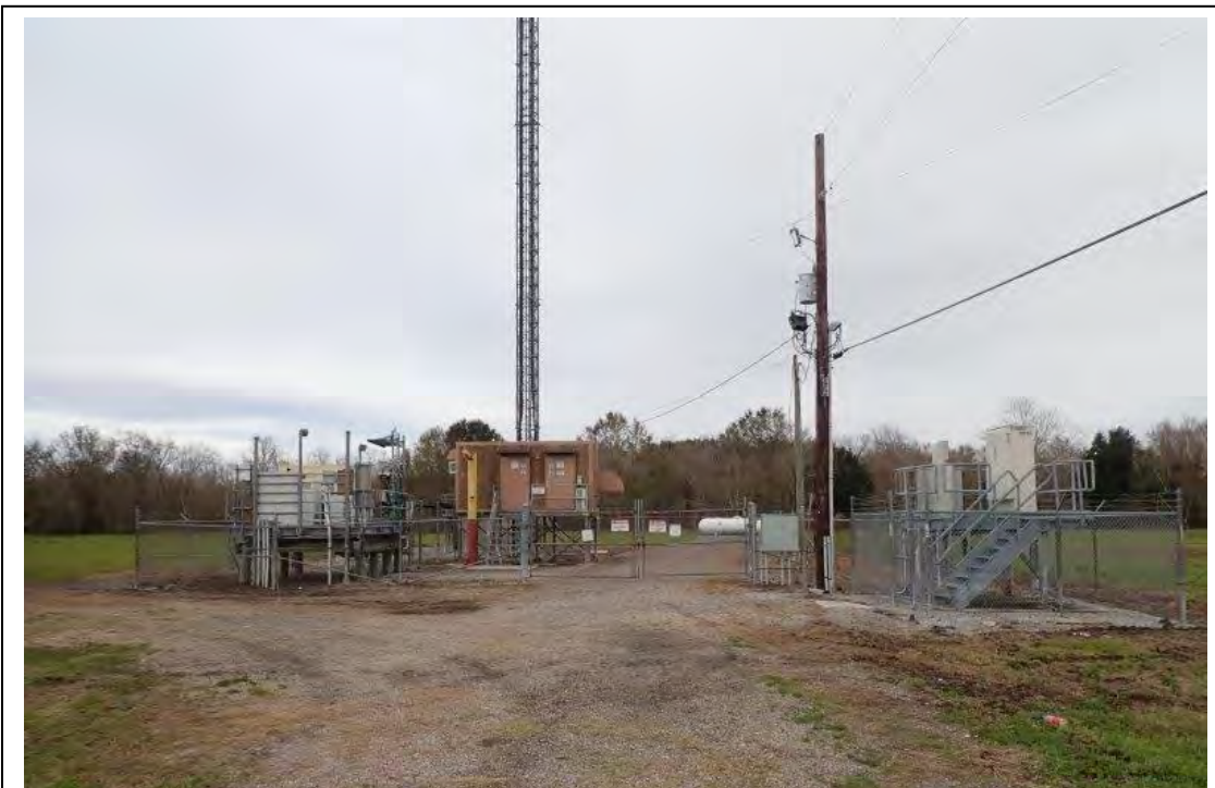
Photograph 80. Cell Tower Site (29°39'5.16"N, 89°58'32.10"W)
