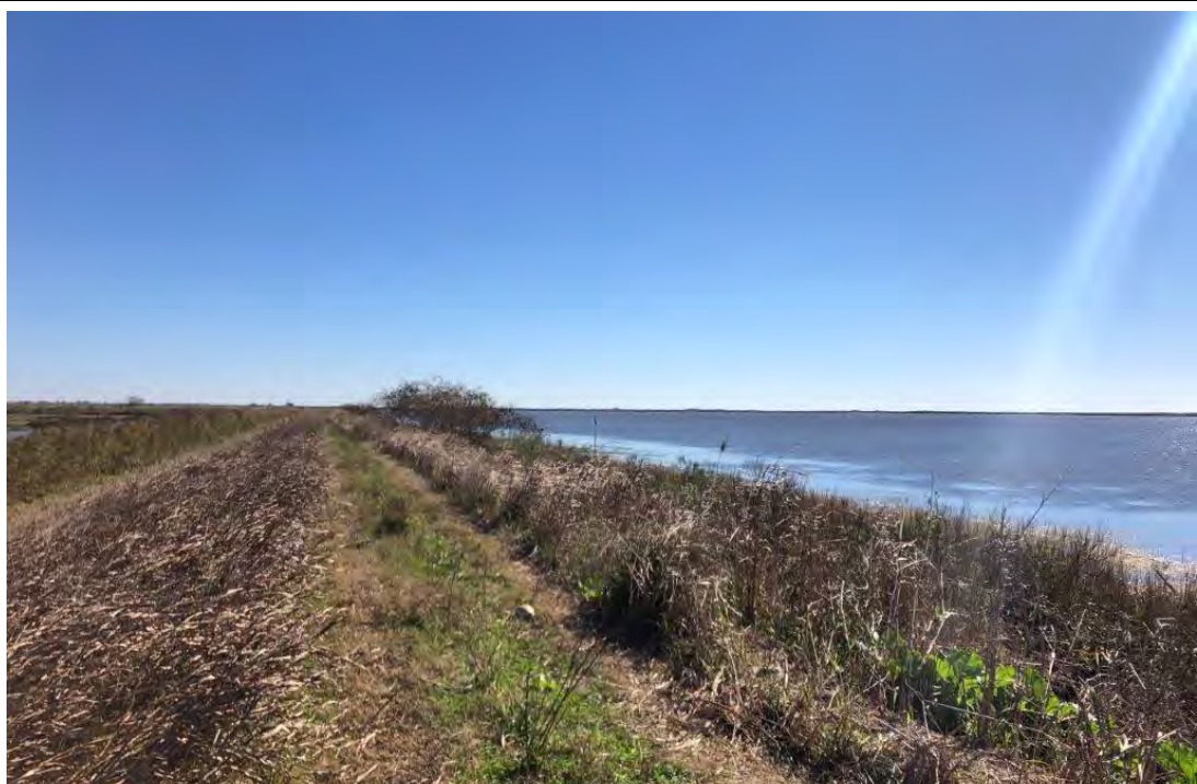
Photograph 48. Overview of Parish Levee Area Facing West
