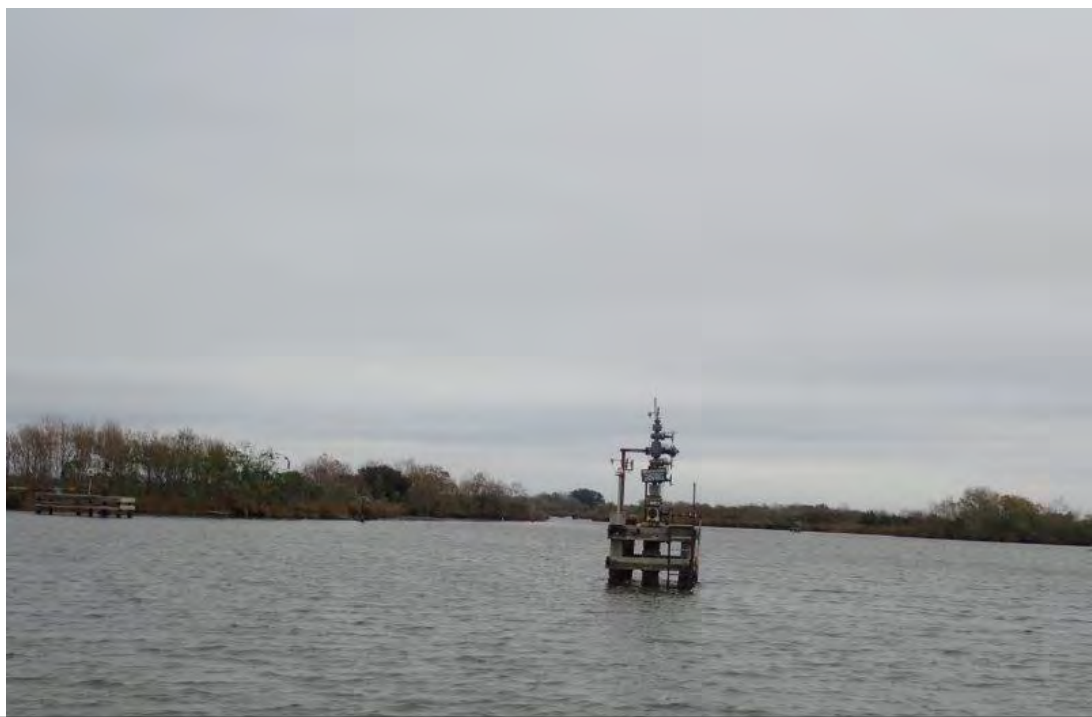
Photograph 133. Site 32: Oil Field Facility Structures
