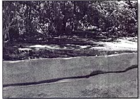
X-Tex used for Silt Fence
