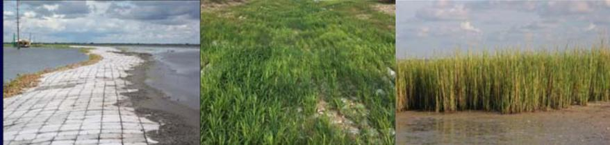
The Demonstration would be a comparison of a shoreline with ACBs, vegetated ShoreFlex II, and an existing marsh control section with no protection.
