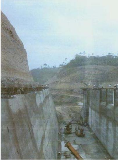
The very workable "wet shotcrete" mix was placed through heavy rebar and mesh directly onto a twenty-five meter high dirt excavation requiring extensive temporary support. By using shotcrete, the initial support and final one meter thick structural walls were done simultaneously. ST-ALKALI FREE ACCELERATOR was used for water control and temporary ground support.
