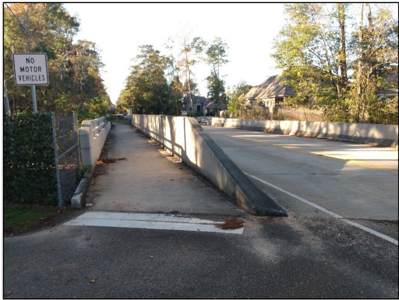
Figure D:10-53 New Bridge at W 15 Avenue Crossing Mile Branch
