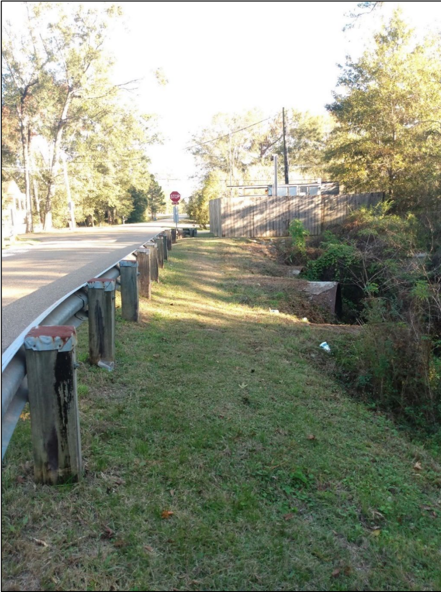
Figure D:10-51 Vehicular Bridge at W 19 Avenue Crossing Mile Branch
