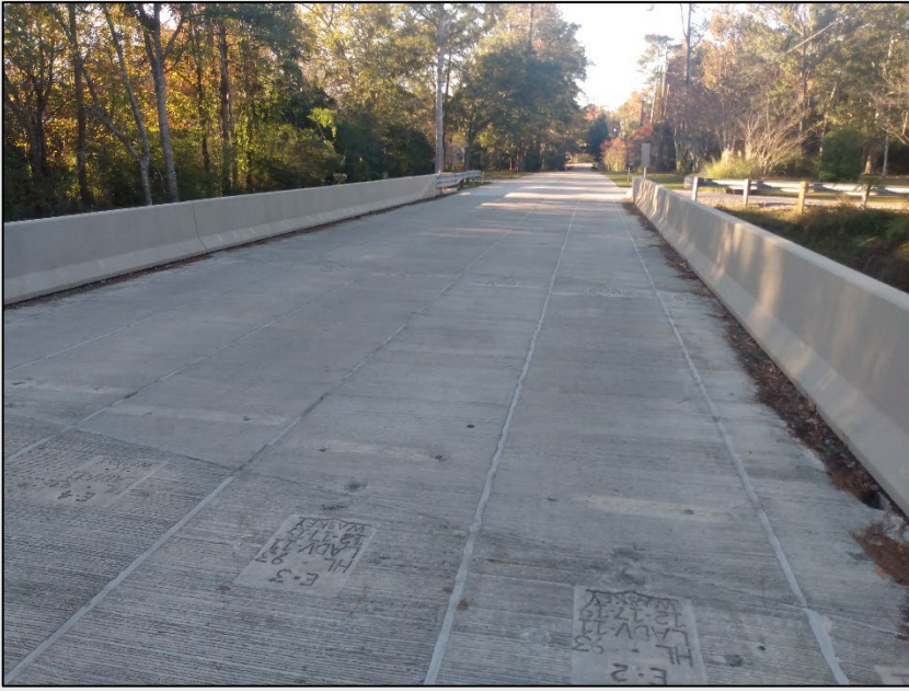
Figure D:10-54 New (Waskey) Bridge at W 11 Avenue Crossing Mile Branch
