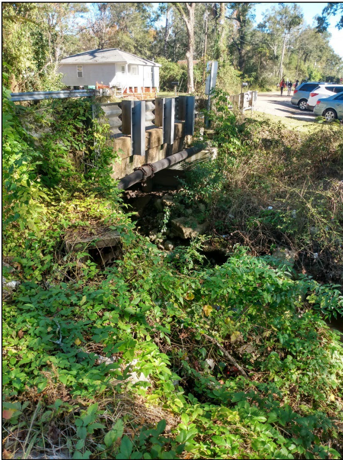
Figure D:10-45 Vehicular Bridge at W 29th Avenue Crossing Mile Branch
