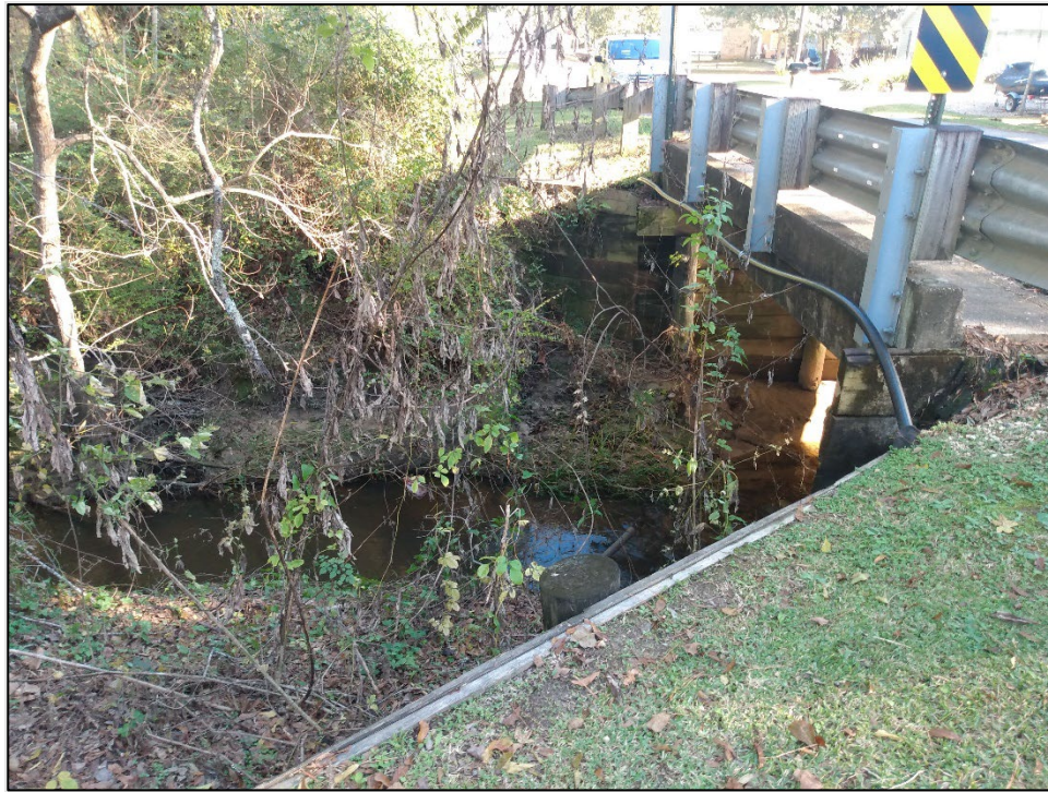
Figure D:10-49 Vehicular Bridge at W 23rd Avenue Crossing Mile Branch
