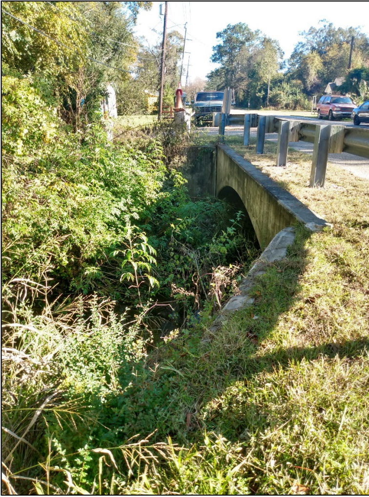
Figure D:10-46 Vehicular Bridge at W 28th Avenue Crossing Mile Branch
