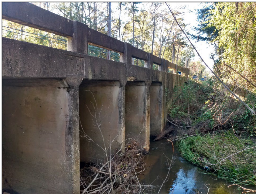
Figure D:10-50 Vehicular Bridge at W 21st Avenue Crossing Mile Branch
