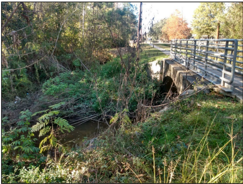
Figure D:10-47 Pedestrian Bridge at W 27th Avenue crossing Mile Branch
