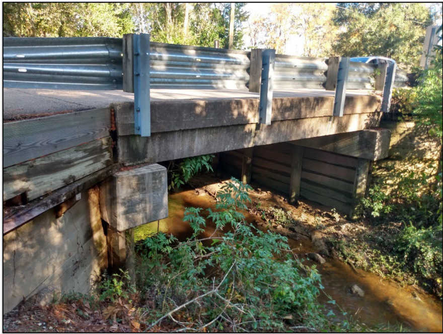
Figure D:10-48 Vehicular Bridge at W 25th Avenue crossing Mile Branch
