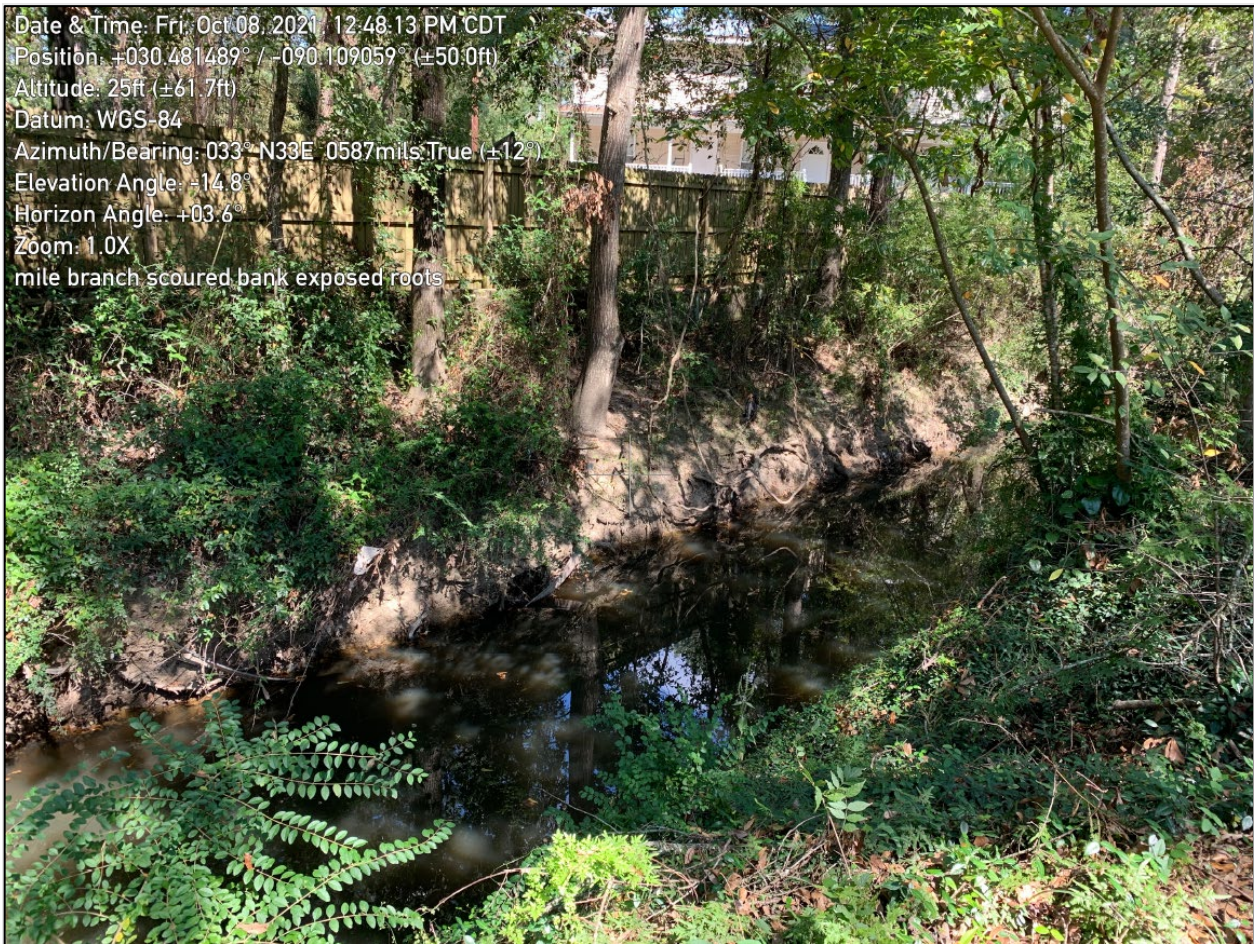
Figure D:10-42 Mile Branch (2021)
