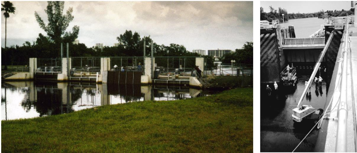
**Figure 14.** Water control structure retrofitted with pressure sensitive technology (left). Retrofitting of St. Lucie Lock with acoustic sensors (right) to protect manatees from being crushed as the gates close. (Photographs by FWS and B. Brooks)
