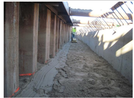
5. Materials are backfilled into the ground
