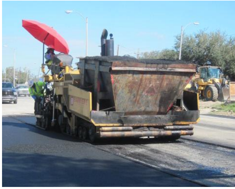
6. Roadway is restored
