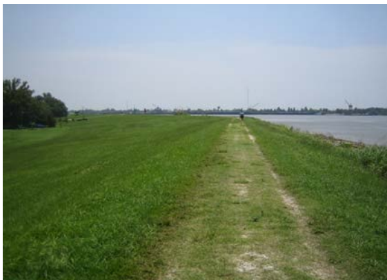
Photograph 2-2. Holy Cross levee with recreational trail
