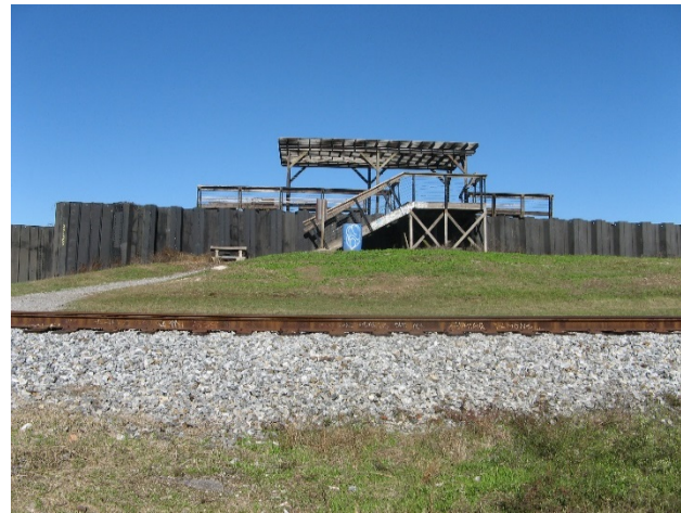
Photograph 2-4. Permanent viewing platform in the Lower Ninth Ward.
