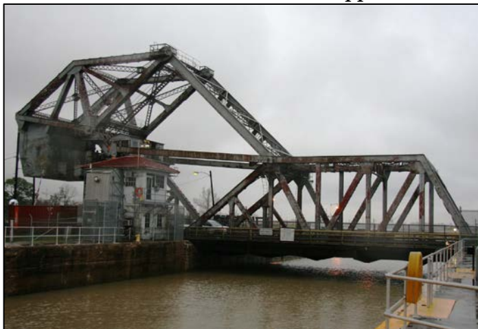
FIGURE A2-8: IHNC Lock Lower Approach Area
