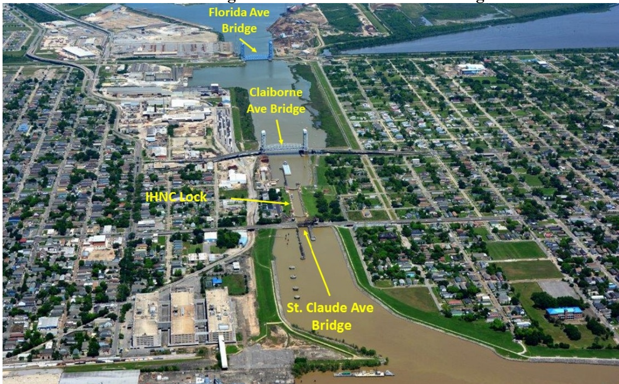
FIGURE 1-1: Inner Harbor Navigation Canal Lock and Related Bridges
