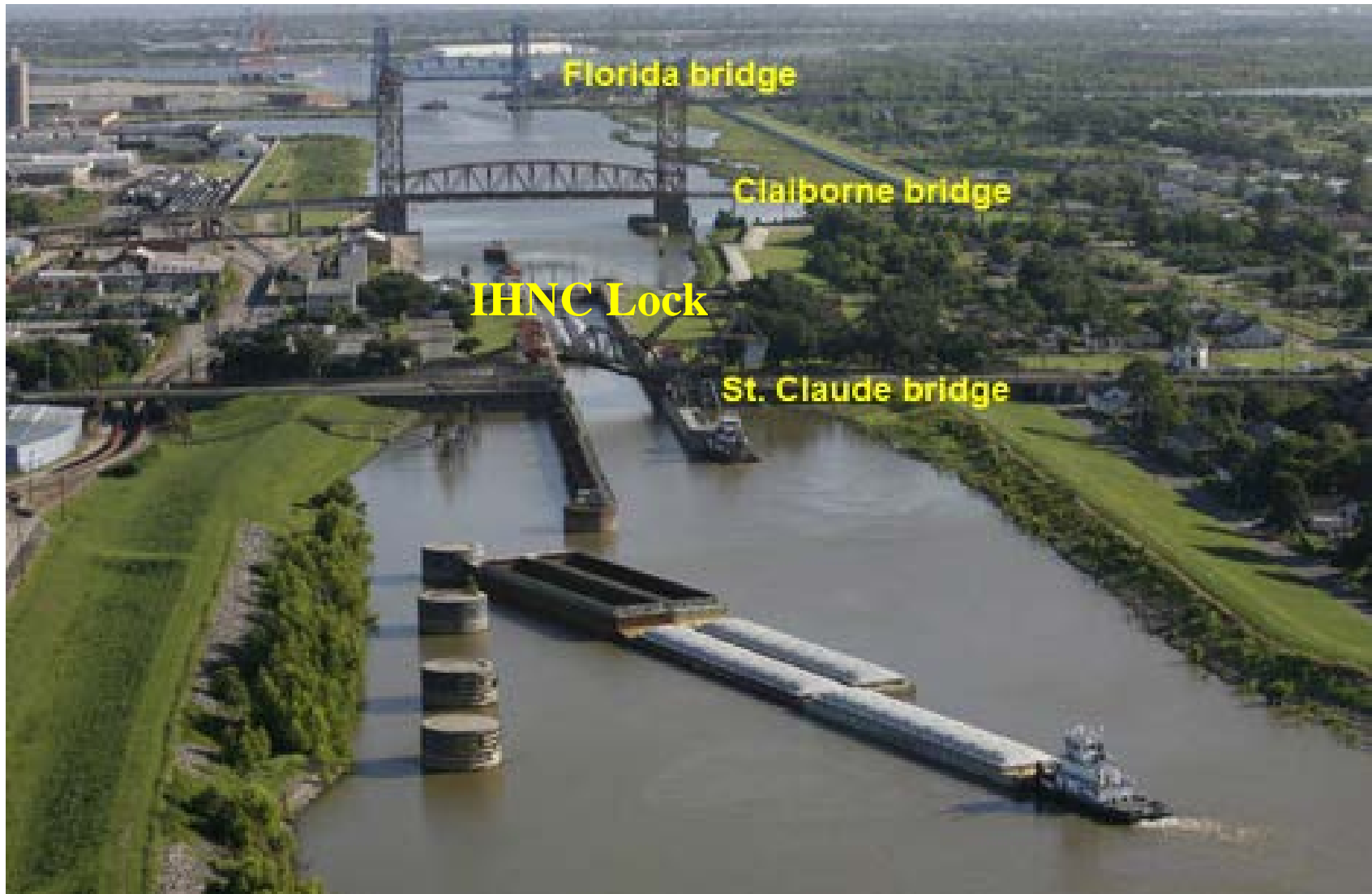
Figure 4: Looking North at IHNC Lock Complex
