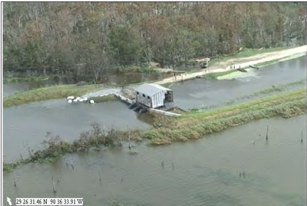
Figure 2-4. Breach at Lashbrook Pump Station on Ward 7 Levee along Boudreaux Canal Scour has undermined timber fronting protection, allowing water to seep under pump station.
