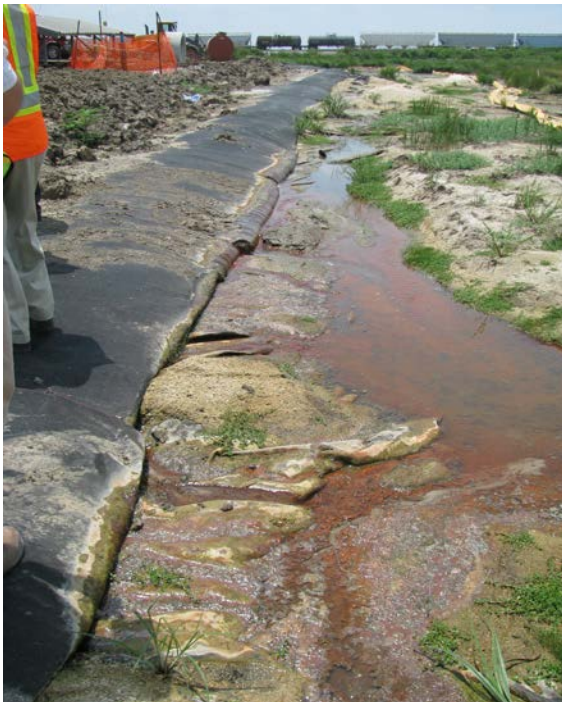
Figure 1. Water removal from levee system
