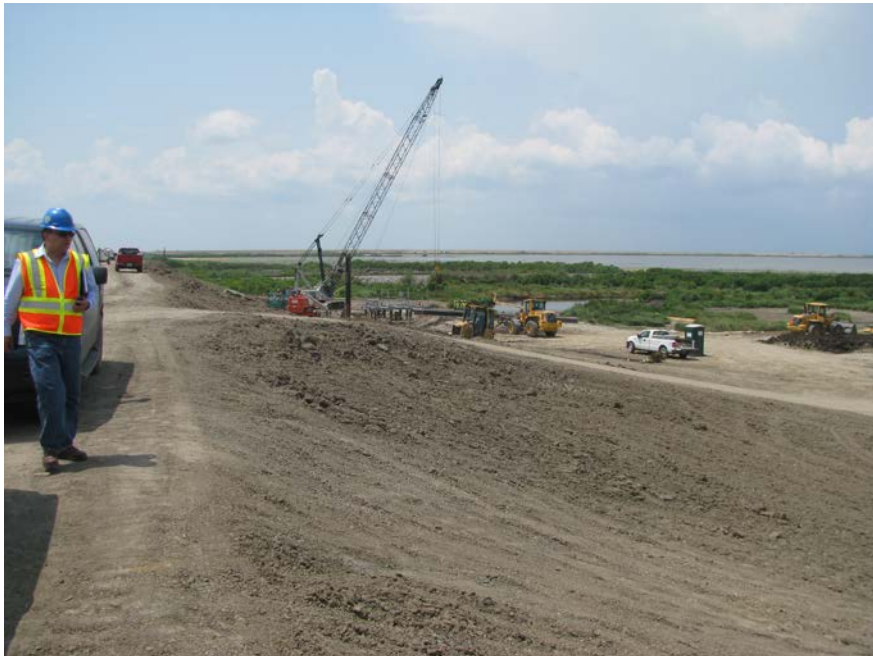
Figure 3. Levee with Pump Station No. 2 construction in the distance
