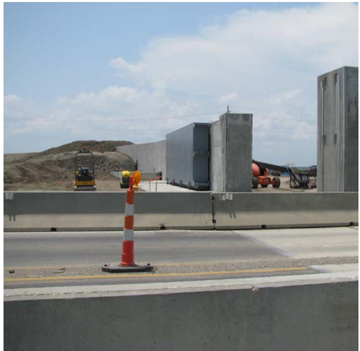
Figure 2. View of Highway closure gate at US-90
