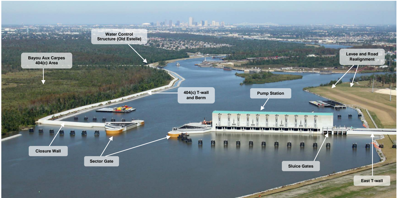
Image of the GIWW-West Closure Complex
