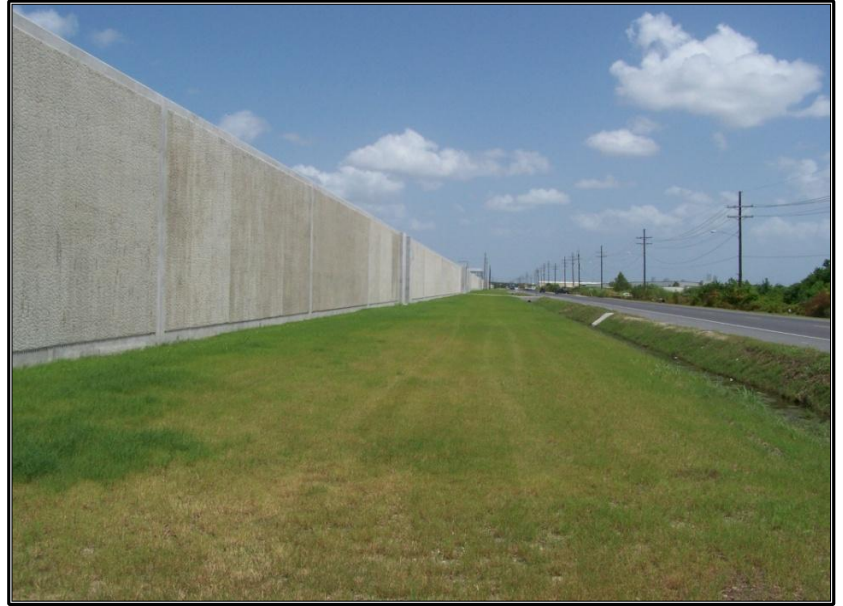
View of the Harvey Canal Floodwall along Peters Road.
