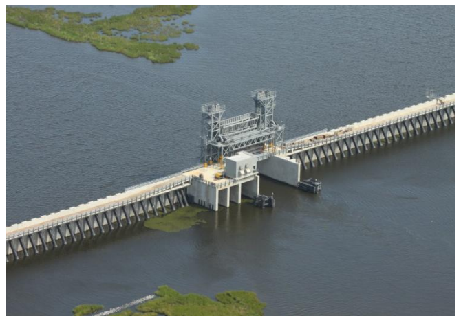
Vertical Lift Gate at Bayou Bienvenue
