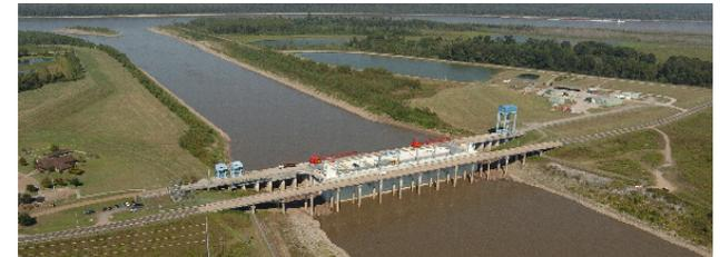
The Sidney A. Murray Jr. Hydroelectric Station is the largest prefabricated power plant in the world and Louisiana's first hydroelectric power plant.
