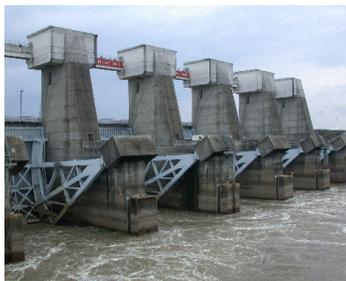
The Auxiliary Structure works together with the Low Sill Structure to maintain a 70-30 flow distribution between the Mississippi and Atchafalaya rivers, respectively.
