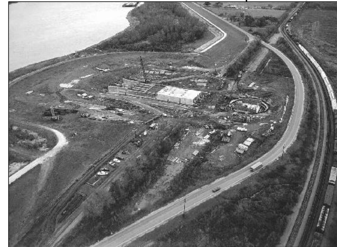
The state highway and railroad, now detoured to the right, will pass over Davis Pond when completed.
