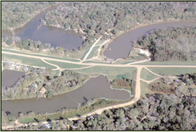
Bayou Courtableau Control Structure
