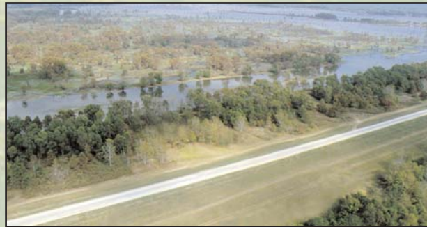
West Atchafalaya Basin Protection Levee looking into the Atchafalaya Basin
