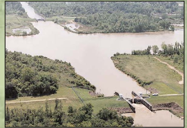
East and West Calumet Floodgates
