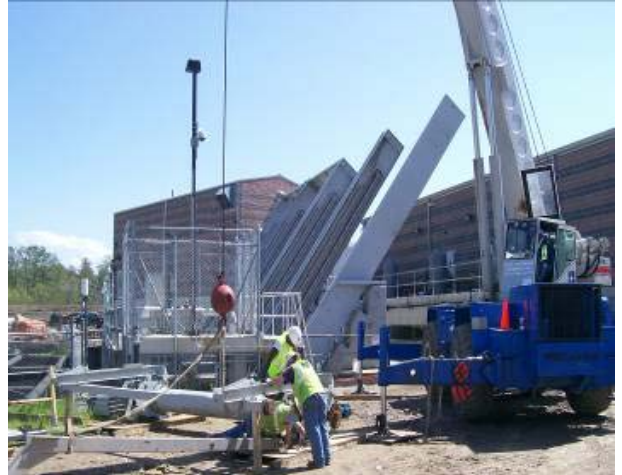
Climber Screens at Westminster Pump Station
