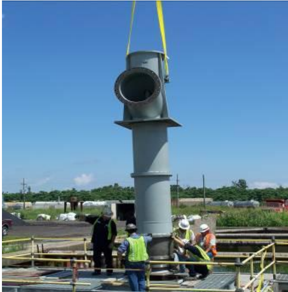
Installation of vertical pump at Elaine Street Pump in Orleans Parish
