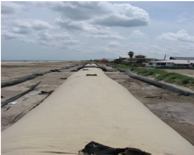
Geotextile Center Tube with Anchor Tubes
