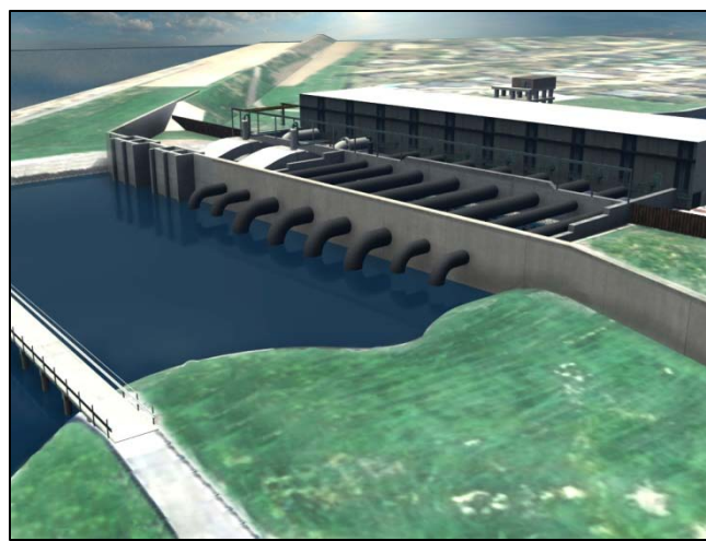
Pump station with Fronting Protection in place.
