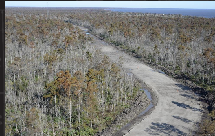
SP2 Sand base placed along levee alignment
