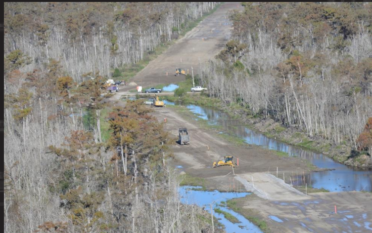
SP2 Sand base placed along levee alignment
