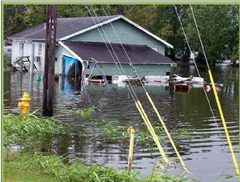
Hurricane Ike flooding in Delcambre, Louisiana 2008.
