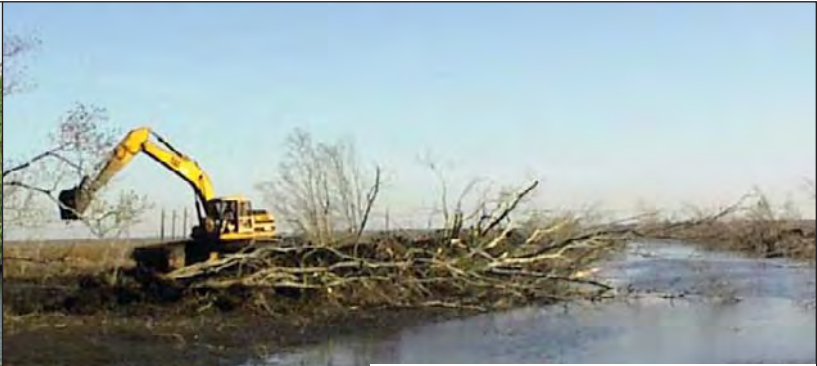
CANAL BACKFILLING IN PROGRESS
