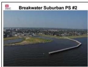
This is the Breakwater Suburban pump station. Concrete piles knock the waves down so it helps the pump station. We're planning to maybe have a break fall at pump station one and four. Two and three already have it.
