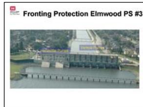
There is fronting protection at each pumping station. There are vertical pumps which are cylinder discharges and there are horizontal pumps. There are 13 pumps [inaudible] 1,000 cubic feet per second.
