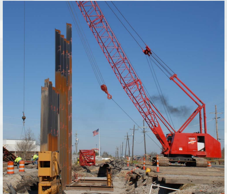
Construction of concrete T-walls will require pile driving.
