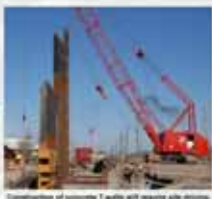
Construction of concrete T walls will require pile driving.
