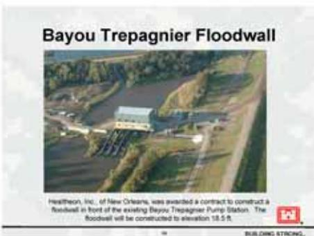
At Bayou Trepagnier, we are going to be doing an existing drainage structure there as the law required because of the Cross Bayou Pump Station. We are removing the existing structure and replacing that with a T-wall and we will also be doing is replacing a floodwall called [Inaudible] in front of the Bayou Trepagnier Pump Station.
