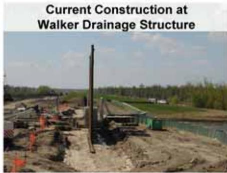
flowing underneath the structure from flood side to protected side. After they finish driving the sheet piles they will go ahead and drive new H-piles and then they will pour the stability slab and then they will pour the new T-walls.
