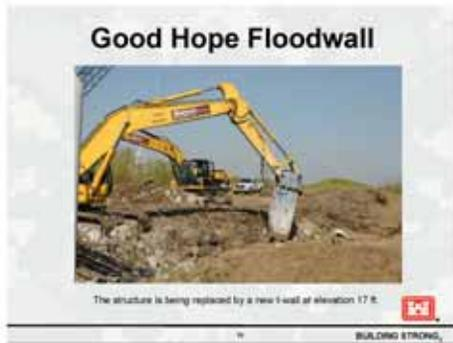
You can't see it here in this picture, but off to the flood side, there is temporary flood protection installed to the elevation of +6. I told you about that, it protects from high lake levels and high tide outside of hurricane season. What they are doing is demolishing the existing wall here before they begin driving piles and then reforming and pouring new concrete T-wall.
