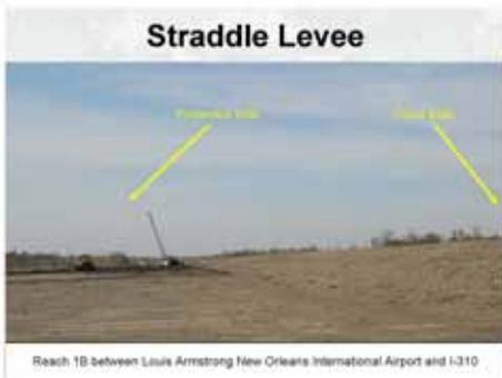
And this is just a picture of a nearly completed levee. This is near the railroad gate by the airport looking down towards 310. This is called Reach 1B and this is called a straddle levee section where they have just gone on top of the existing levee and added additional material to both the berms and the levee raising it up to our 100-year designed standards.
