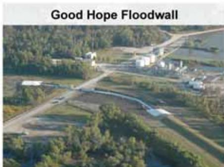
At the Good Hope Floodwall, we are going to be increasing the levees, it's actually going to be replacing this portion right here and then we are going to replace the existing floodwall with a stronger and higher T-wall. This picture is looking at the west side of the wall right here, they have already begun to demolish.
