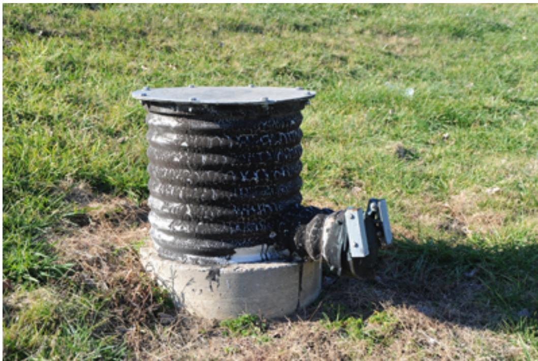
**Figure 3: Typical relief well with a diameter of 8 inches standing approximately 20 inches above ground. A concrete pad (not shown in this picture) would be present to direct flow from the well.**
