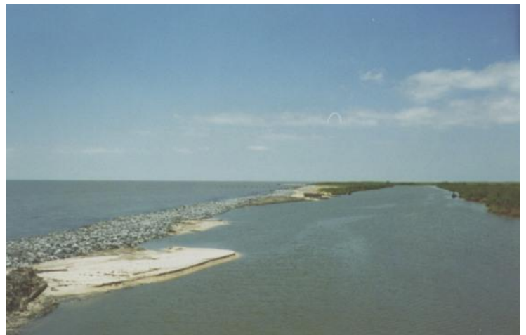
This section of Mobil Canal was backfilled and armored with rock to reestablish the separation between the canal and the gulf so that salt water would be prevented from damaging the intermediate marshes in the interior of the island.
