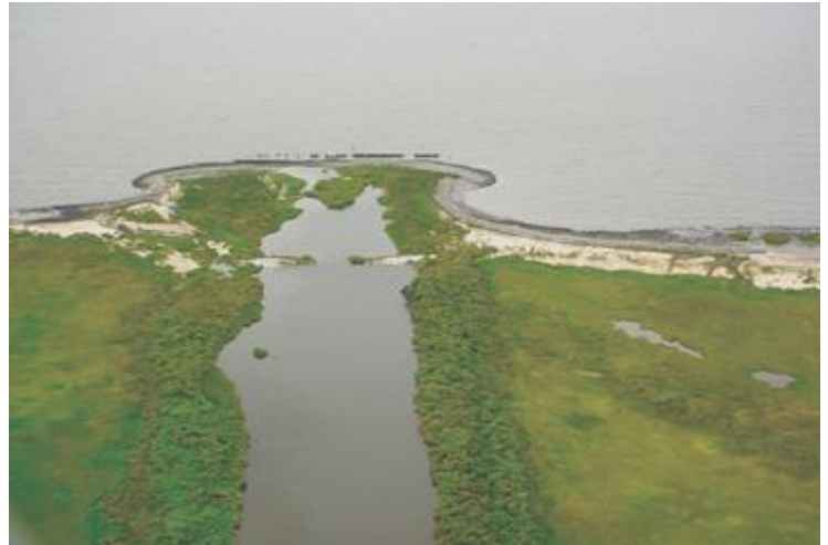
The beach where a pipeline canal meets the Gulf of Mexico has been stabilized with concrete mats thus preventing saltwater intrusion into the interior wetlands of Point au Fer Island.
