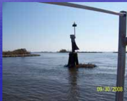
Southeast side of Structure No.6
