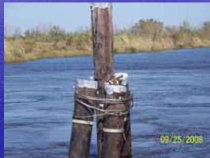
Typical Timber Dolphin – Structure No.1
