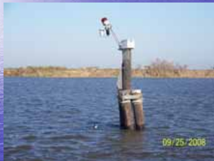
Timber Dolphin – Structure No.14A
