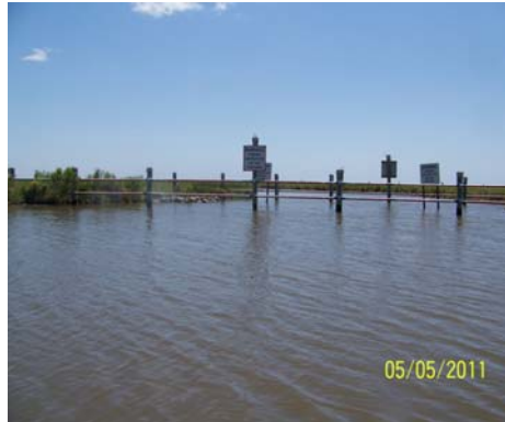
Weir #5 looking east
