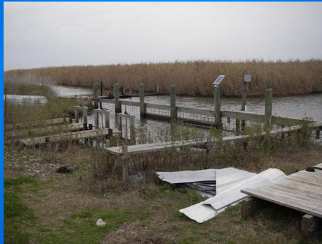
View of Structure No.1
