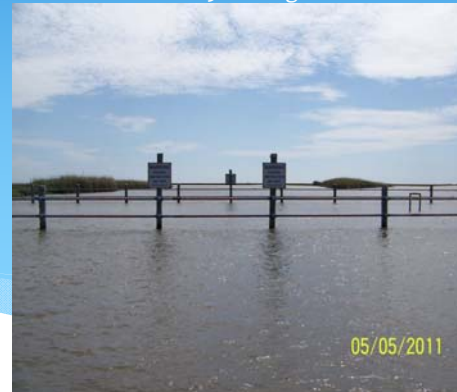
Weir #9 looking east
