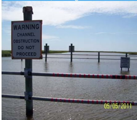
Weir #7 looking northwest
