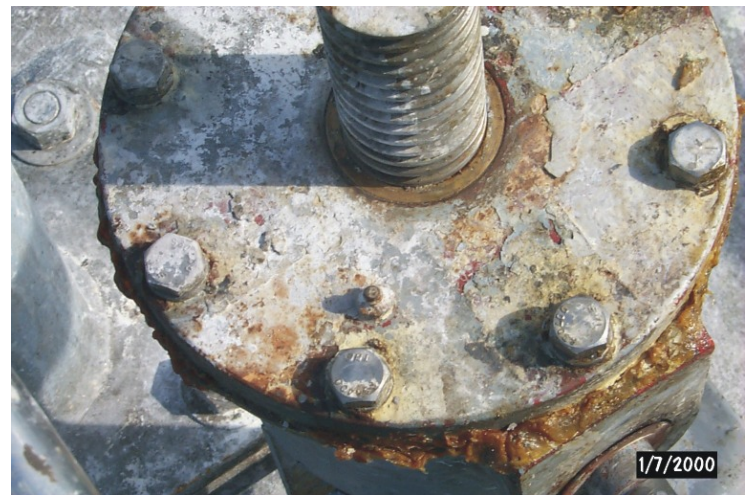
The salty environment of the project area leads to severe corrosion of unprotected pipes, fittings, and valves. This corrosion can eventually leave the water control structures inoperable.
