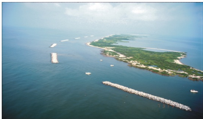
Rock breakwater construction for the prior demonstration phase of this project was completed on the east end of the island in June 1997. Taken immediately after construction was complete, this 1997 photograph shows no sand behind the breakwaters.
