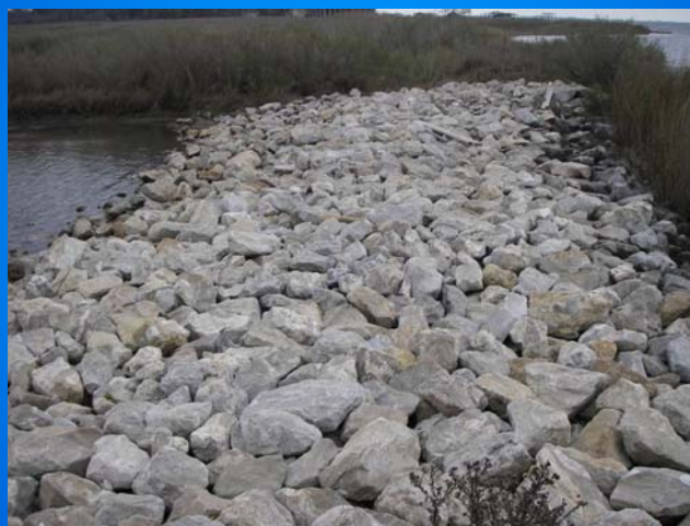
View of Structure No.8
