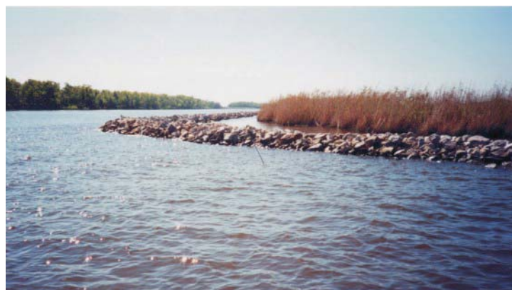
Limestone riprap was placed within a 4.3 mile reach along the north bank of the GIWW between the Vinton Drainage Canal and Perry Ridge.
