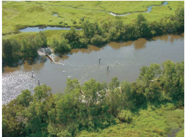
A low-level weir constructed across the British American Canal within the project area.
