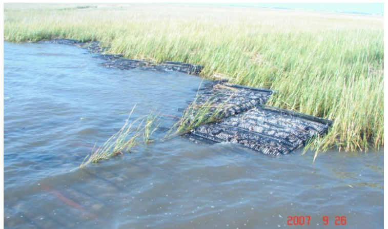
Installed Gabion Mats along the north shore of Lake Barre.
