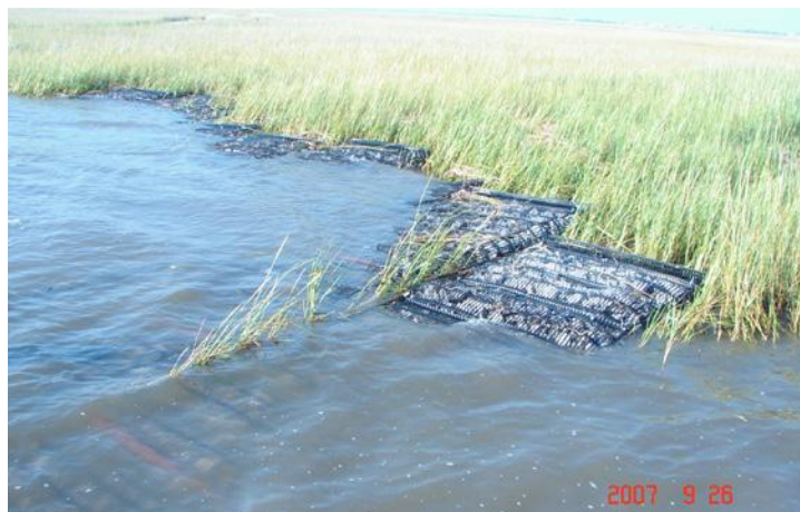
Installed Gabion Mats along the north shore of Lake Barre.
