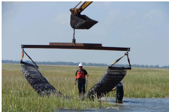
Installation of Gabion Mats (one of the three techniques being used on this project) along the north shore of Lake Barre.
