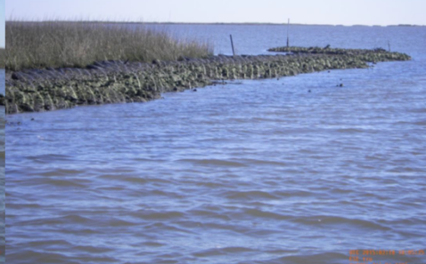
Gabion Mats Reach E
