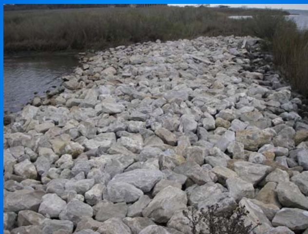
View of Structure No.8
