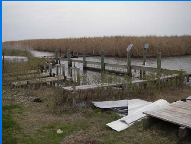
View of Structure No.1
