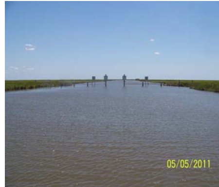
Weir #6 looking east
