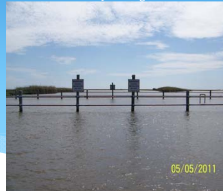
Weir #9 looking east
