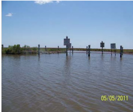
Weir #5 looking east
