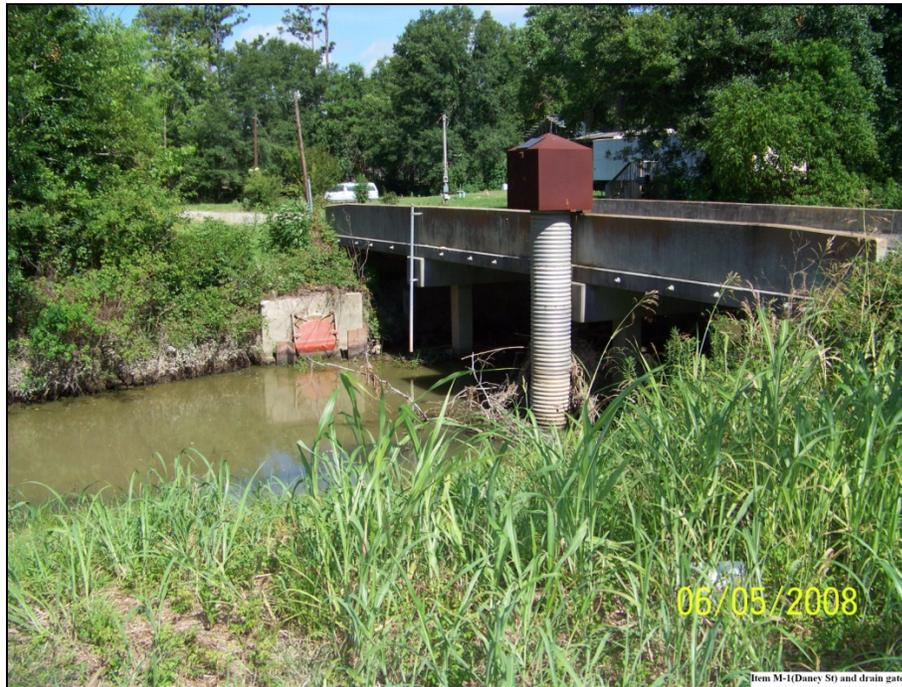
Figure 34. Item M-1, USGS Stream Gaging Station at Daney Street Bridge
