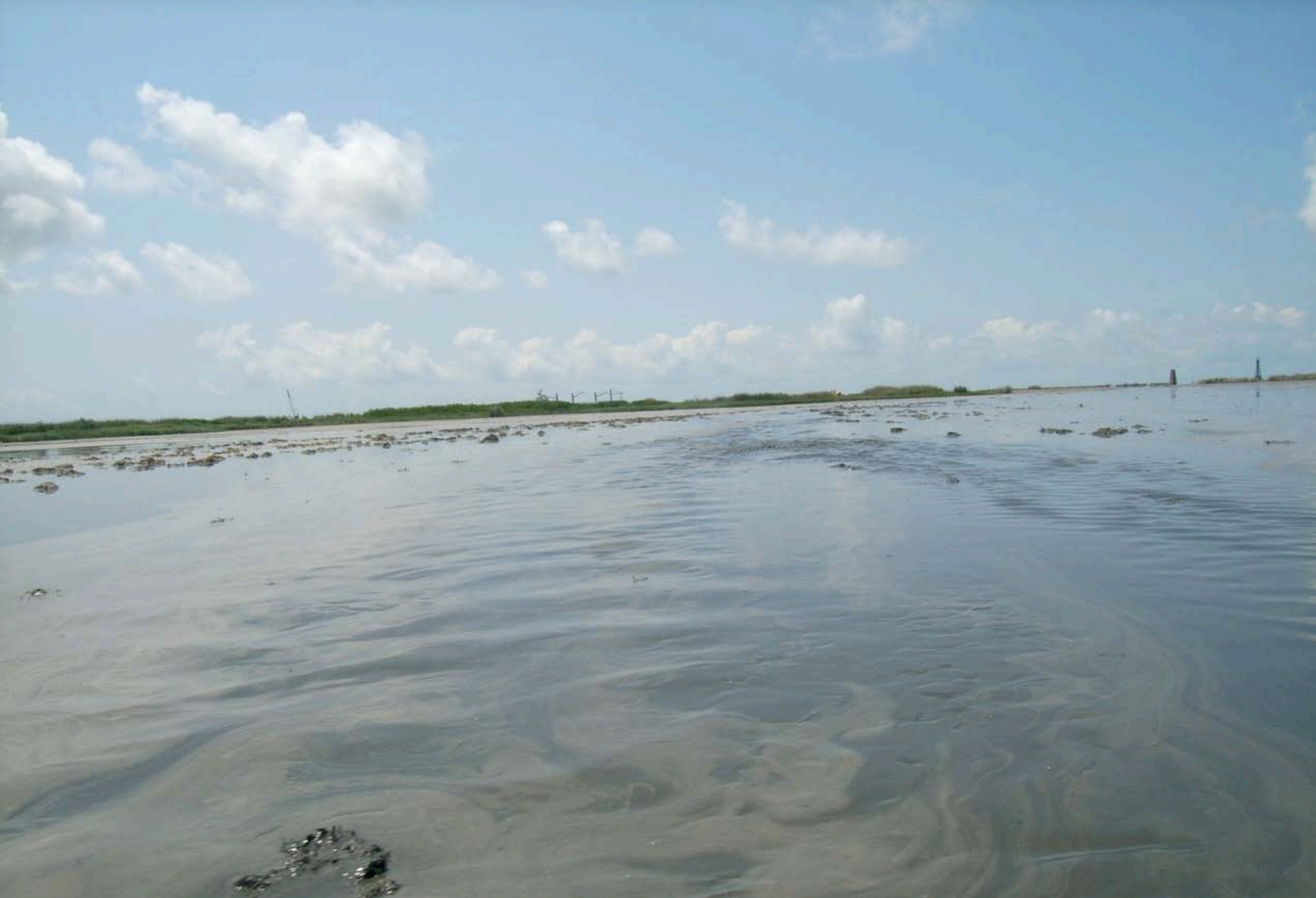
Picture 1. Upper boundary of Placement Area #1, looking towards the right-descending bank of Southwest Pass. The dredge CALIFORNIA was actively pumping into this beneficial use placement area, & flowing dredged material slurry generated the surface ripples visible in this photo.
