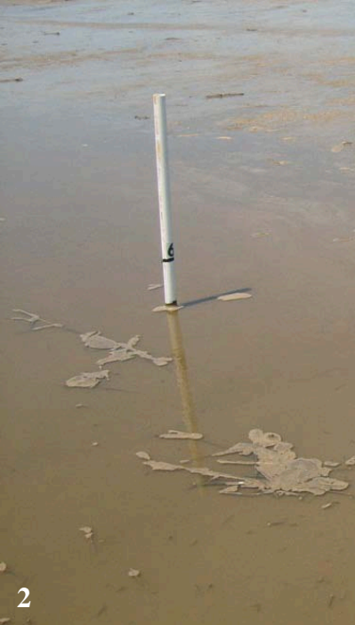
Pictures 2-3. Elevation marker denoting target slurry elevation of 5.5' (left). The CALAFORNIA was working near river mile 14 BHP (top). Other equipment was nearly obstructed by marsh grass within the placement area (below).
