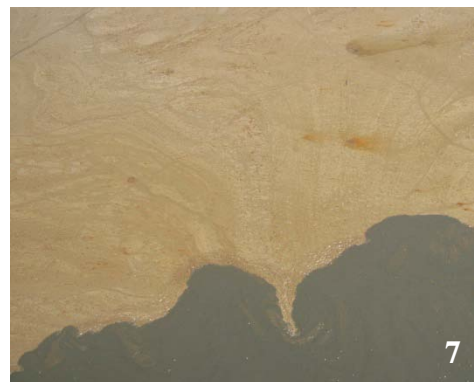
Pictures 5-8. Dredged material discharged into Placement Area #1 was predominantly fine-grained sediments mixed with organic material. Trail made by the leading airboat exposed its pudding-like consistency (above). Organic foam was scattered throughout the site (below).
