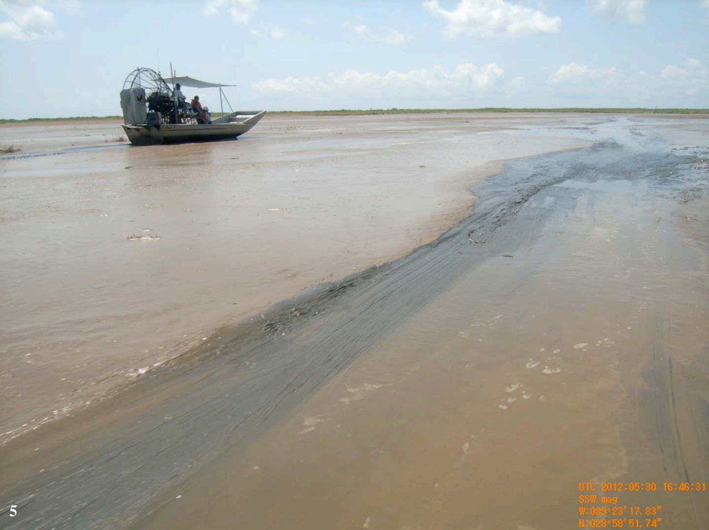
Pictures 5-8. Dredged material discharged into Placement Area #1 was predominantly fine-grained sediments mixed with organic material. Trail made by the leading airboat exposed its pudding-like consistency (above). Organic foam was scattered throughout the site (below).
