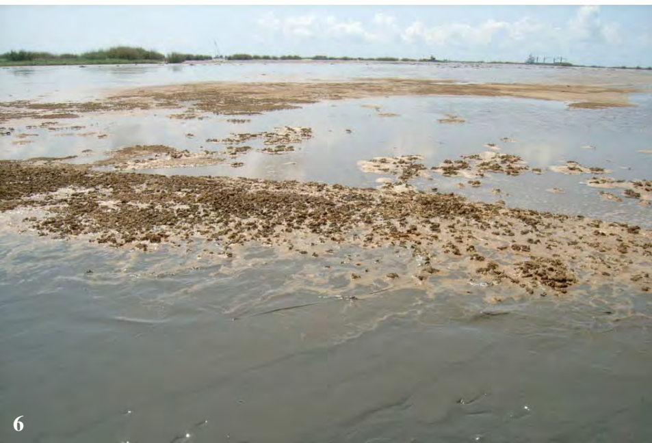
Pictures 5-8. Dredged material discharged into Placement Area #1 was predominantly fine-grained sediments mixed with organic material. Trail made by the leading airboat exposed its pudding-like consistency (above). Organic foam was scattered throughout the site (below).
