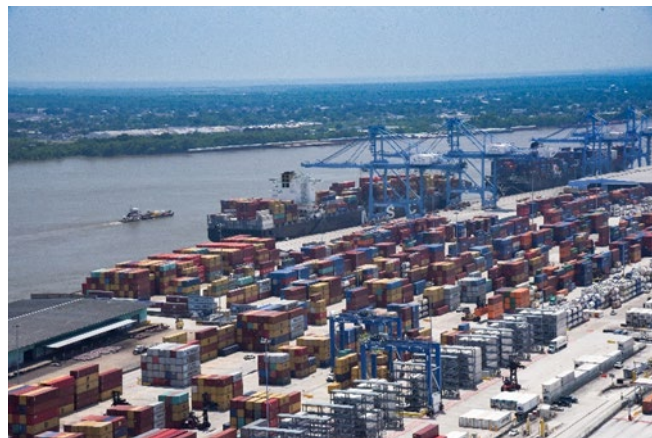
Figure 1: Port of New Orleans seen from near Napoleon Ave, New Orleans.
