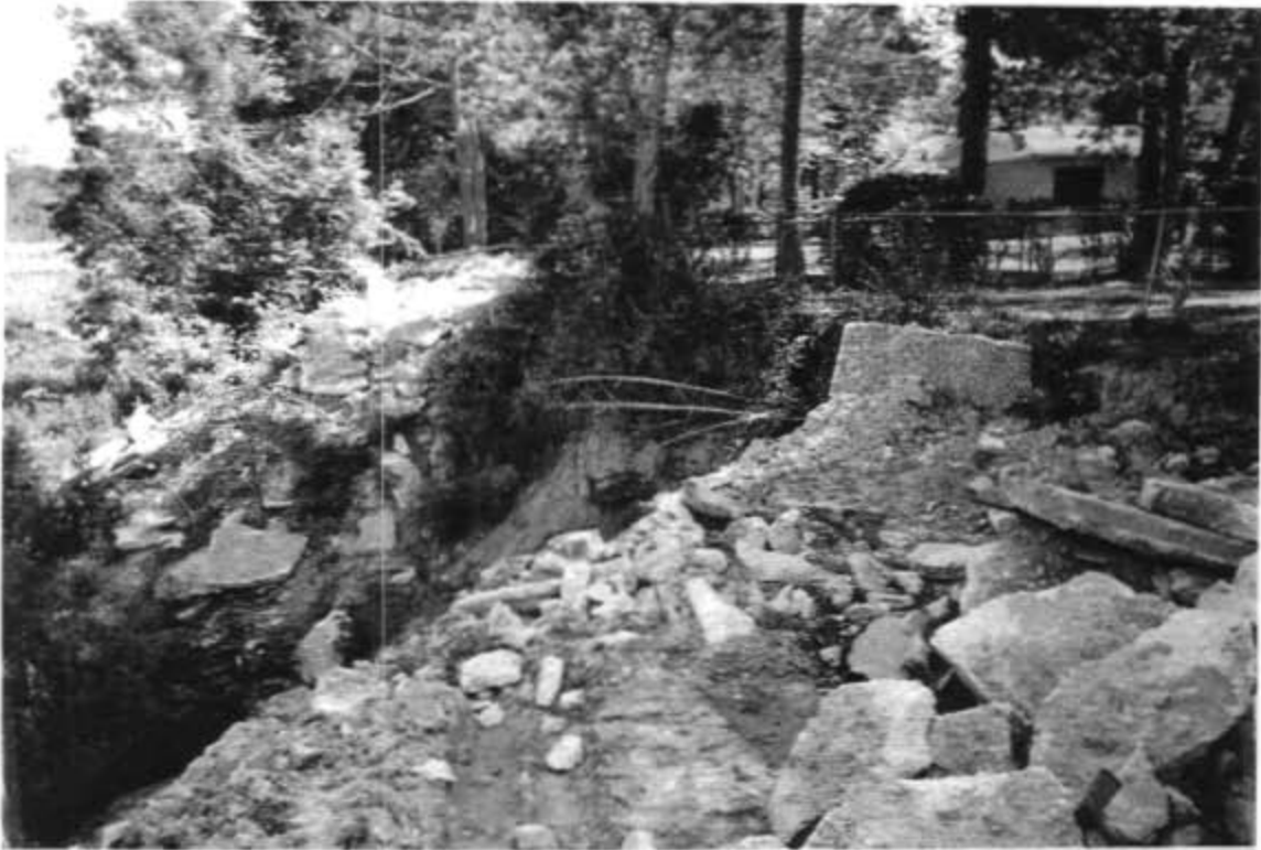
NORTH BRANCH WARD CREEK-BANK FAILURE AND ATTEMPTED RIP-RAP REPAIR
