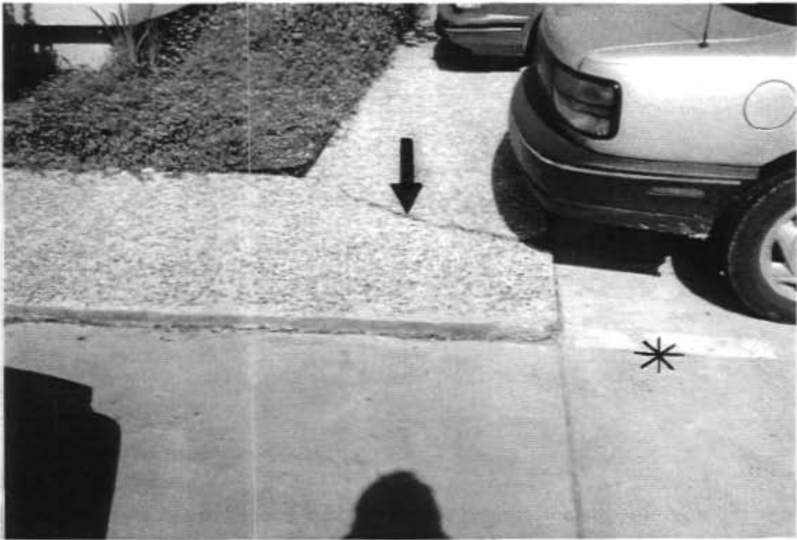
NORTH BRANCH WARD CREEK-EVIDENCE OF GROUND MOVEMENT CLOSE TO BUILDING (*REFERENCE POINT PREVIOUS PHOTO)
