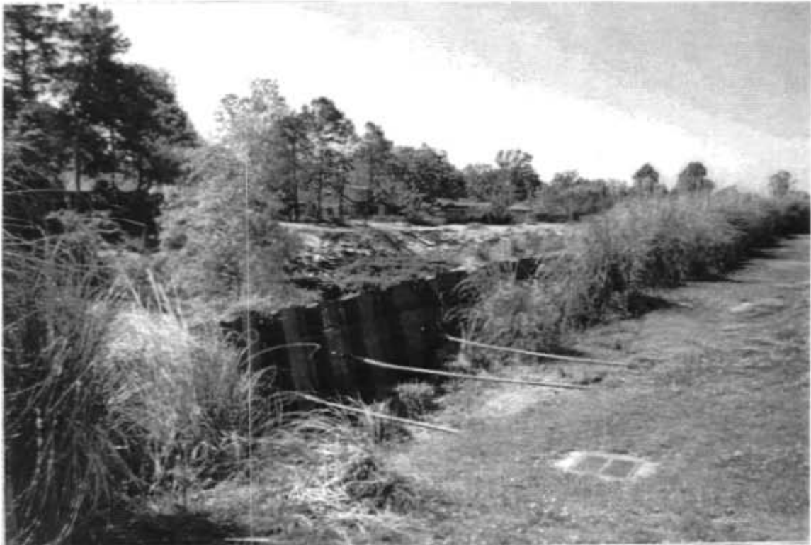
NORTH BRANCH WARD CREEK-SHEETPILE RETAINING WALL FAILURE
