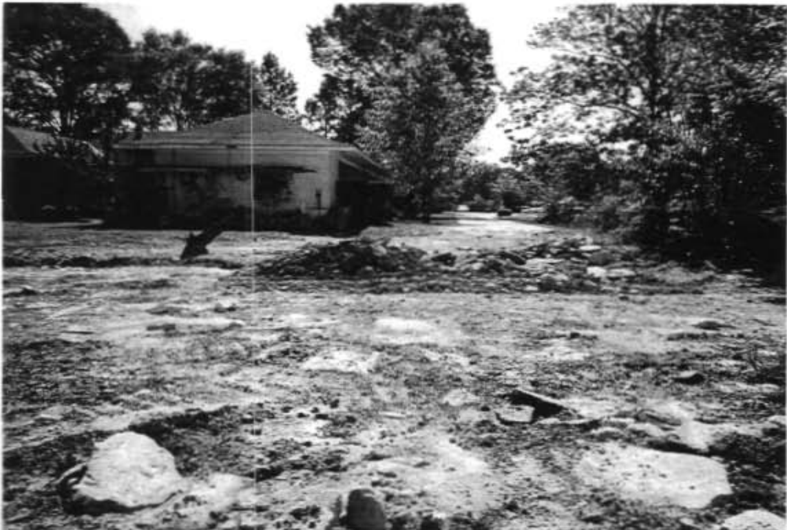
NORTH BRANCH WARD CREEK-BANK FAILURE AND ATTEMPTED RIP- RAP AND FILL REPAIR; NOTE NEW FAULT CLOSER TO STRUCTURE
