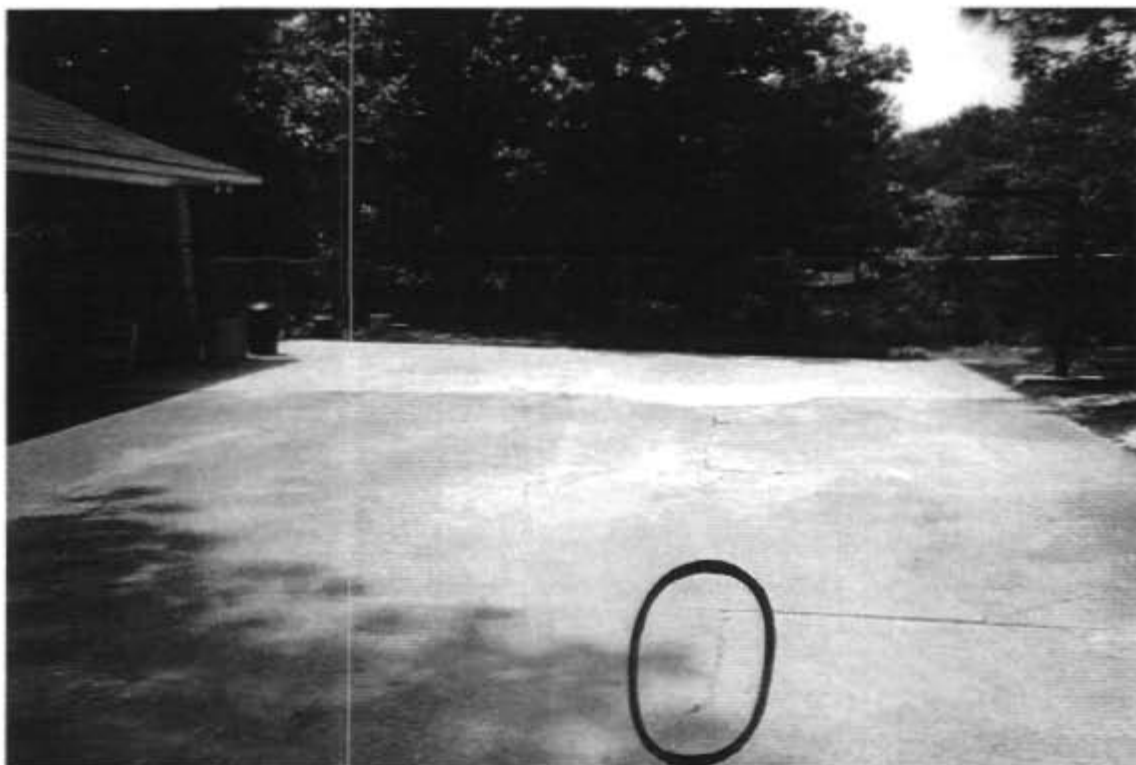
JONES CREEK-GRADE LEVEL, FENCE AND SLAB REPAIR (NORMAL TO CREEK VIEW); NOTE DAMAGE EXTENTION DISTANCE
