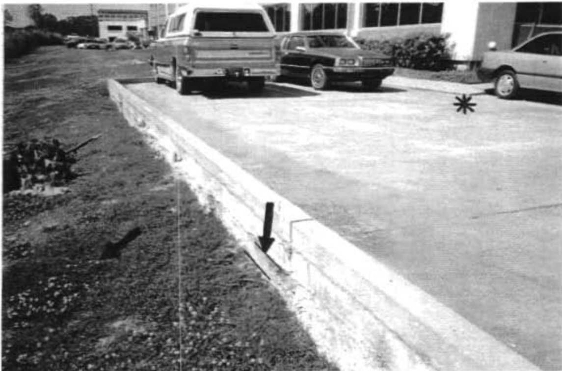
NORTH BRANCH WARD CREEK-BANK FAILURE: NOTE MOVEMENT TRANSLATION (*REFERENCE POINT NEXT PHOTO)
