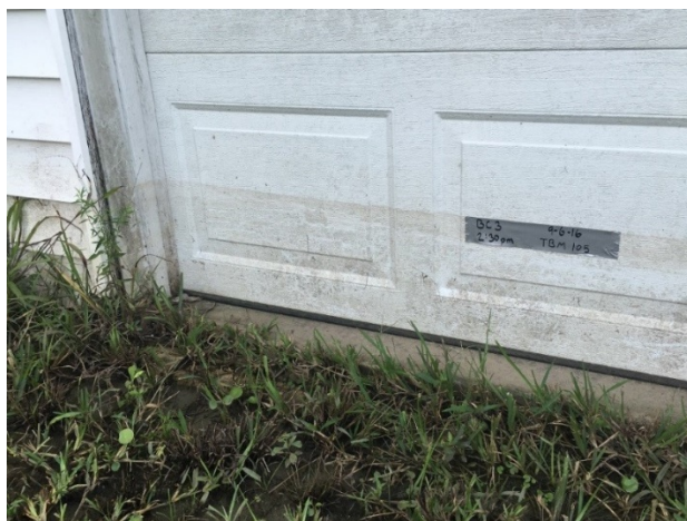
Figure 8: Example mudline on exterior of building.
