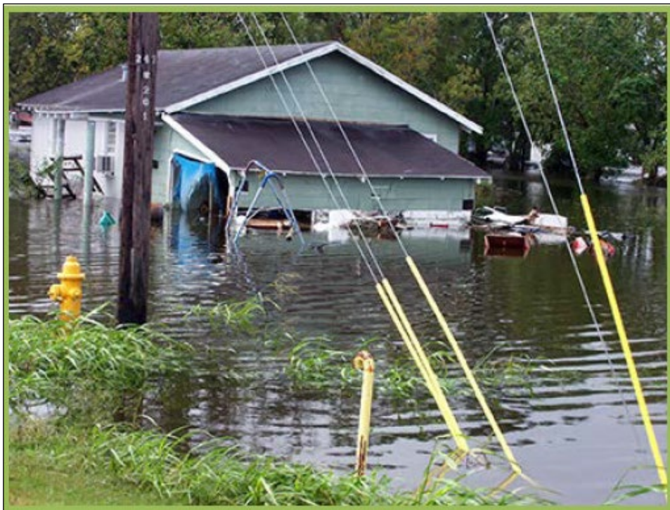
Hurricane Ike flooding in Delcambre, Louisiana.
