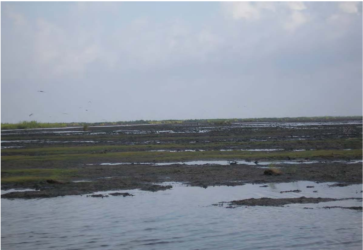
Figure 5. Proposed planting area damaged by Hurricanes Rita and Ike (September 2005 and 2008). Photo taken in July of 2009.
