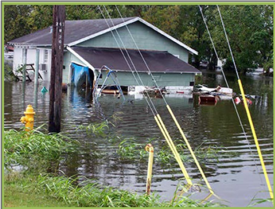
Hurricane Ike flooding in Delcambre, Louisiana 2008.
