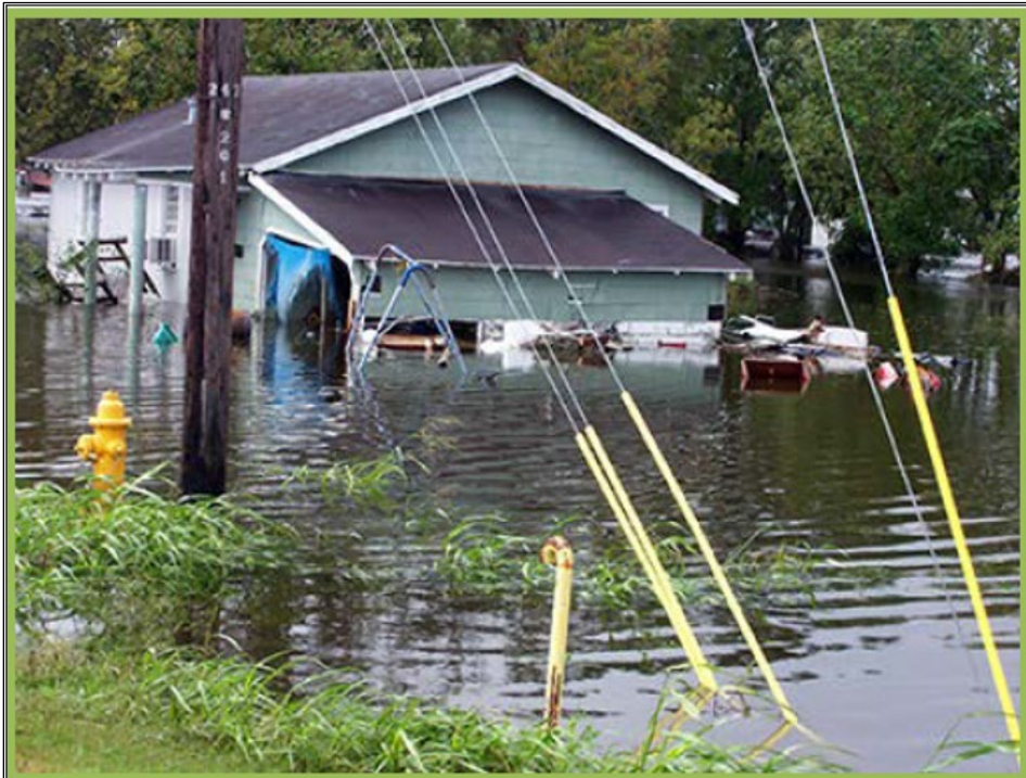
Hurricane Ike flooding in Delcambre, Louisiana 2008.
