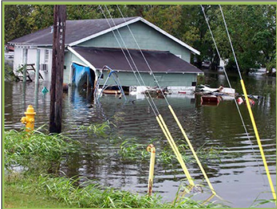
Hurricane Ike flooding in Delcambre, Louisiana 2008.
