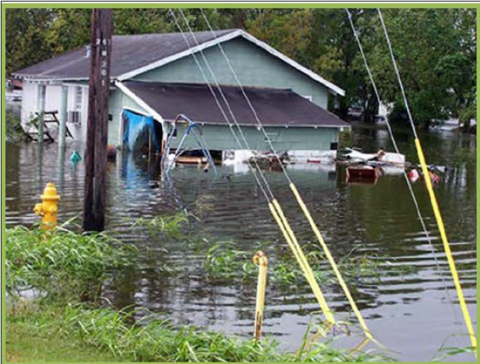
Hurricane Ike flooding in Delcambre, Louisiana 2008.
