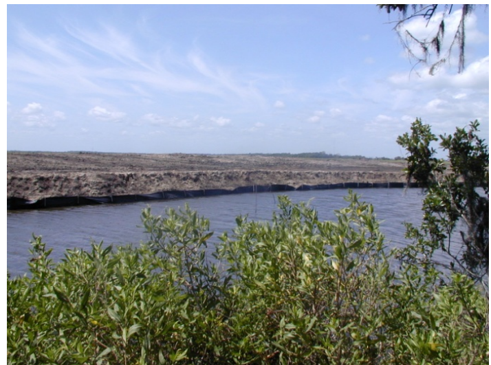
Levee Reach J-1 Construction
