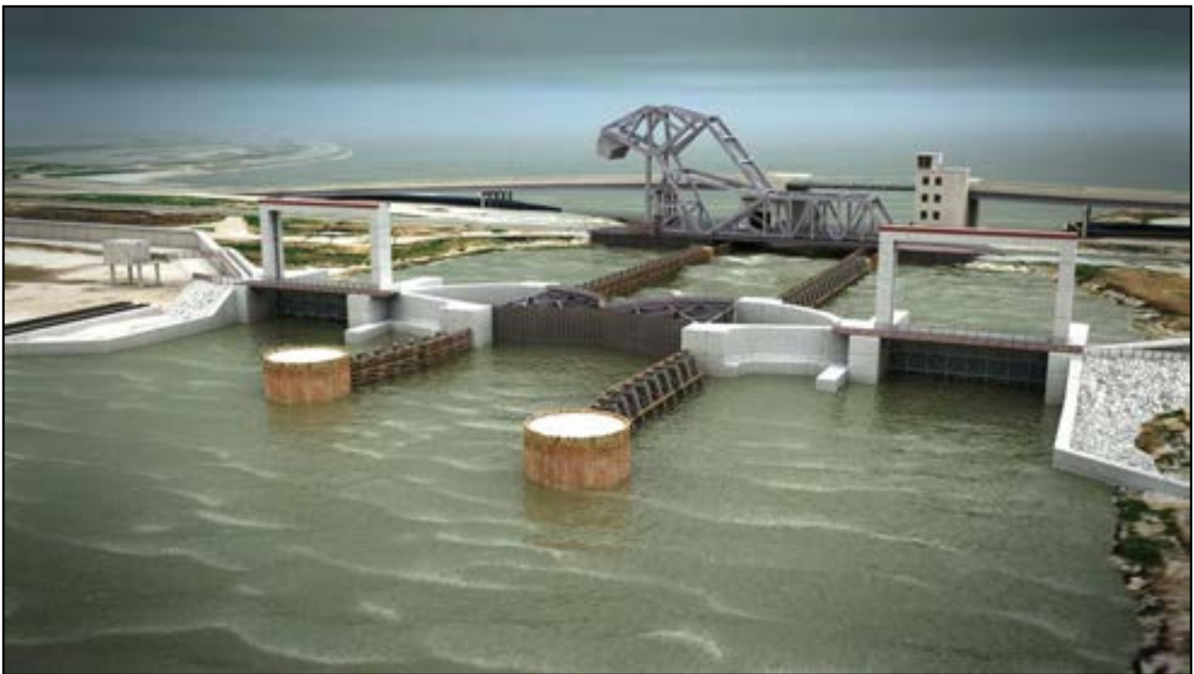
Figure 10. Simulated Image of Proposed Action Alignment in the Open and Closed Positions (During storm conditions when gates are closed, water level will be higher on the floodside of gates)
