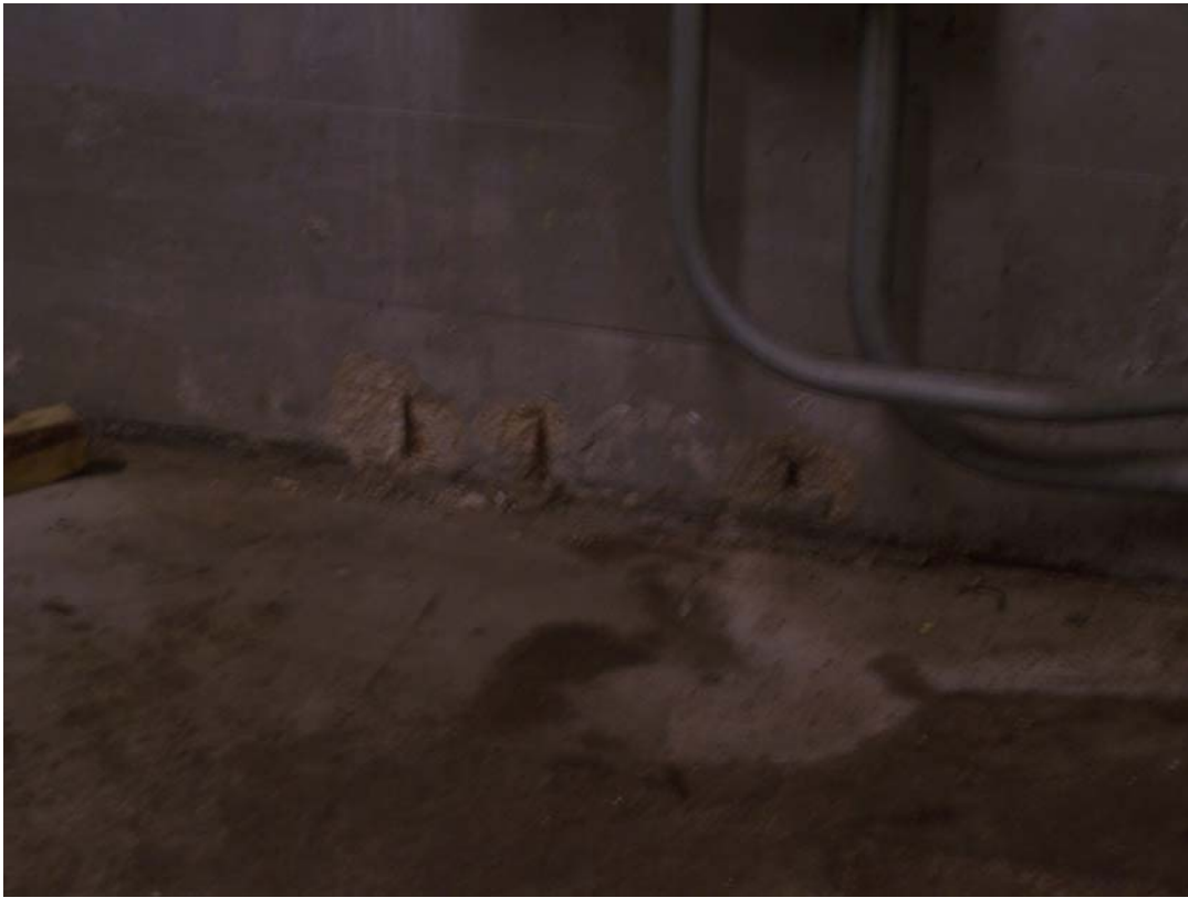
Photo 153 Popouts in Room 2 caused by corroding steel.
