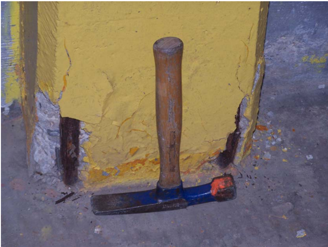
Photo 106 Bottom of column in the wall in room 5. Delamination continues up the column.
