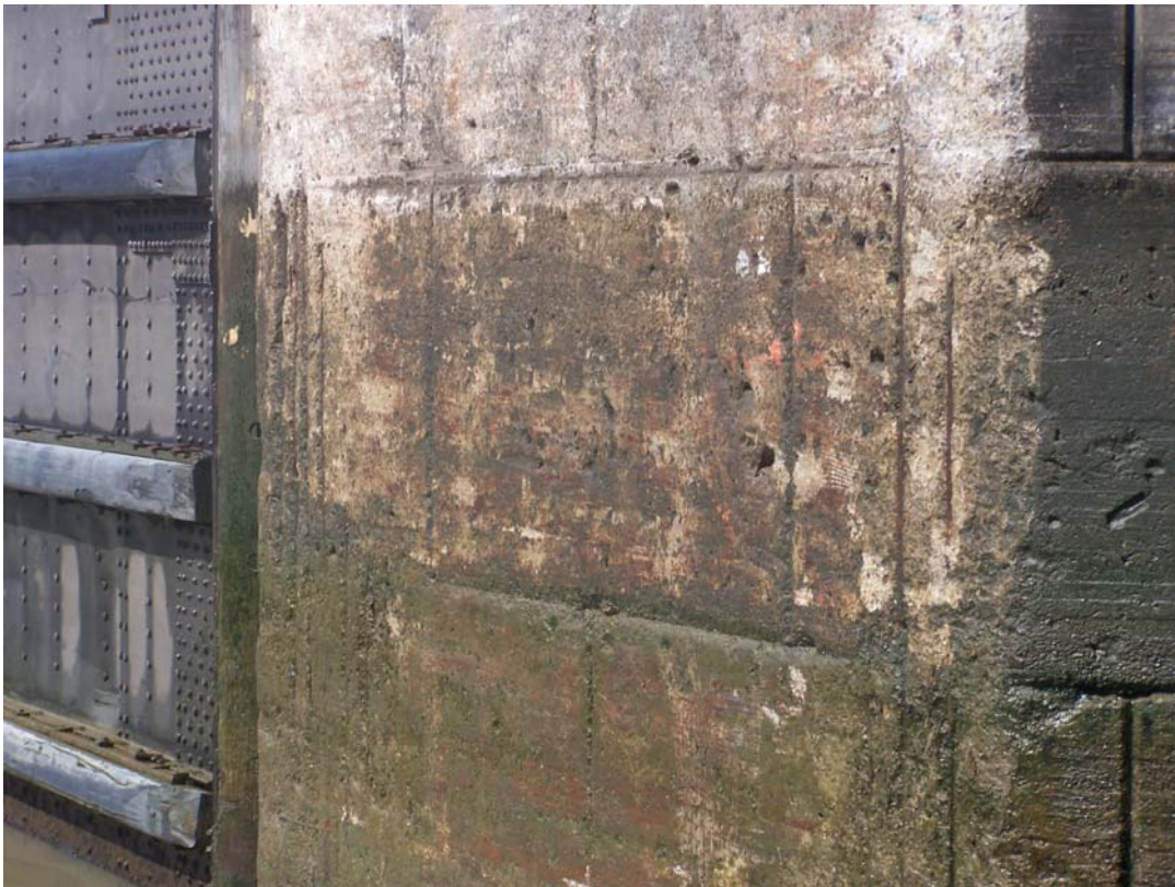
Photo 188 Northwest gatebay wall between the gates.
