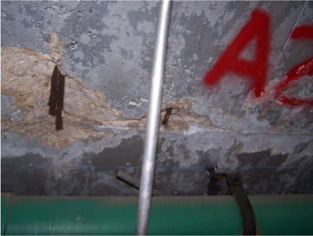
Photo 55 Spalling with corroded steel in ceiling over gate 3 machinery.
