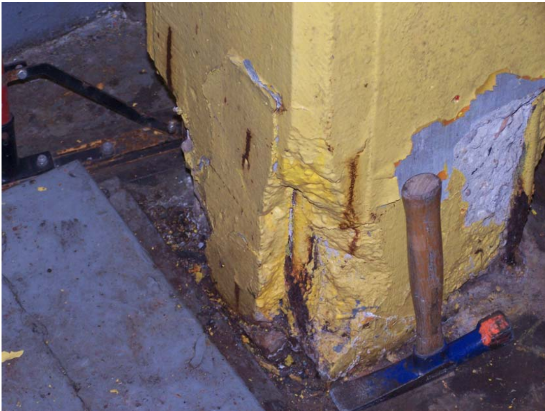
Photo 110 Spalling and corroded steel at the bottom of the column near the louvers by the hinge of gate 5. Damage to about 20" up from floor.
