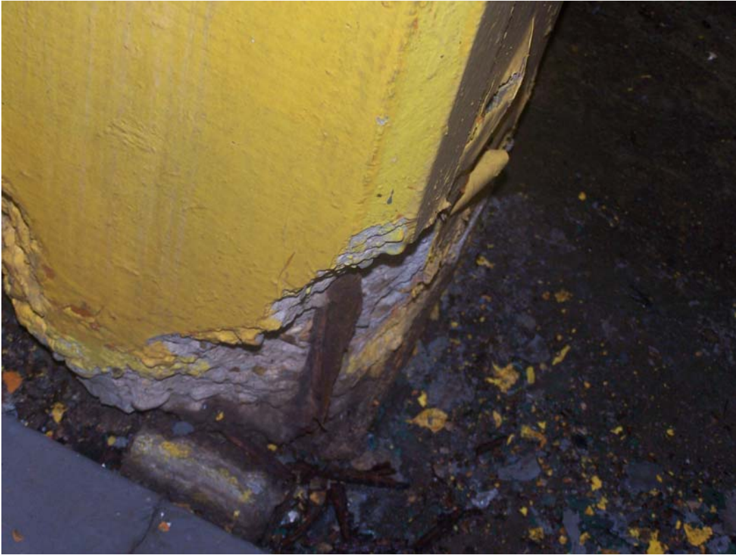
Photo 175 Large spalls with corroded steel in the bottom of the column near the hinge in Room 6.
