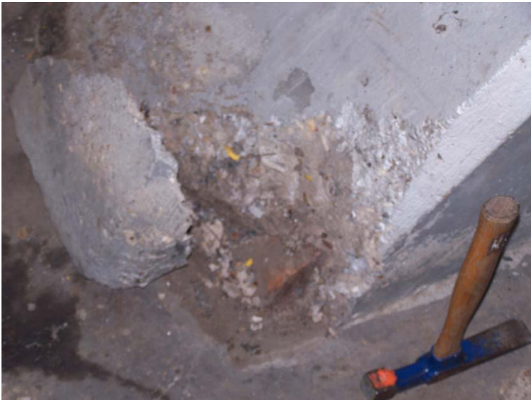
Photo 38 Large spall with exposed steel near the hinge for Gate 3.
