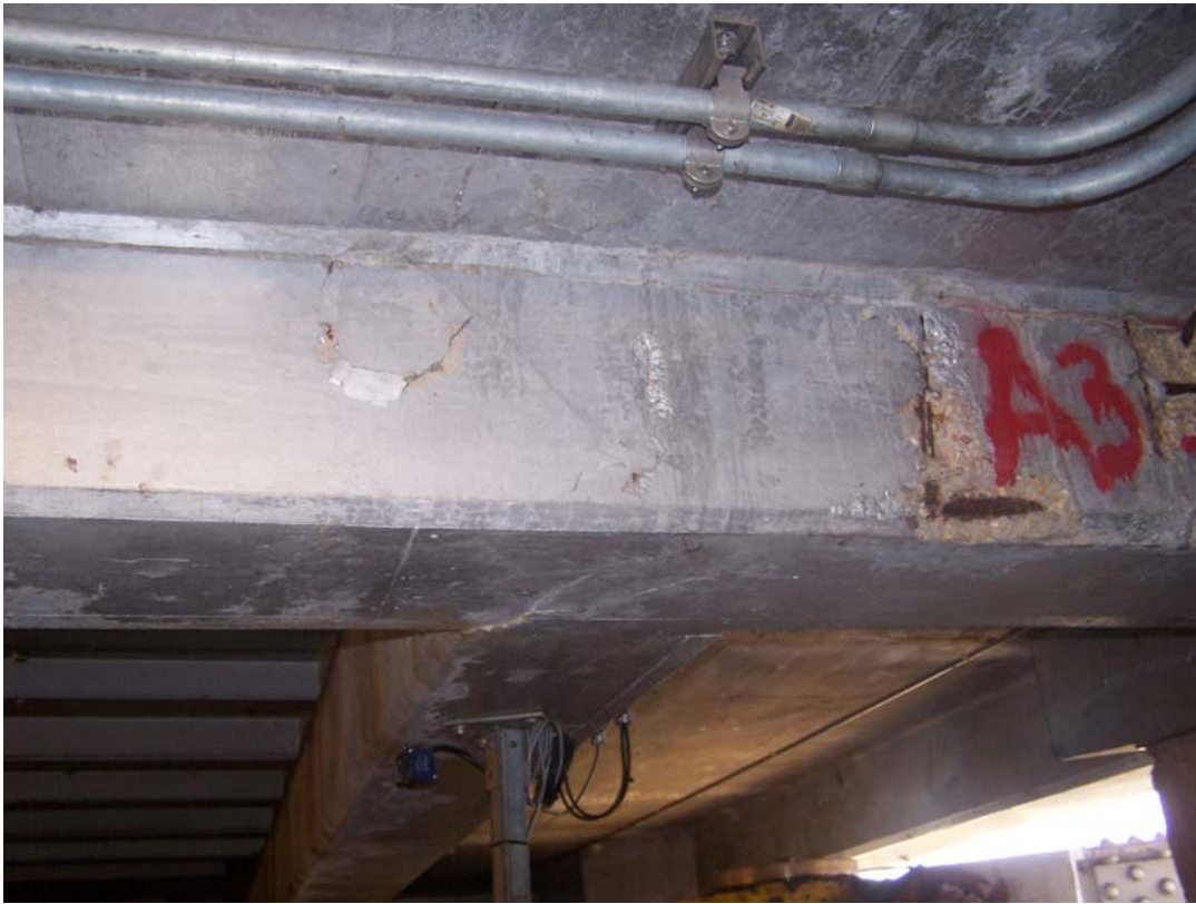
Photo 159 Spalling and corroding steel in beam in Room 2.
