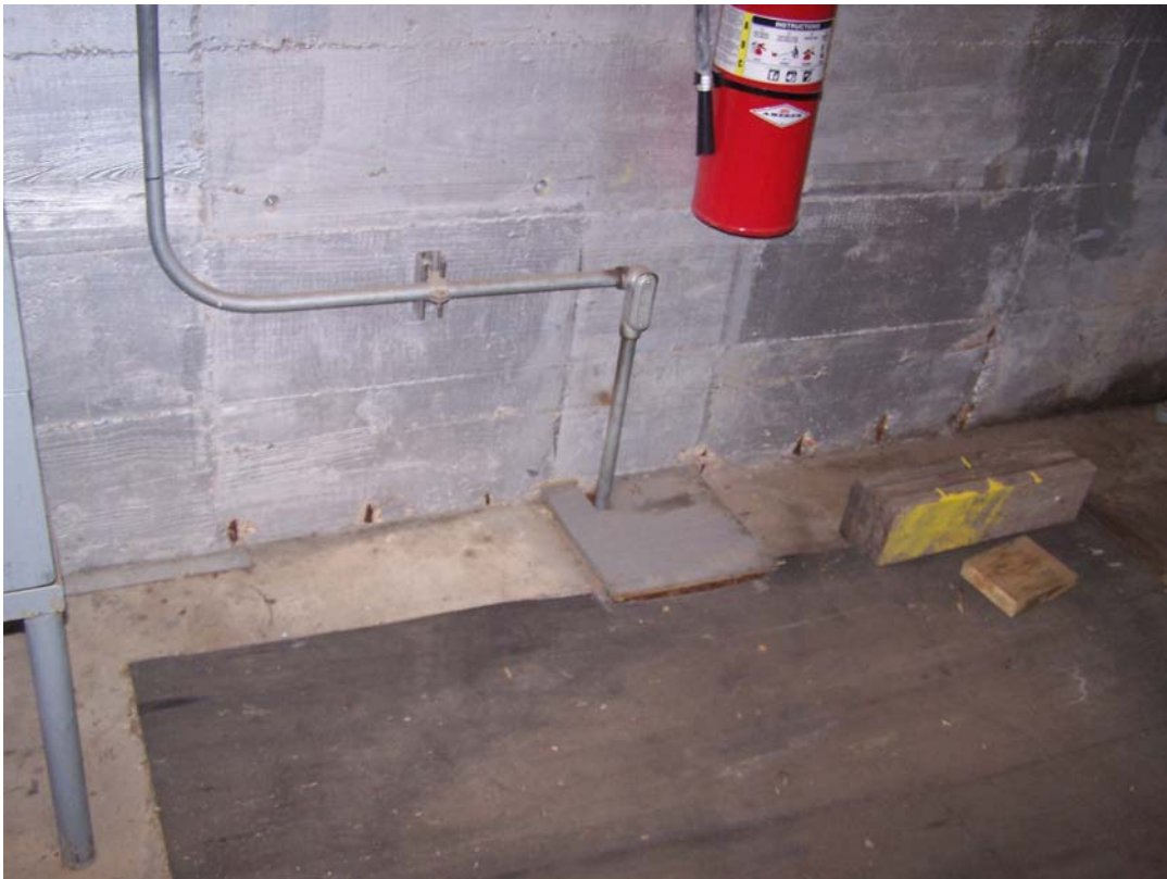
Photo 118 Popouts along the bottom of the wall near valves 15 and 16.
