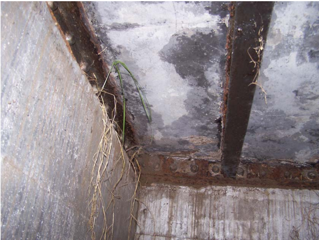
Photo 70 Bottom of hatch cover in west tunnel.
