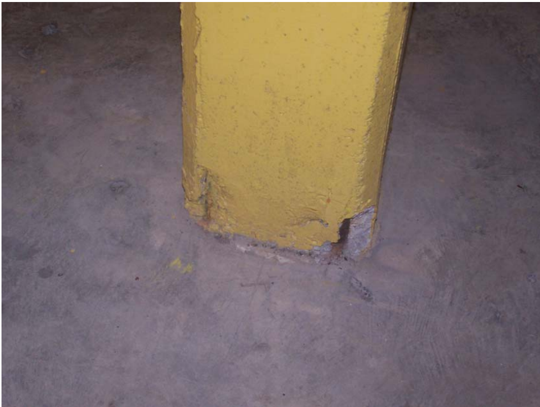
Photo 166 Spalled corners at the bottom of column in Room 2 near the tunnel.
