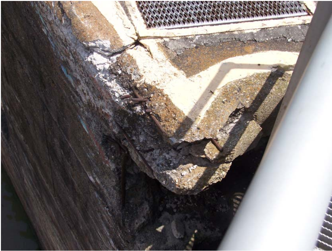
Photo 133 Spalled concrete and exposed steel near hinge of northeast gatebay.
