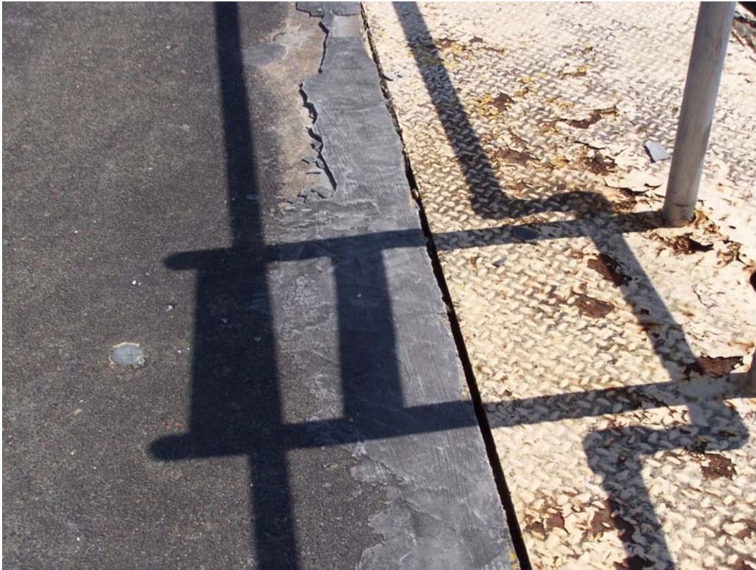
Photo 33 Failing patch material around the steel plate over the bulkhead recess on the west river side.
