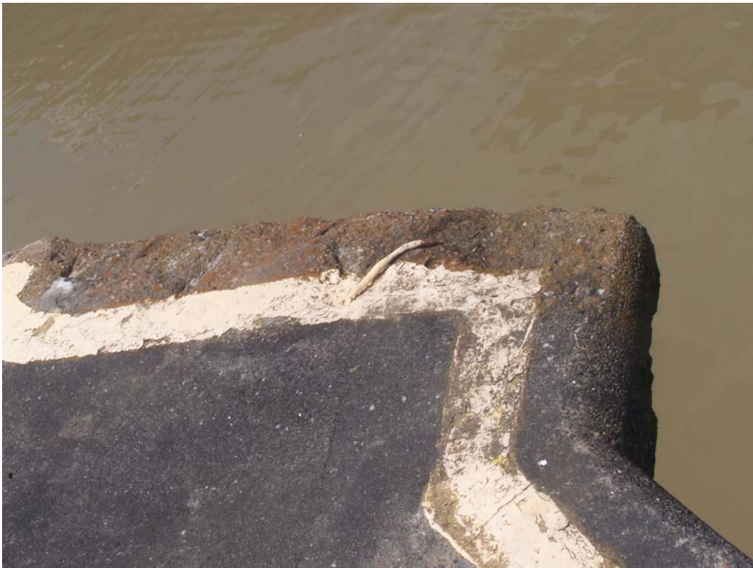
Photo 145 Spalls in north gatebay.
