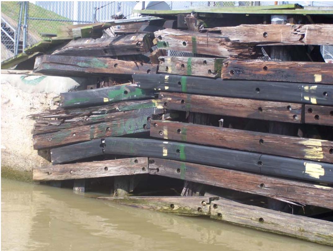
Photo 186 Damage to south end of the northwest guidewall.
