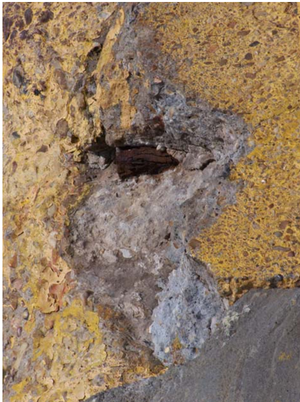
Photo 12 Spalls in top of the west chamber wall near control house.
