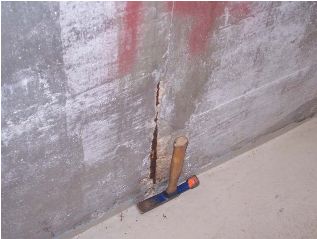
Photo 74 Popout in the bottom of west tunnel wall.
