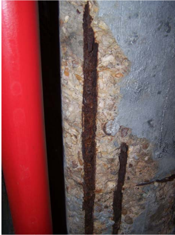
Photo 41 Spalled beam near valve 11. Bottom steel and spiral wire severely corroded.
