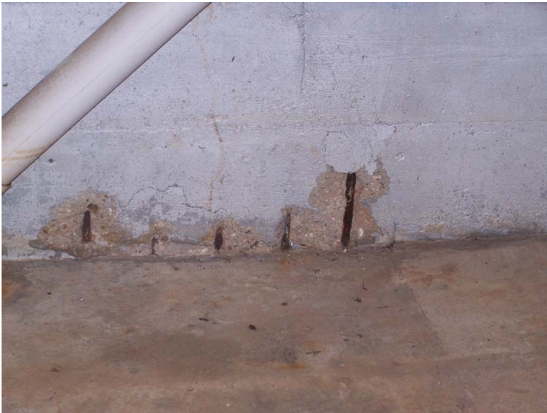
Photo 86 Popouts at the bottom of the wall in room 5.
