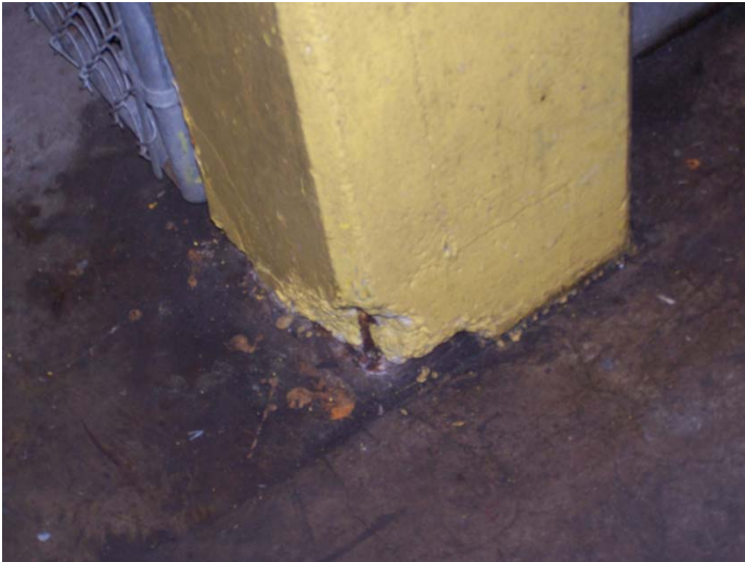
Photo 109 Spall at the bottom of the column by the gate under the stairway.
