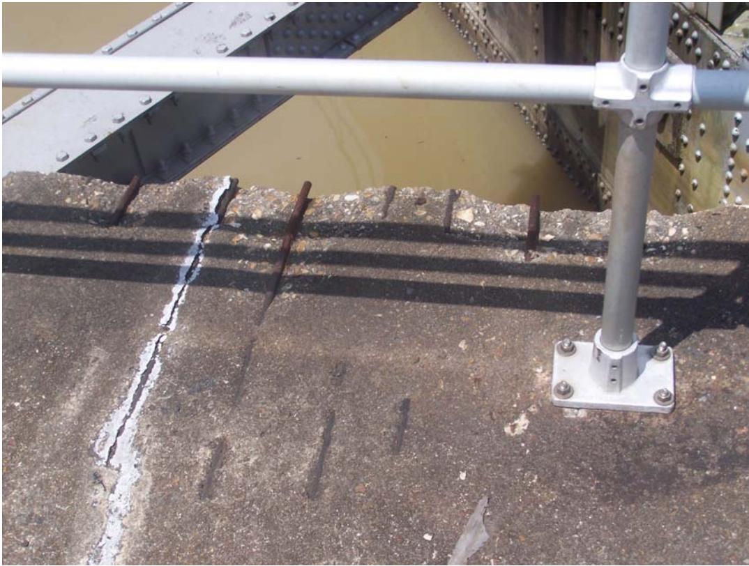
Photo 151 Spalling with exposed steel near the river side gate hinge.
