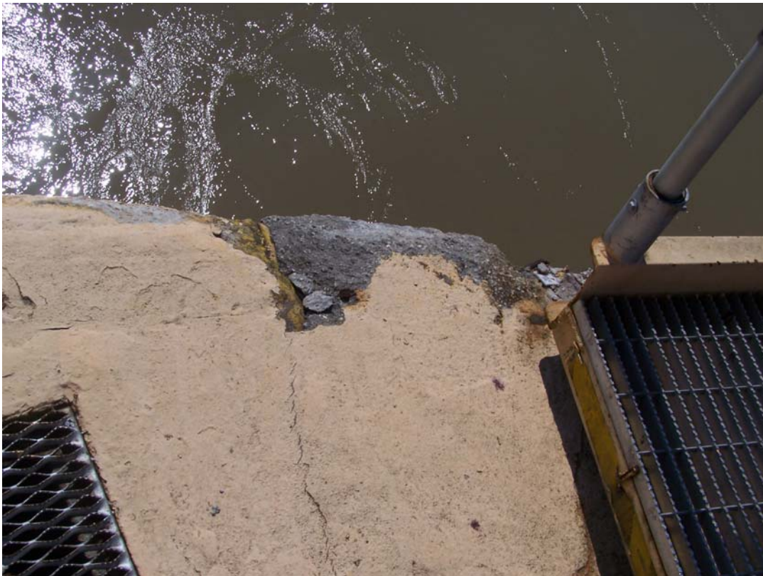
Photo 28 Spall in top of west wall near the hinge for the river side gate.
