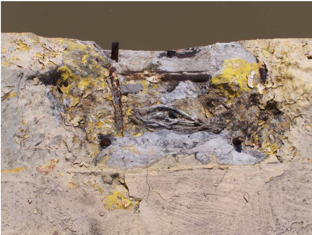
Photo 22 Large spall with corroded steel on top west chamber wall.
