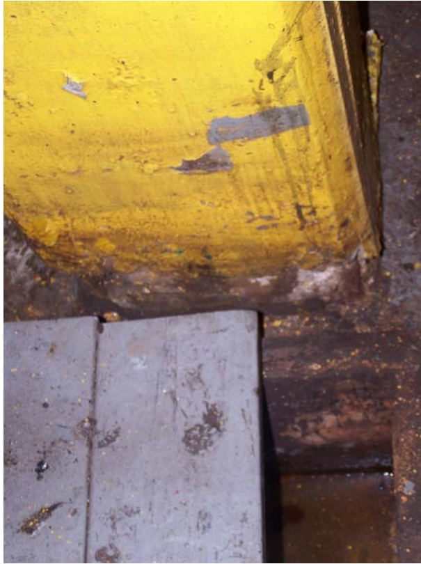
Photo 47 Spalls and delaminations at bottom of columns on both sides of hinge for gate 1.
