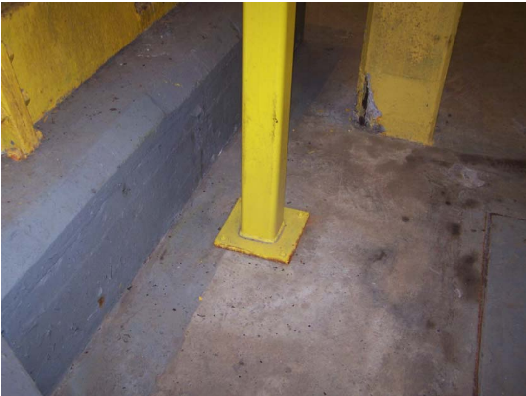
Photo 96 Spall at bottom of column and steel column added to support deteriorated concrete beams and columns.
