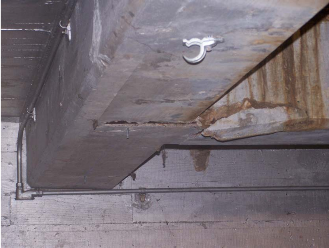
Photo 173 Spalls and corroded steel in beams over machinery in Room 6.
