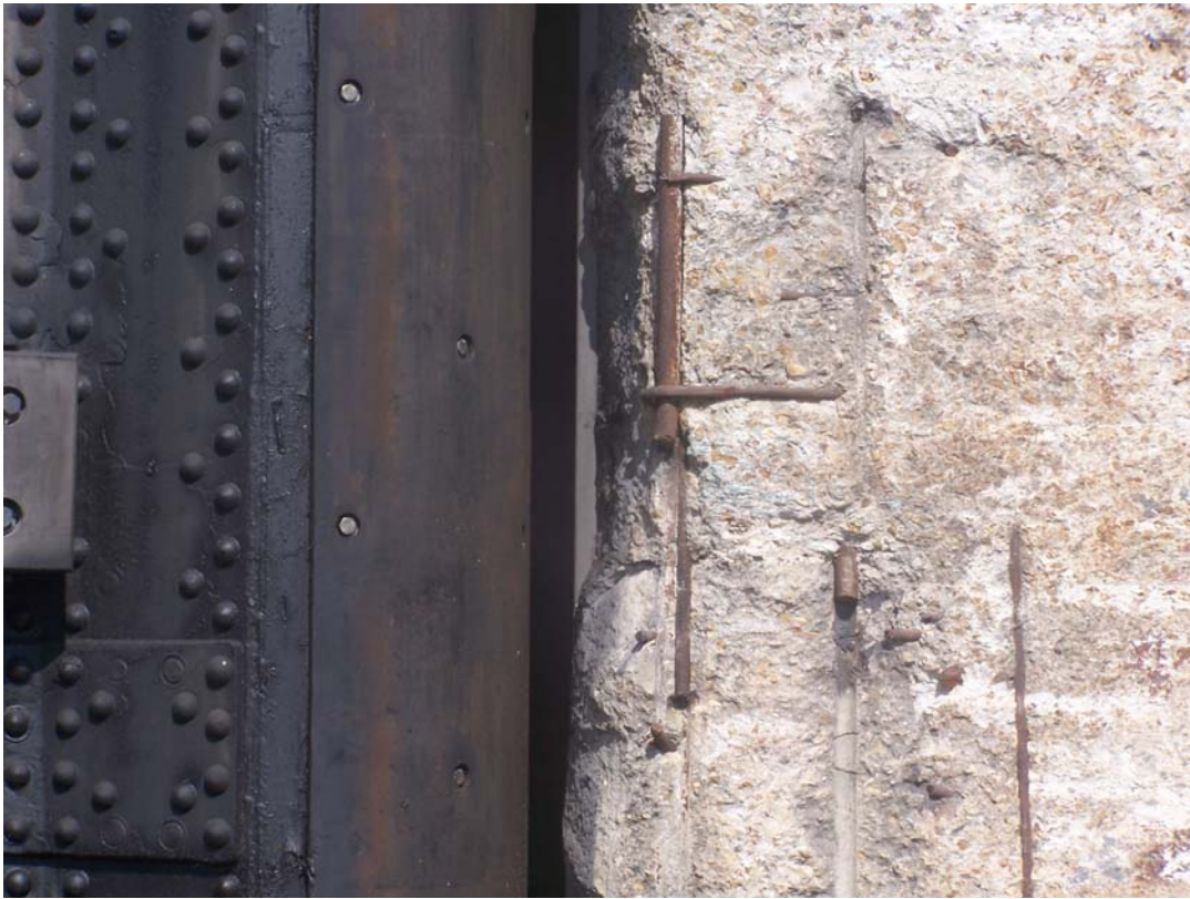
Photo 189 Spalled corner with exposed steel near the hinge for the southwest gate.
