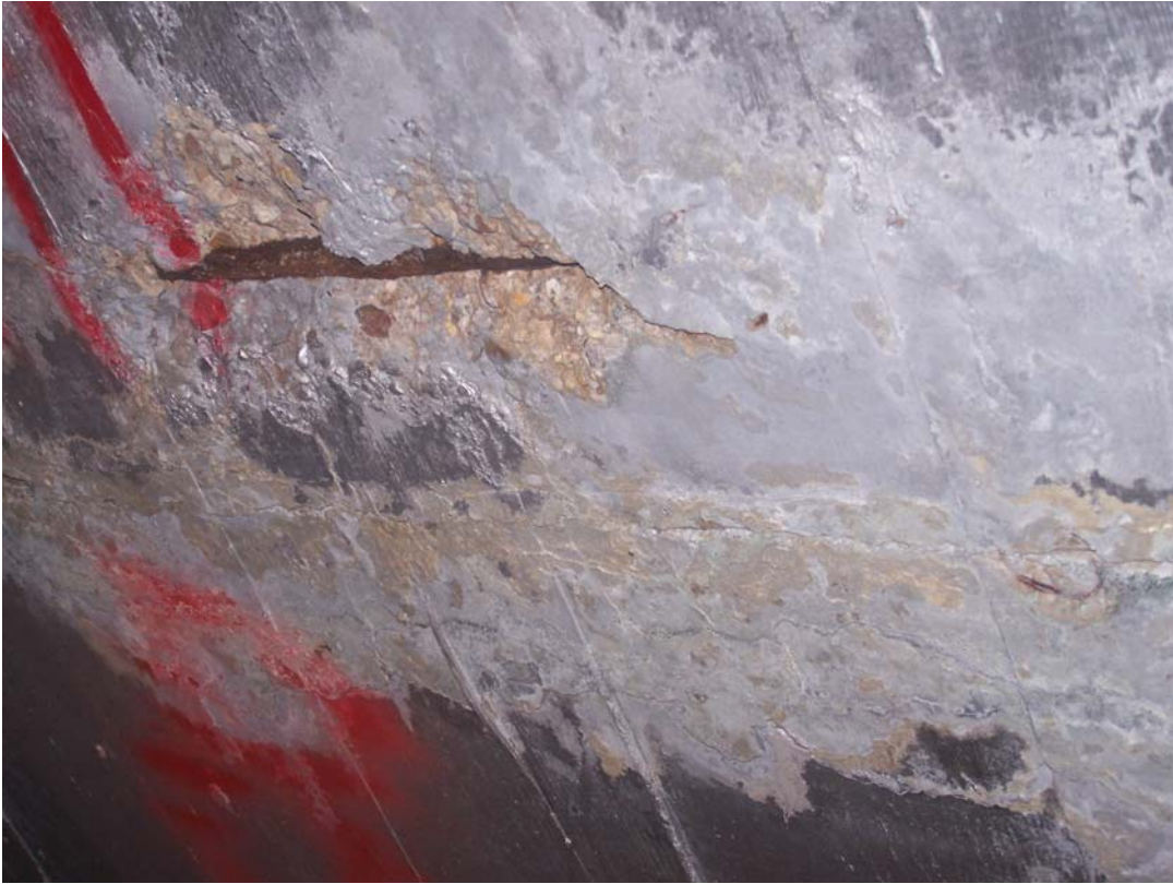
Photo 171 Spalling and exposed steel in ceiling of room 6.
