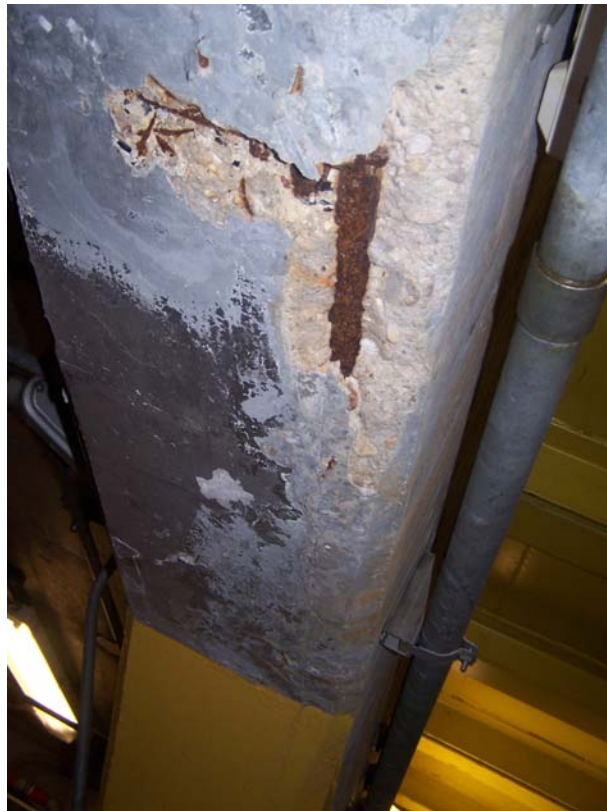
Photo 104 Spall with corroded steel in bottom of beam in room 7.
