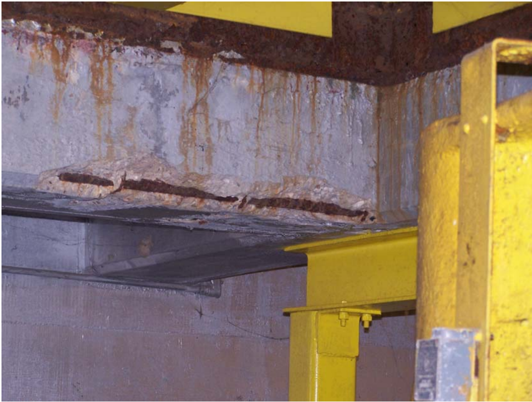
Photo 97 Spalls and corroded steel in beams over machinery in room 5. Note steel beam and columns added to support these beams.
