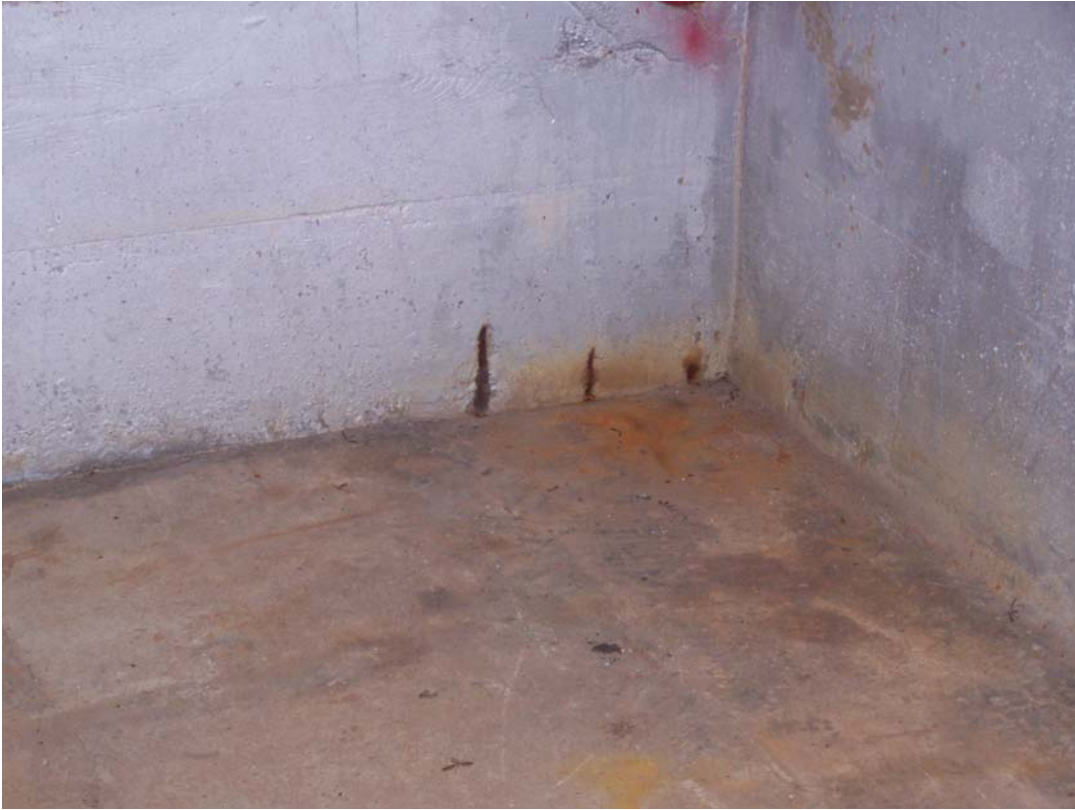
Photo 87 Popouts at the bottom of the wall in room 5.
