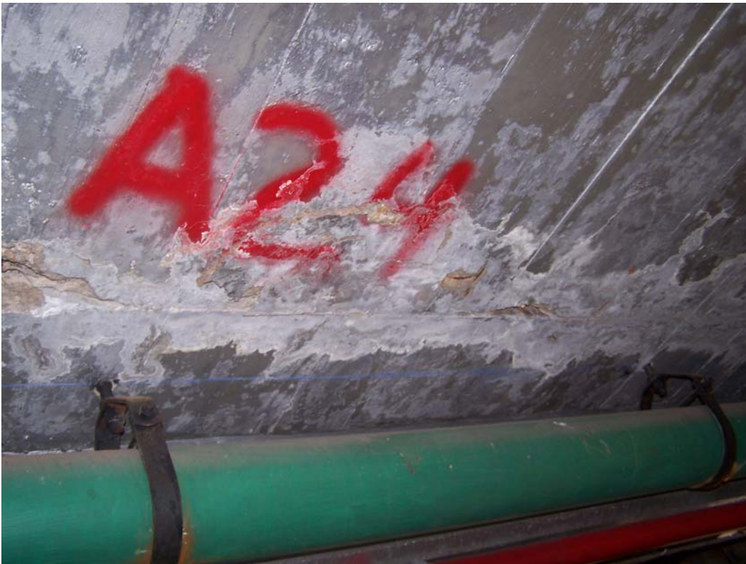
Photo 56 Spalling with corroded steel in ceiling over gate 3 machinery.
