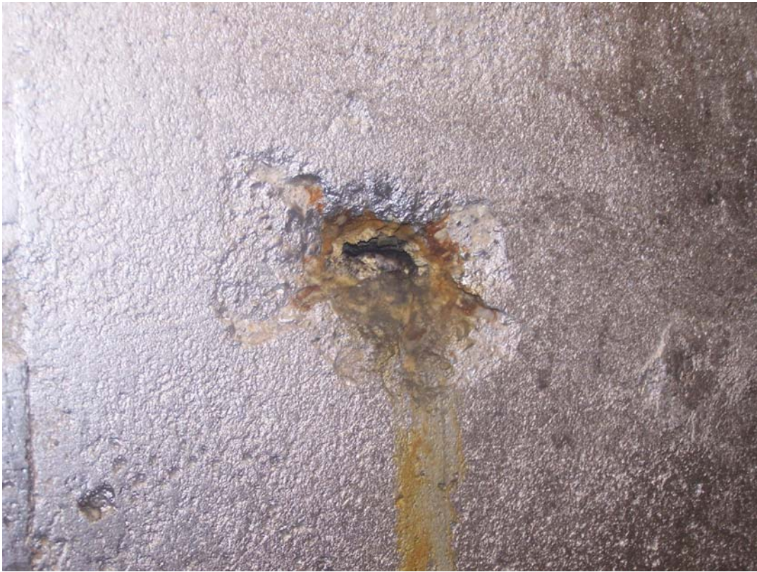
Photo 167 Small popout due to clay in east tunnel.
