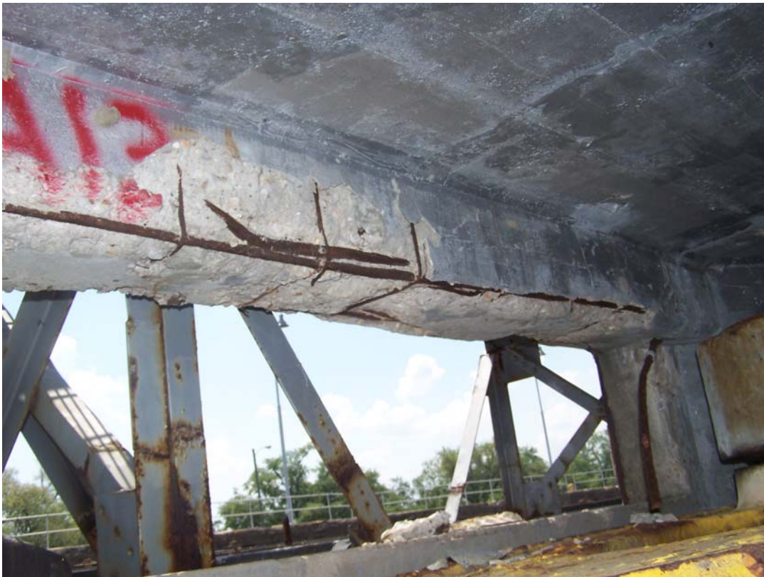
Photo 100 Spalled beam with corroded reinforcing over opening for gate 7.
