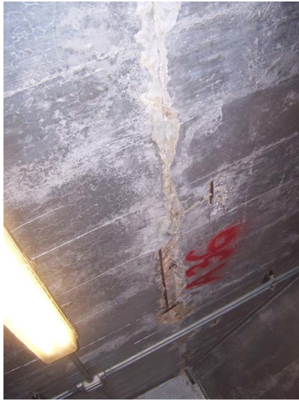
Photo 157 Spalls and popouts with corroded steel in ceiling of Room 2.
