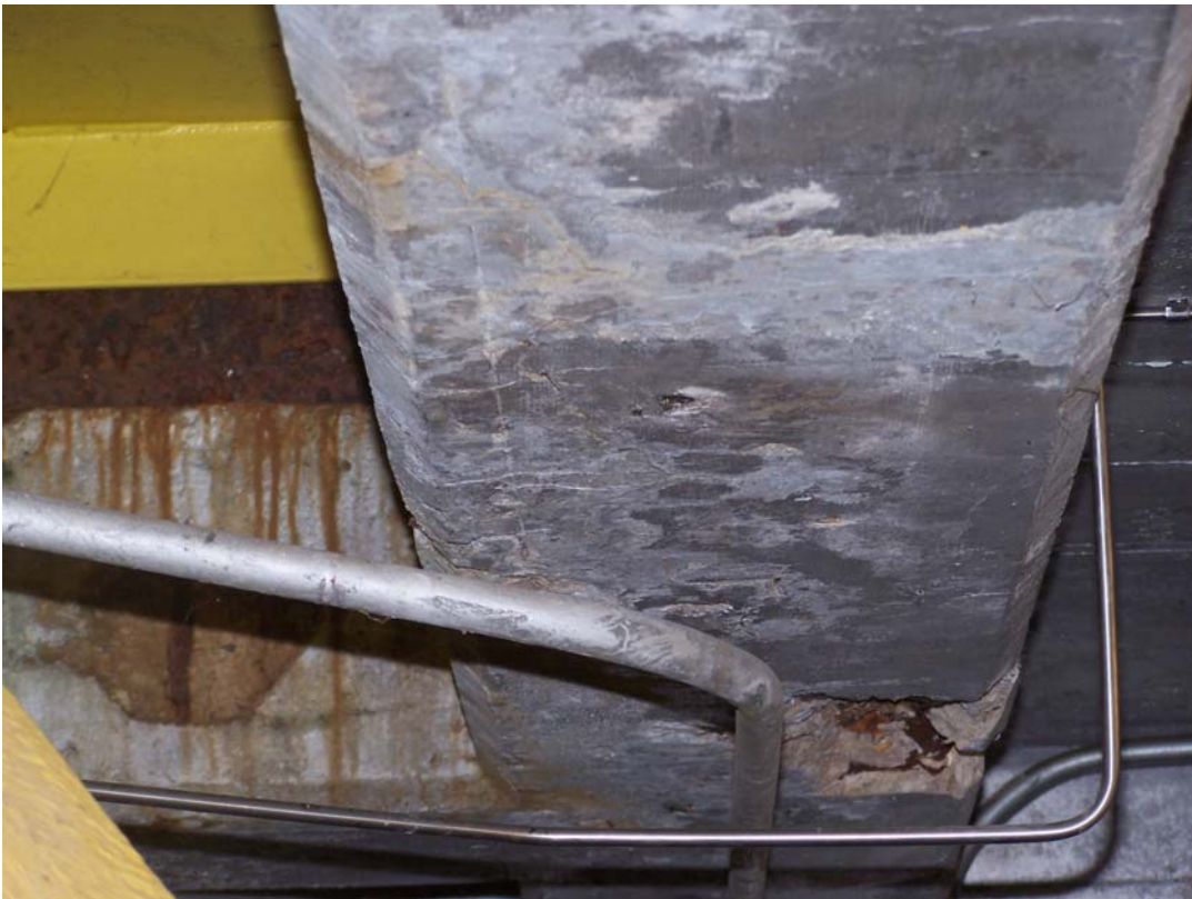
Photo 122 Spall and corroded steel in beam over gate 5 machinery.
