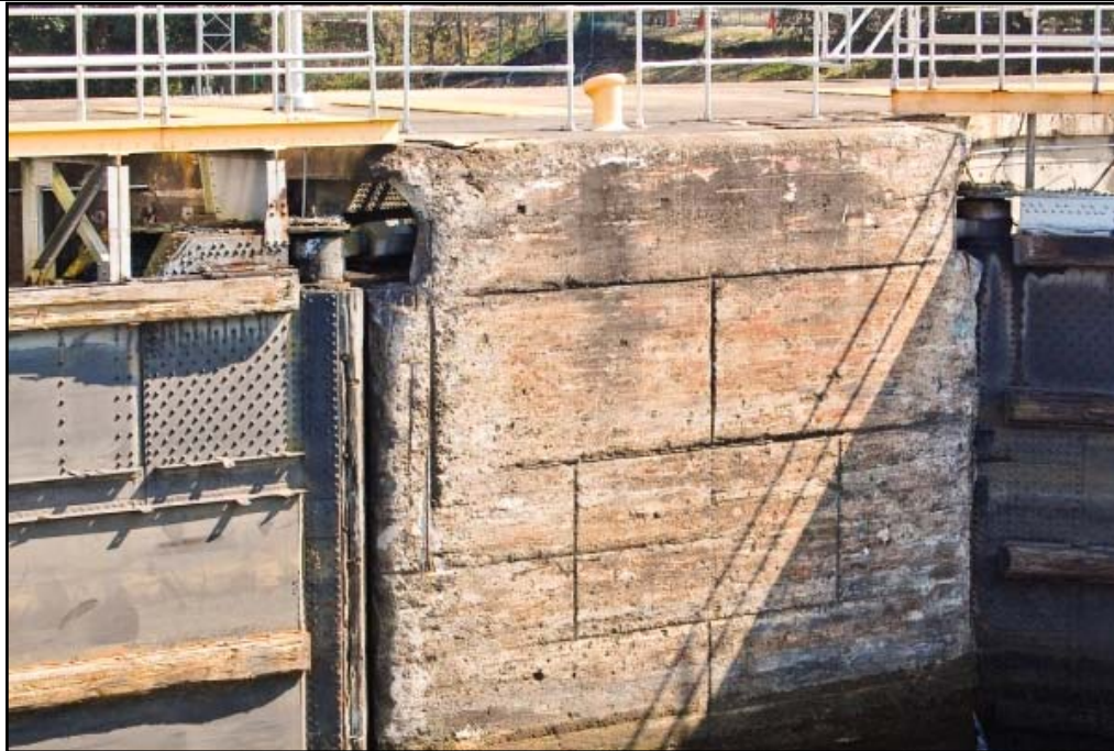
Spalding concrete and exposed rebar on corners of gate bays and top edge of lock wall deck, image is of east wall gate recesses but is typical of all eight gate recesses.
