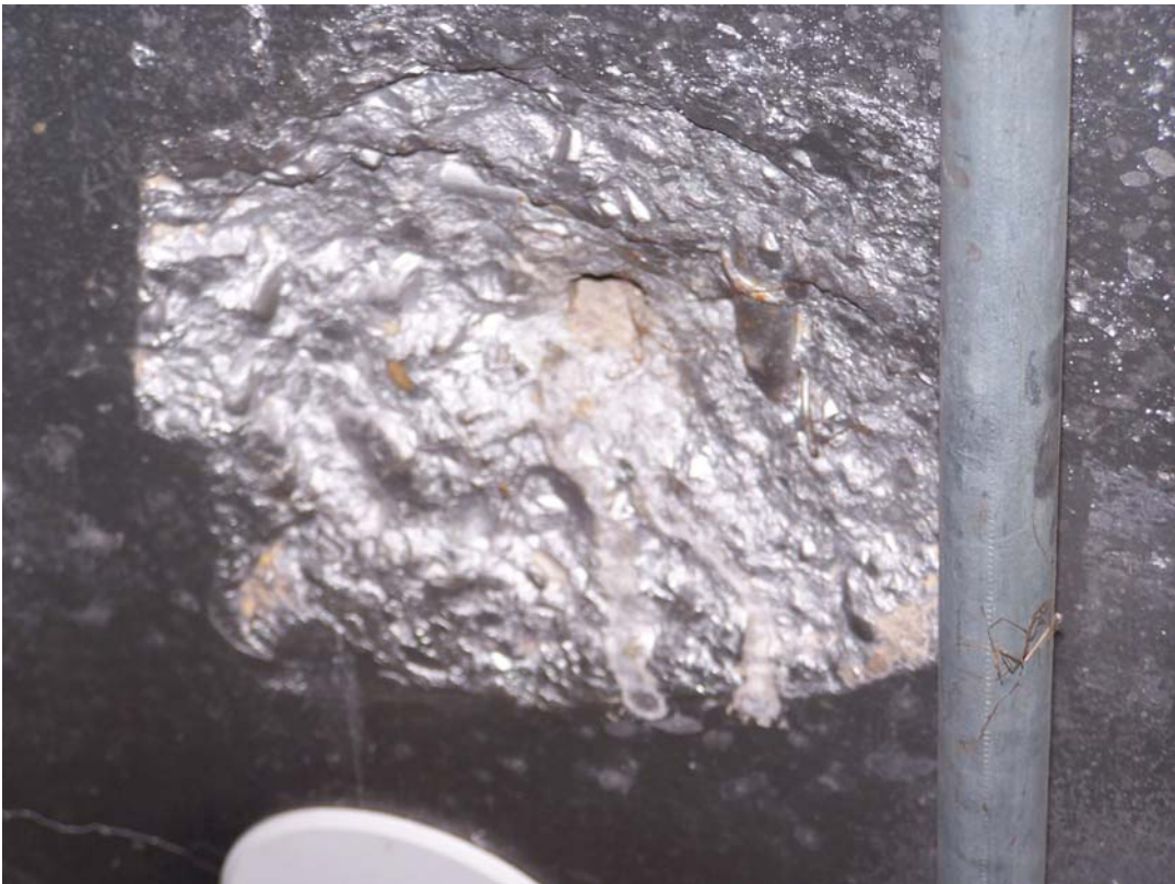
Photo 52 Popout in beam over gate 1 machinery.
