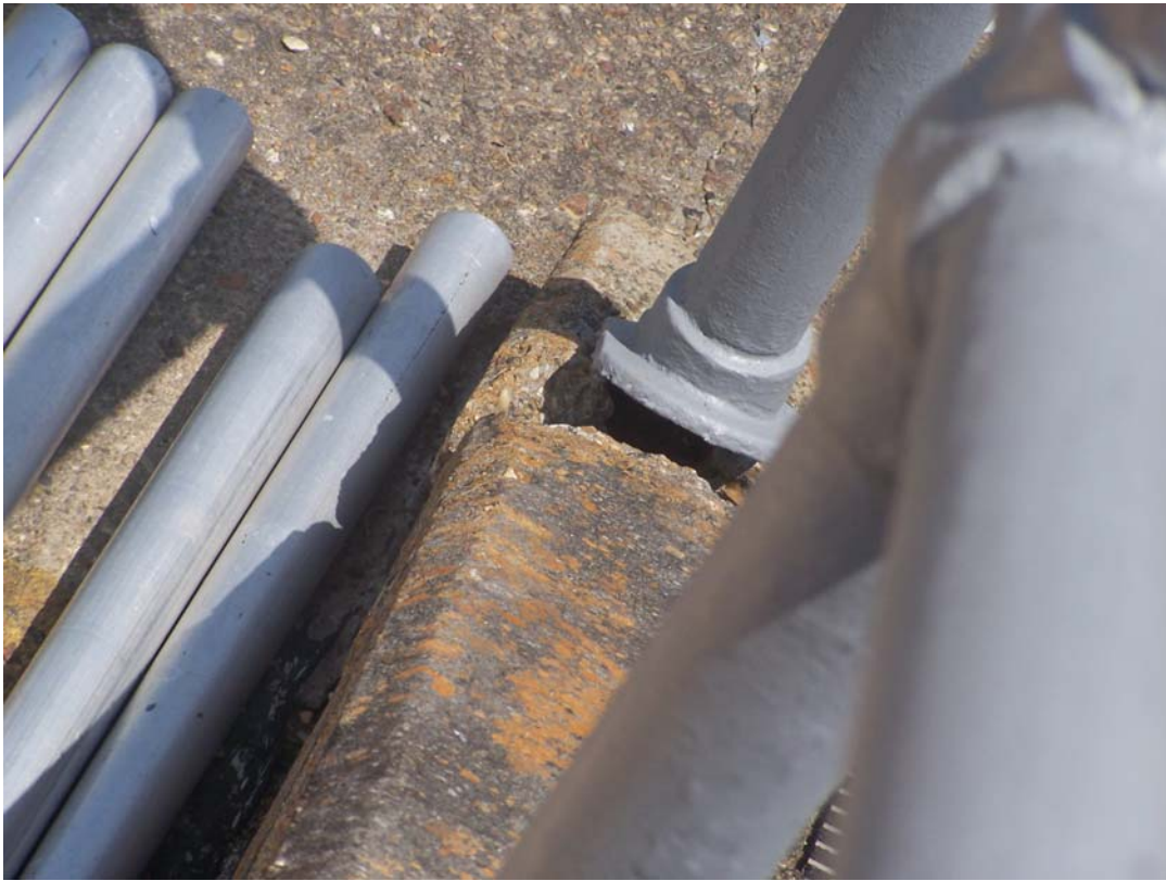
Photo 141 Spall where handrail post embeds in stairway wall. Handrail is loose.
