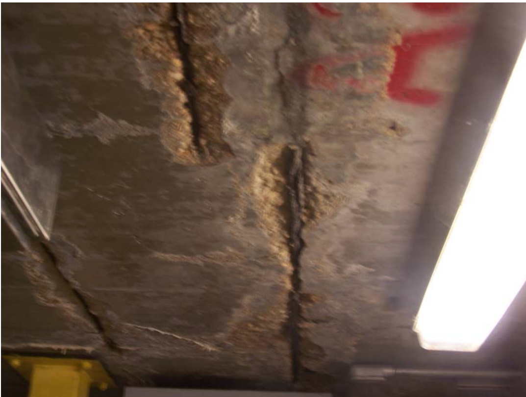
Photo 58 Spalls and popouts in the ceiling of room 3.
