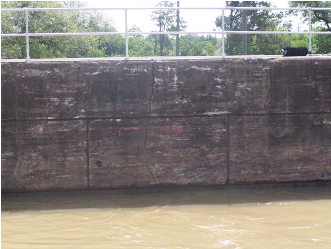
Photo 202 Crack in east chamber wall. (Typical of cracks in chamber walls).
