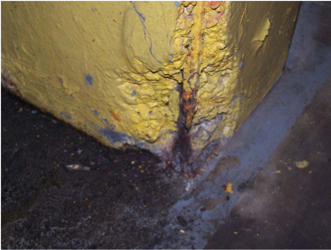
Photo 37 Spall with corroded steel at the bottom of a column in machinery room #3.
