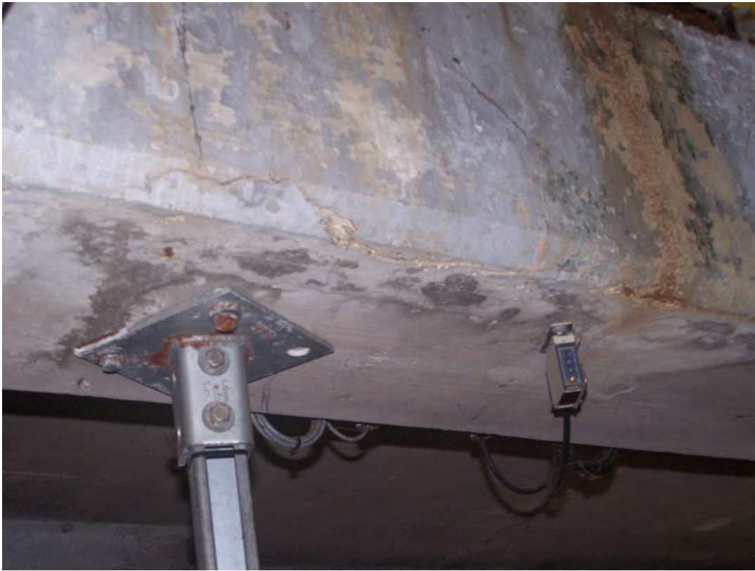
Photo 161 Crack in beam over Gate hinge.
