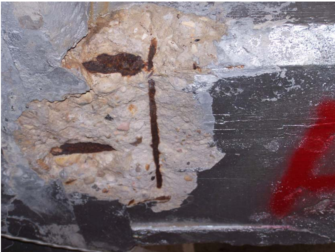
Photo 98 Spall with corroded steel in beam over machinery in room 5.
