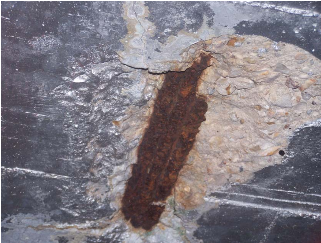
Photo 168 Large spall caused by corroding reinforcing in ceiling of machinery room 6.
