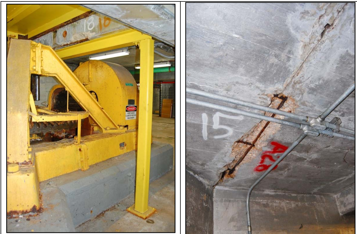
Steel beam and steel support column placed to reinforce failing concrete deck beam.
