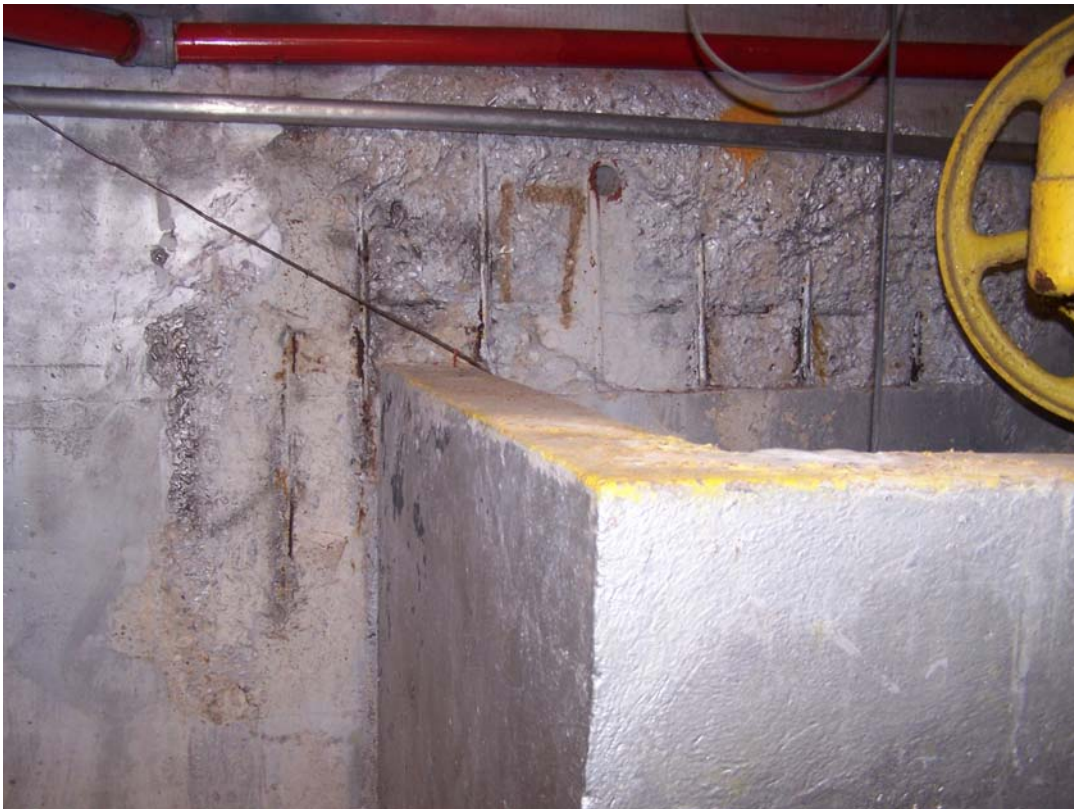
Photo 84 Large spalled area of wall in room 5. Corrosion and spalling continue.
