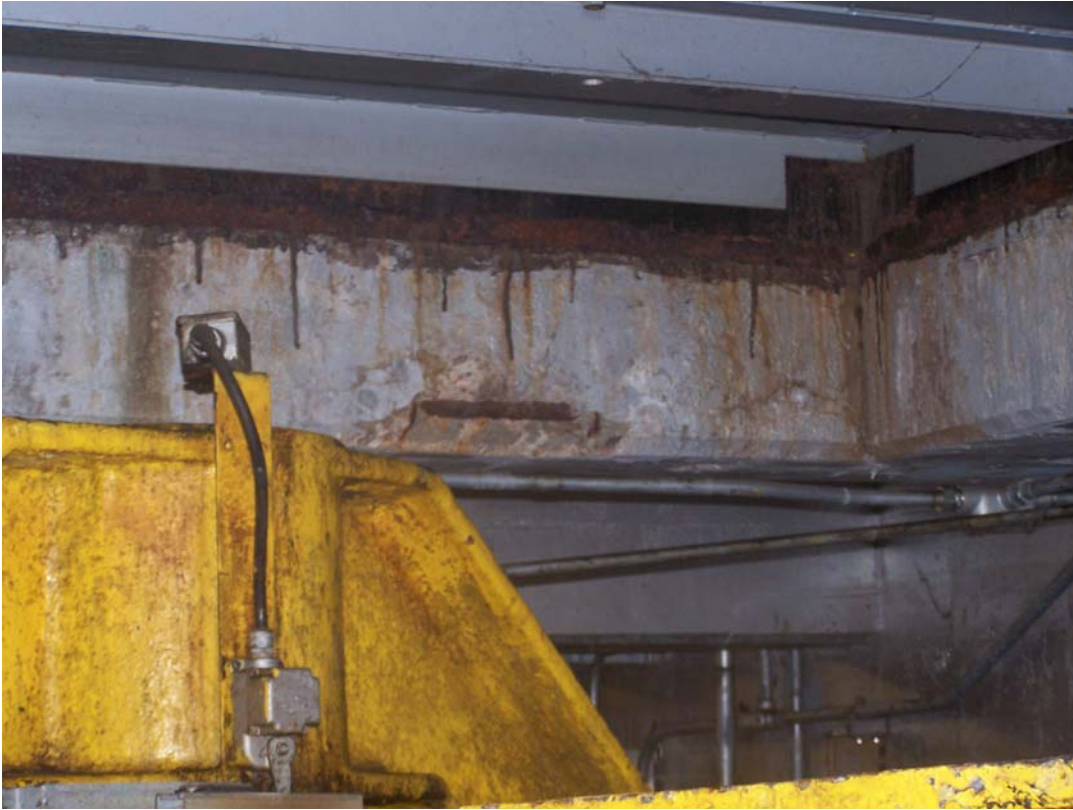
Photo 155 Spall with corroded steel in beam in over machinery for Gate 2.
