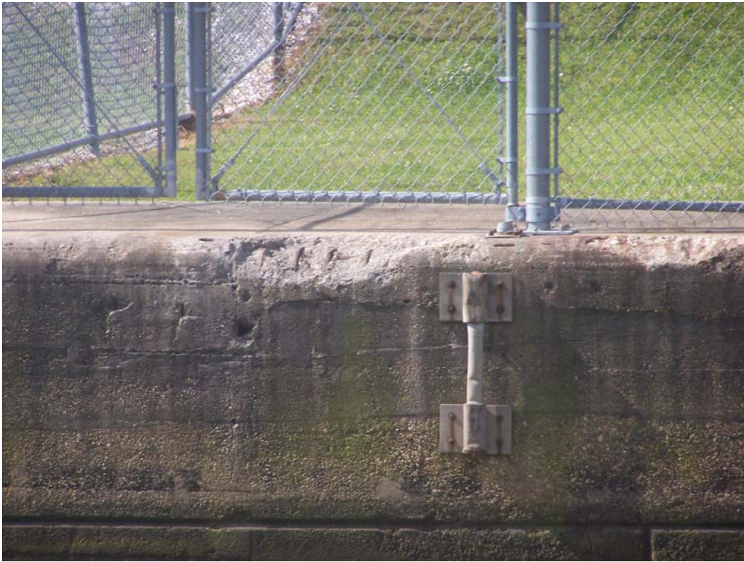
Photo 185 Cracks and spalling in the retaining wall on the northeast side.
