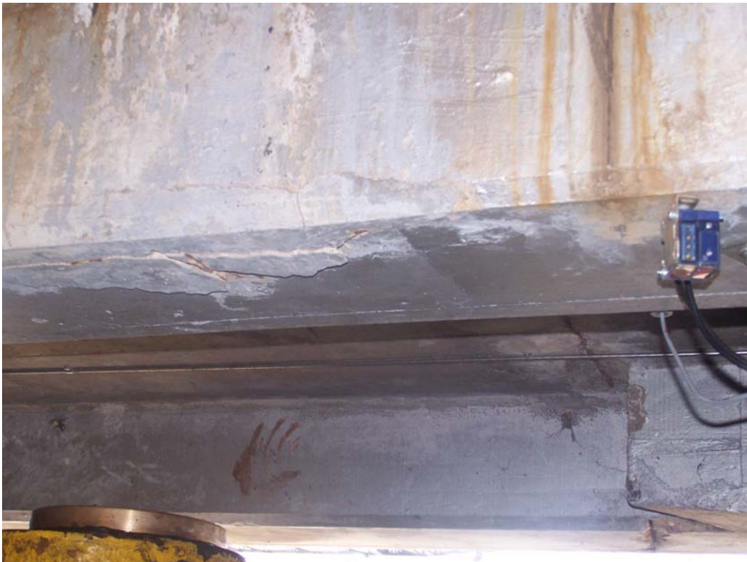
Photo 160 Crack in beam in Room 2.
