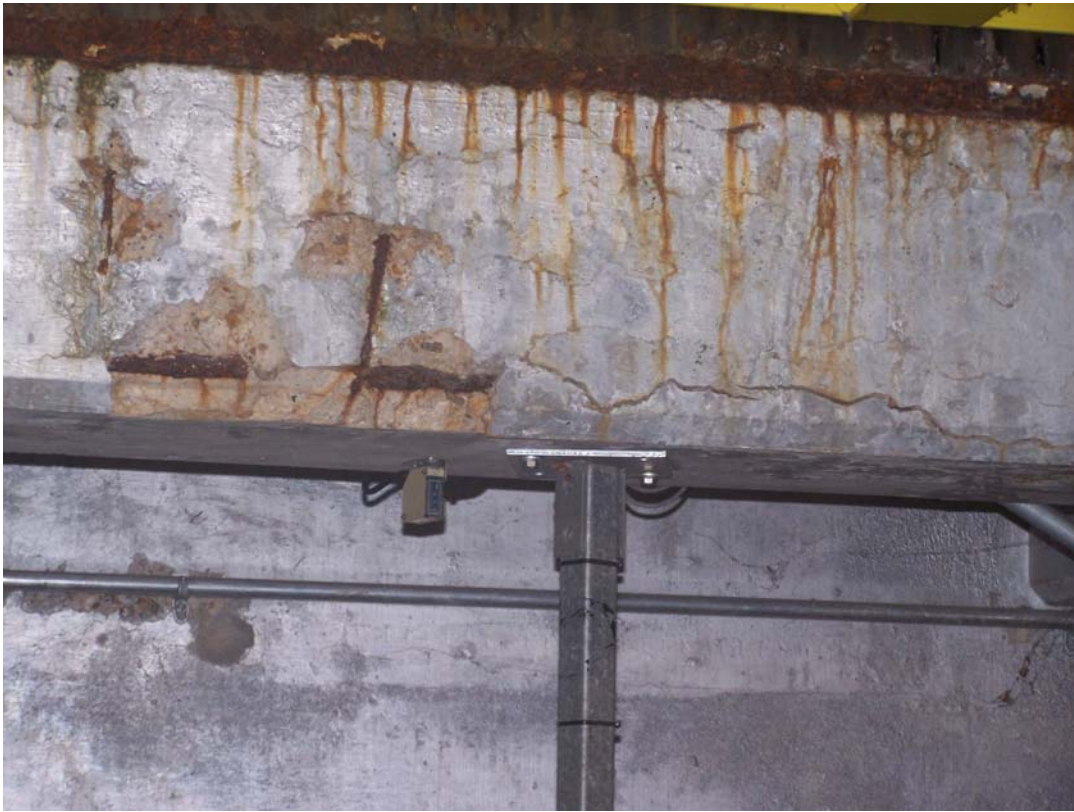
Photo 163 Spall with corroded steel and crack in beam over gate 4.
