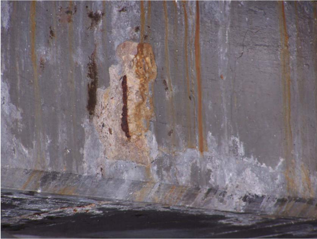
Photo 51 Popout in beam over gate 1 hinge.
