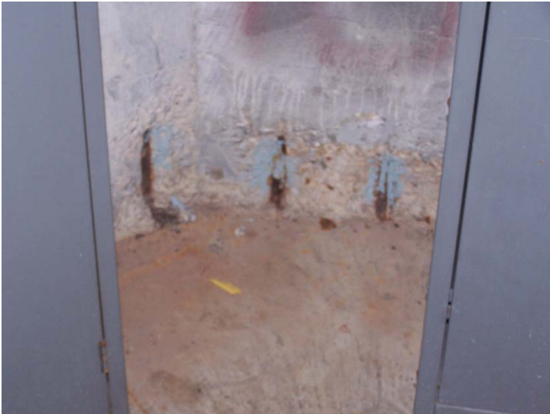
Photo 65 Popouts at the bottom of the wall in room 3.
