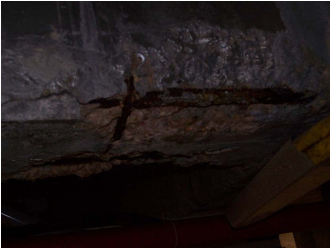
Photo 40 Spalled beam near valve 11. Bottom steel and spiral wire severely corroded.
