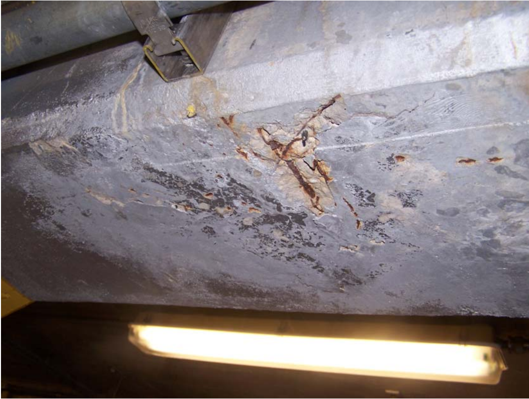
Photo 103 Crack and spall in the bottom of beam in room 7.
