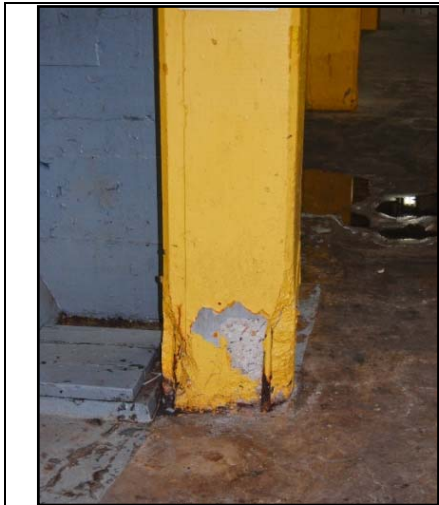
Deck support column in NW machinery room.
