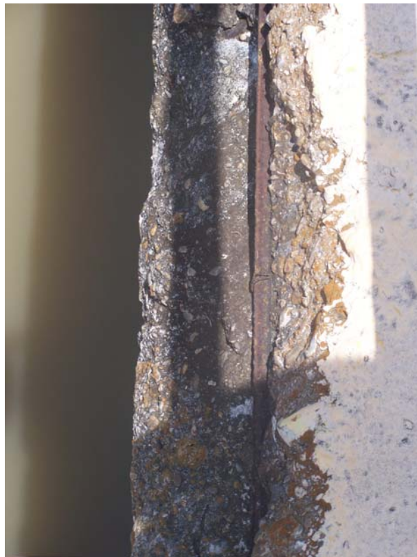
Photo 148 Spalls in east lock chamber wall. (Typical).
