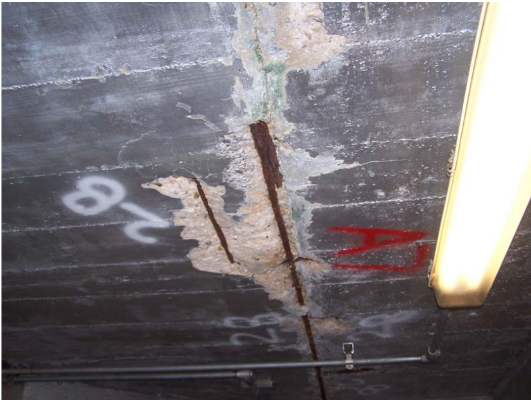
Photo 120 Spalls in ceiling near gate 5.
