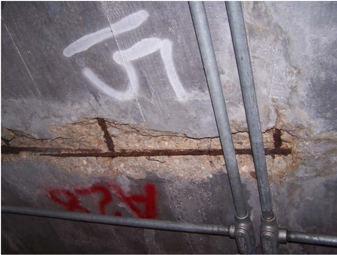
Photo 45 Spalls in ceiling near valve 11 caused by corroding steel. Further deterioration since last inspection.
