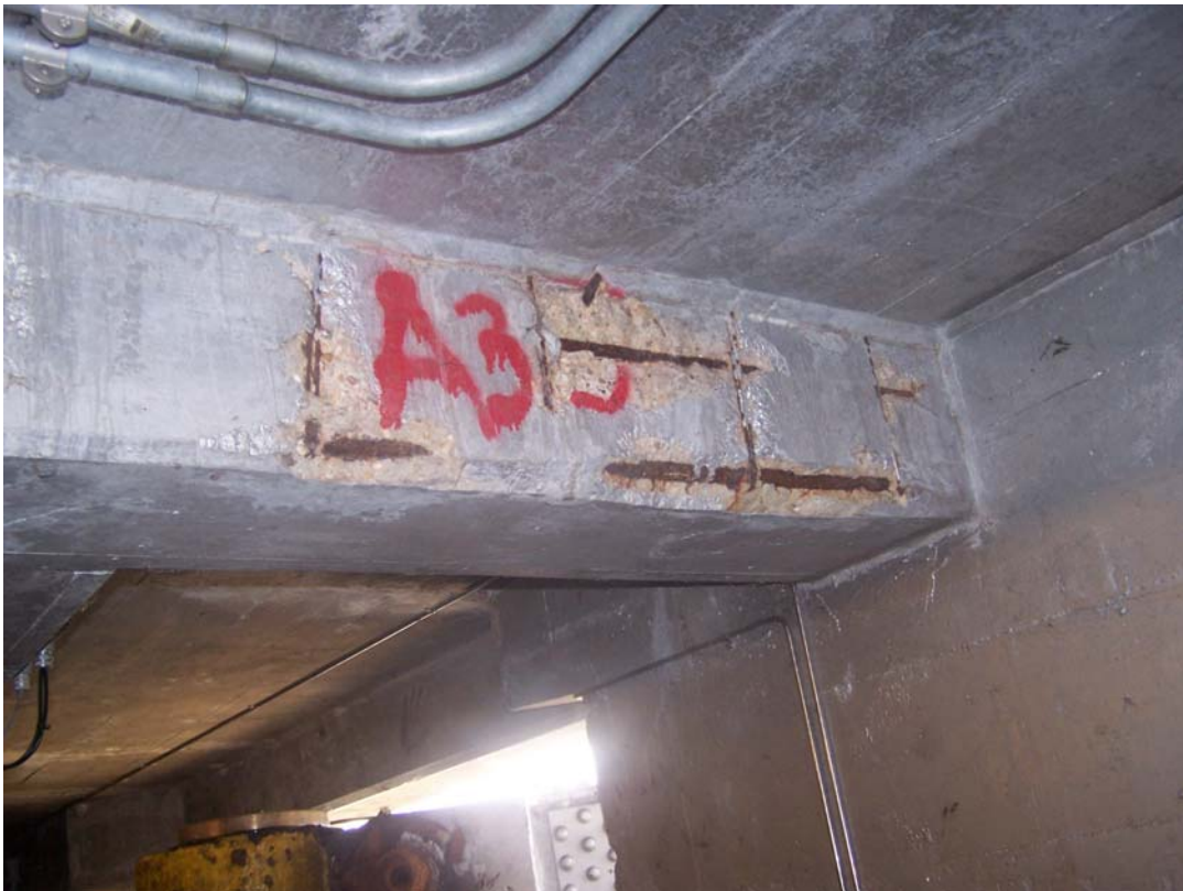
Photo 158 Spalling and corroding steel in beam in Room 2. Further spalling has occurred since last inspection.
