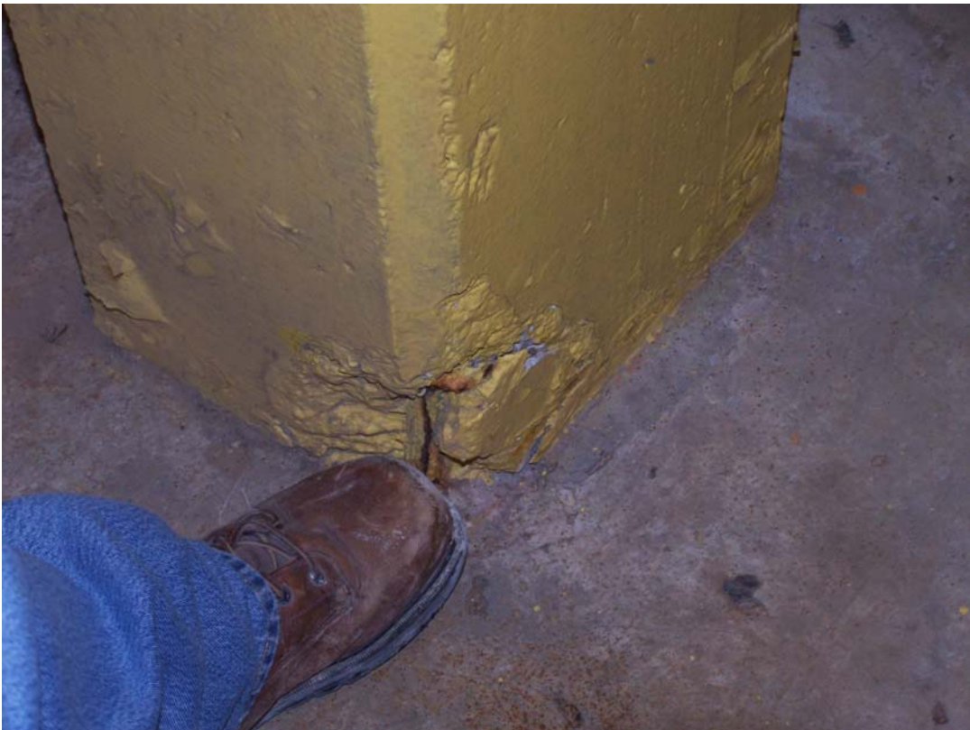
Photo 88 Spall at the bottom of column in Room 5.
