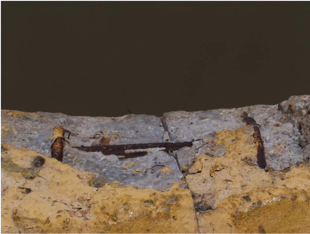
Photo 15 New spall with exposed steel in top of west chamber wall.
