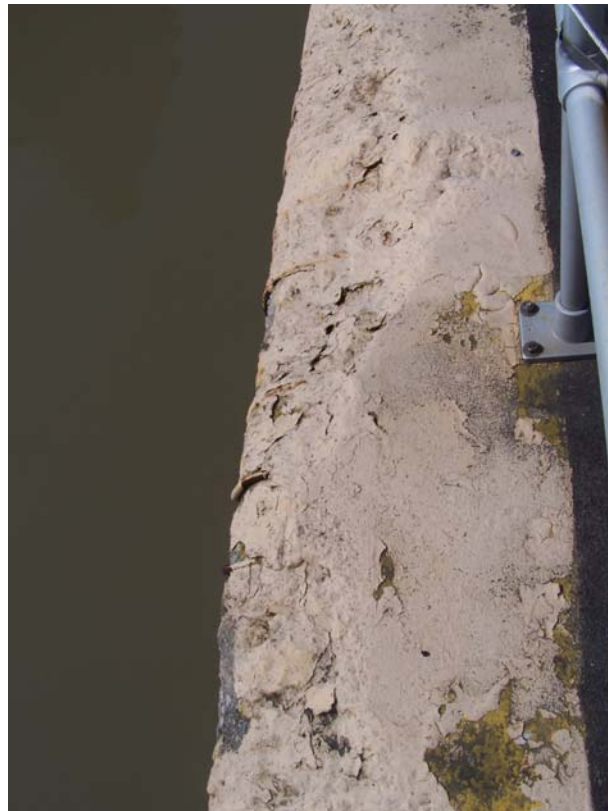
Photo 32 Spalls in west river side gatebay.
