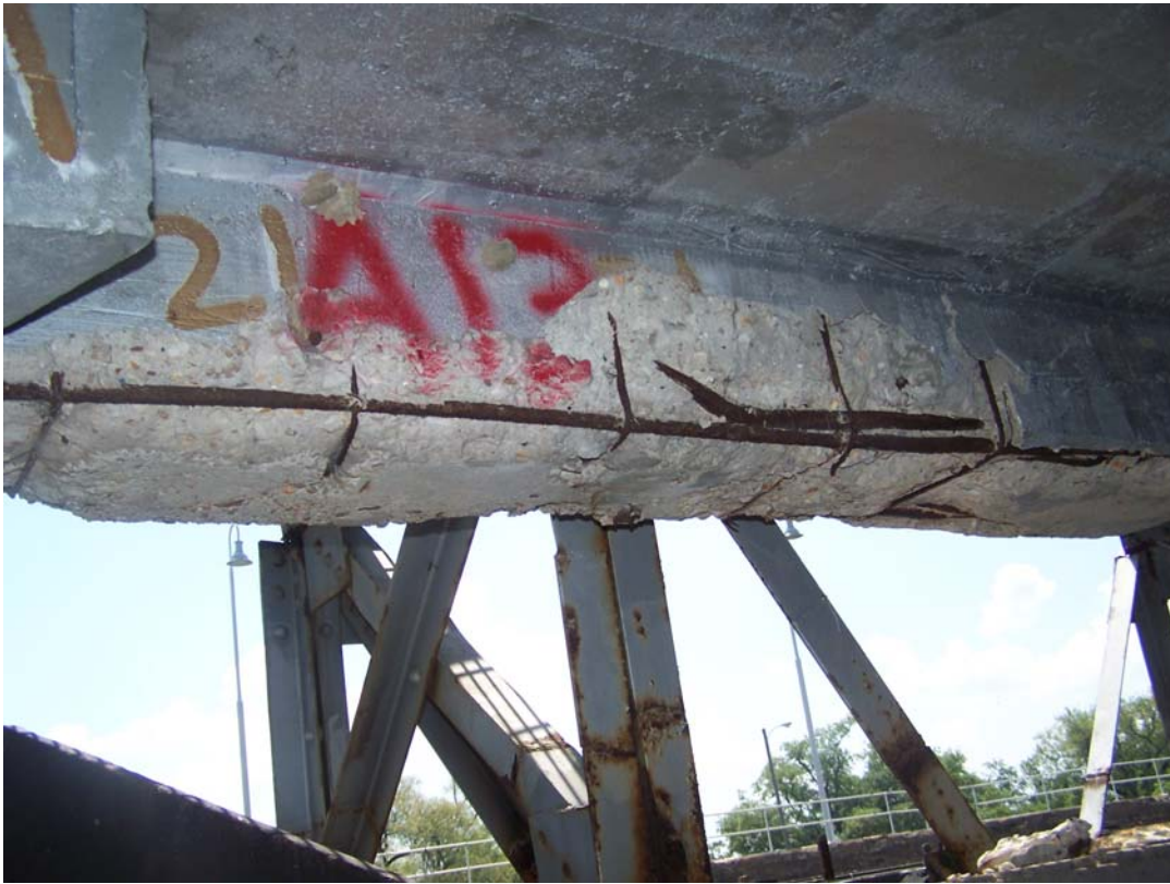
Photo 99 Spalled beam with corroded reinforcing over opening for gate 7.
