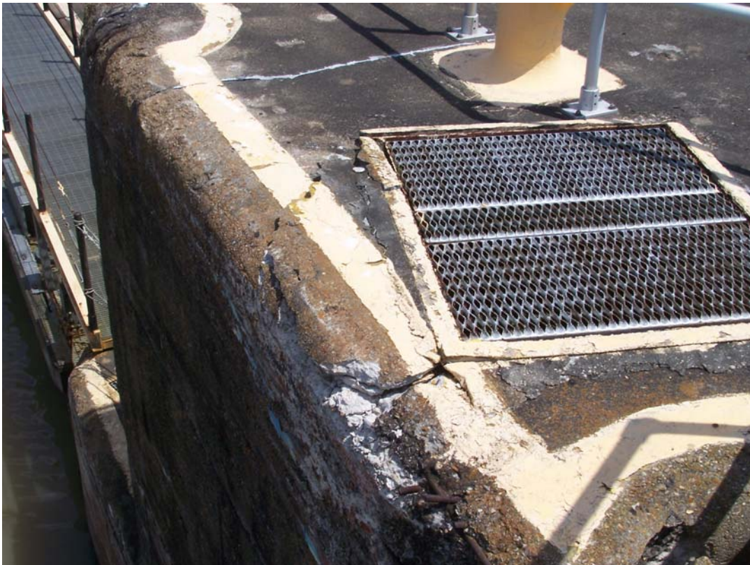
Photo 134 Spalled concrete and exposed steel in northeast gatebay.
