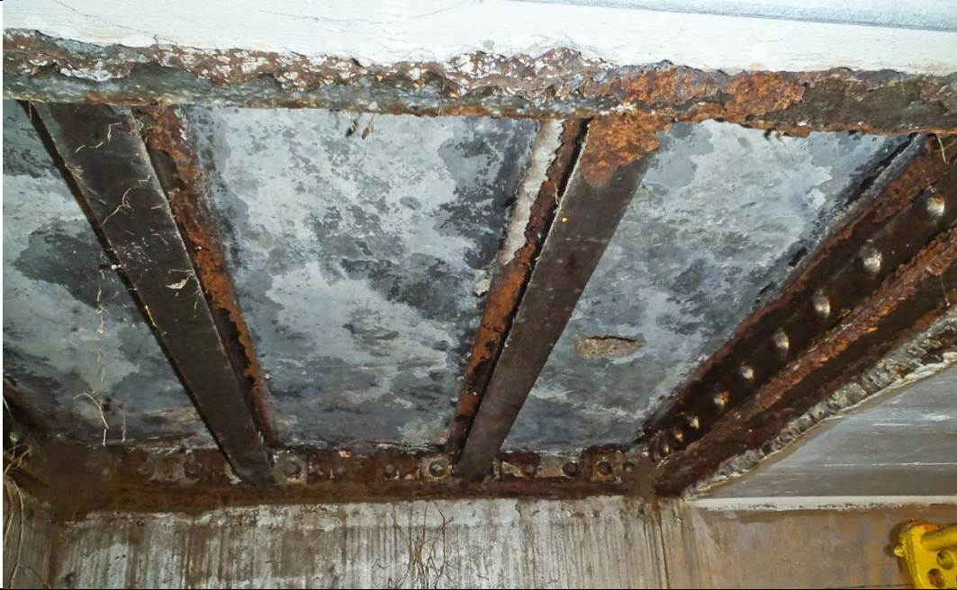
Corroding I-beams supporting hatch cover also showing section loss of beams and hatch recess steel frame. IHNC Lock Photo 04-23-2014No Structure020-1.jpg
