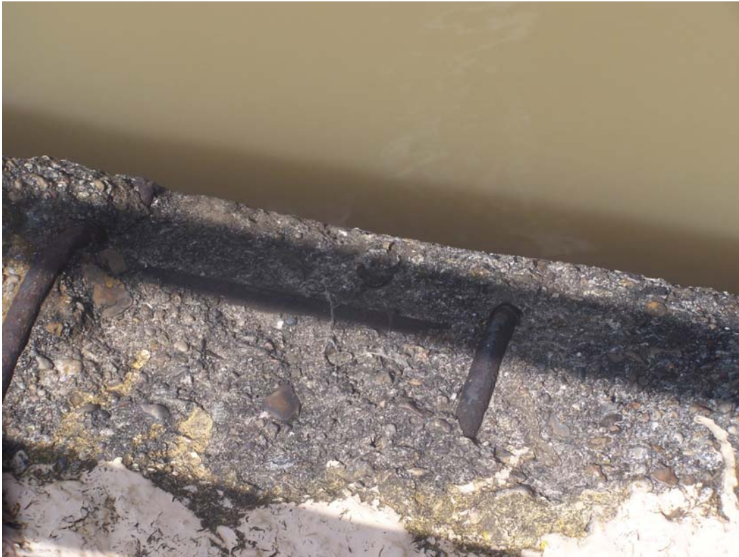
Photo 147 Spalls in east lock chamber wall. (Typical).
