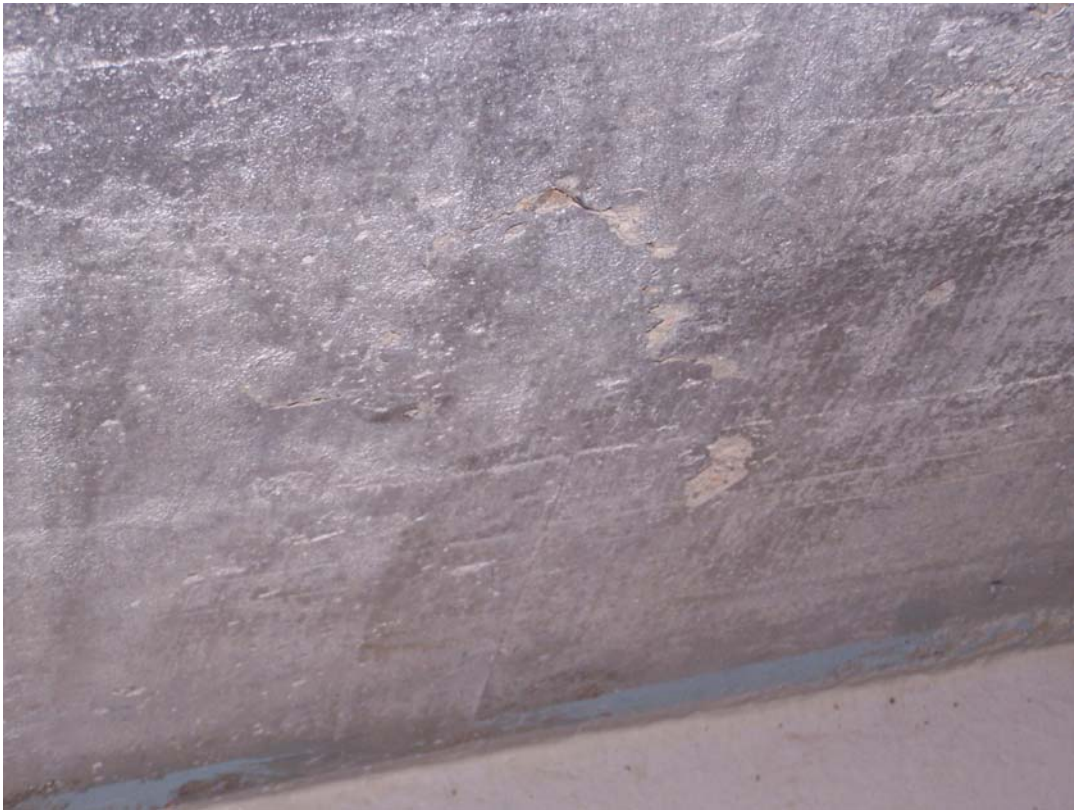
Photo 77 12" x 7" delamination in west tunnel wall.
