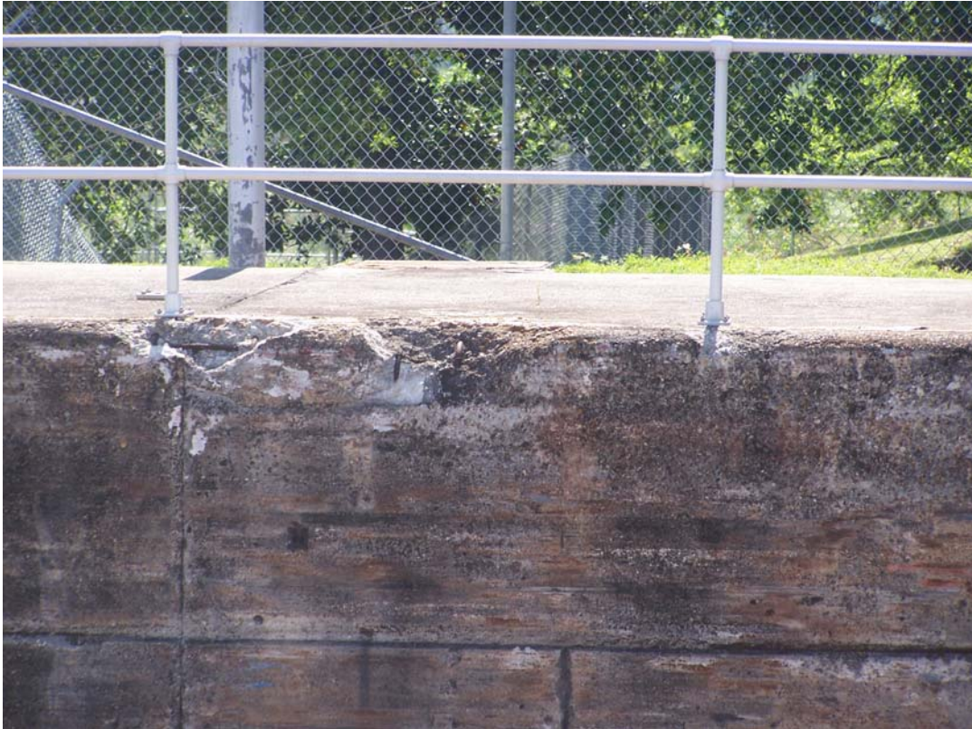
Photo 34 Spalls with exposed steel on the east wall on river side near the gate for the bridge.
