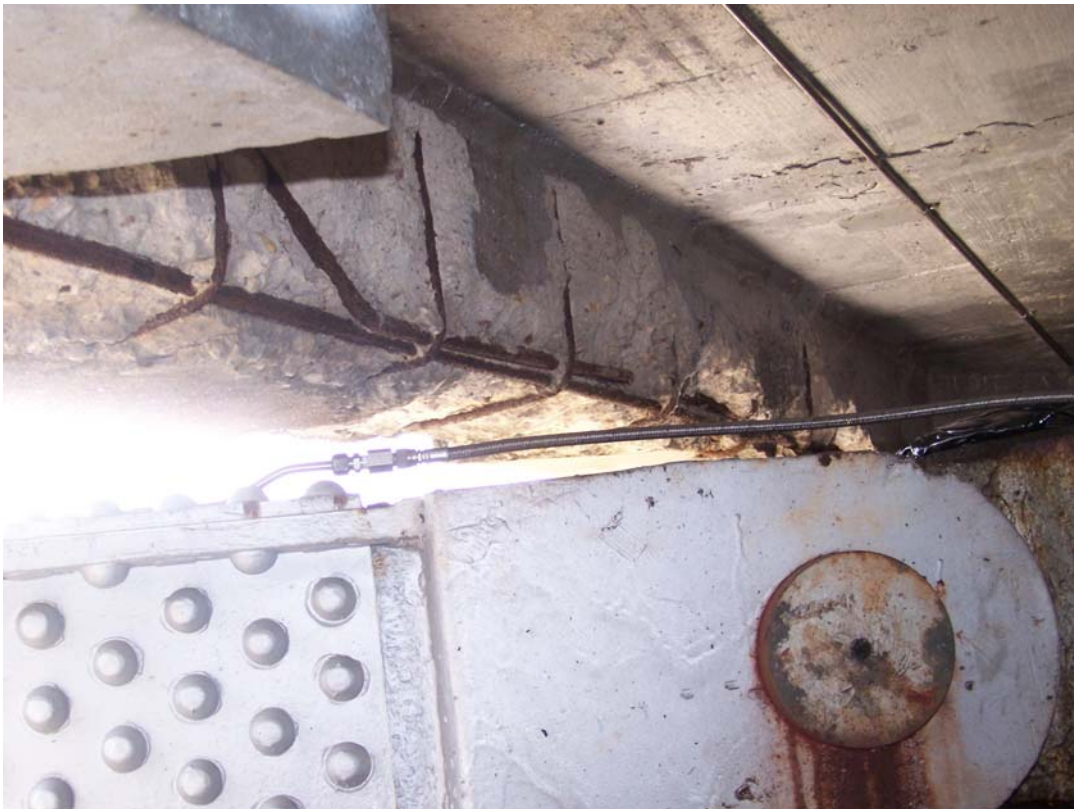
Photo 128 Deteriorated beam over opening for Gate 5.
