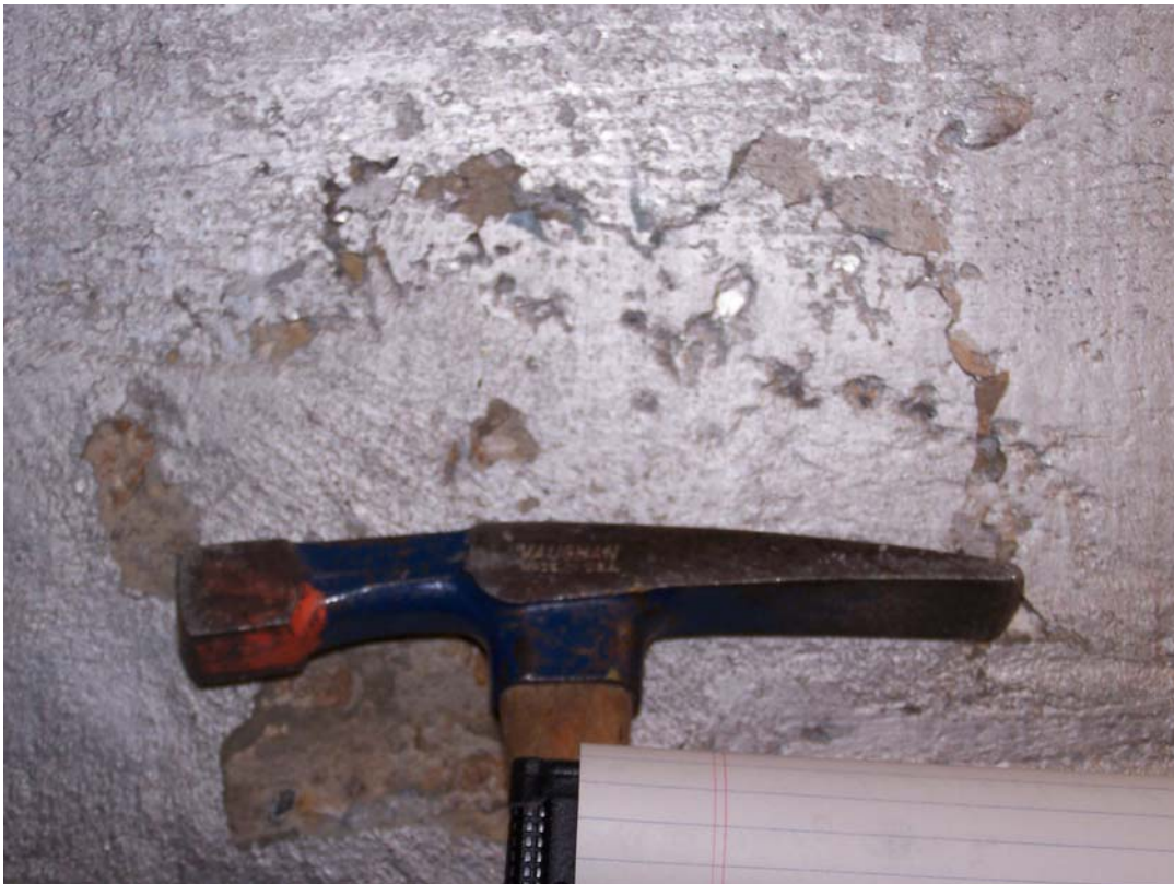
Photo 66 Small shallow delamination in the West tunnel wall.
