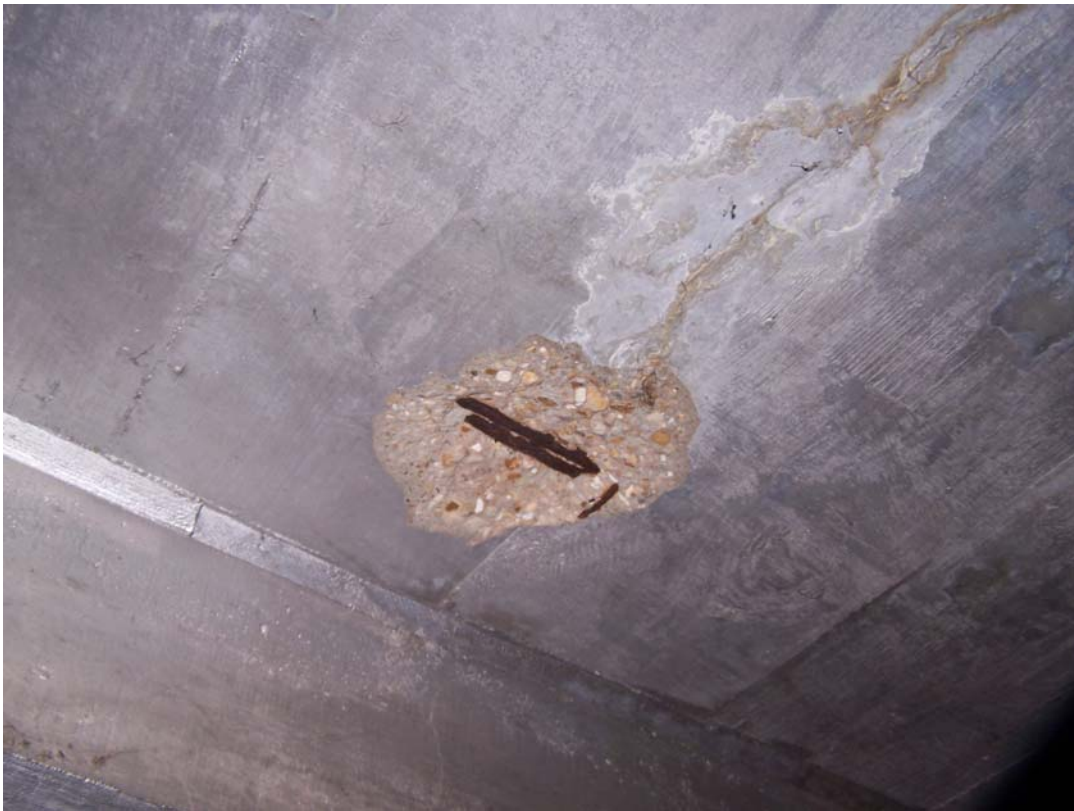
Photo 46 Popout in ceiling near valve 11 caused by corroding steel.
