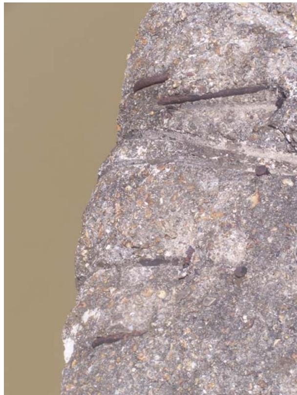
Photo 146 Spalls in north gatebay.
