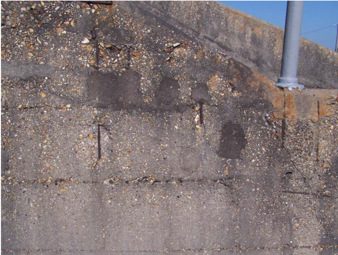
Photo 3 Spalling, cracks, and exposed steel in the wall below stairs between gates 7 and 9 on northwest side of lock.
