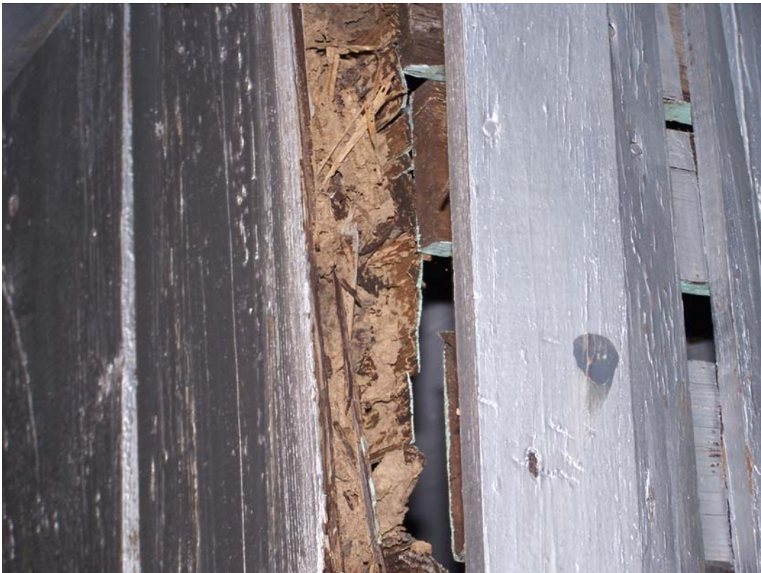
Photo 78 Termite damage in walls of storage area in room 5.
