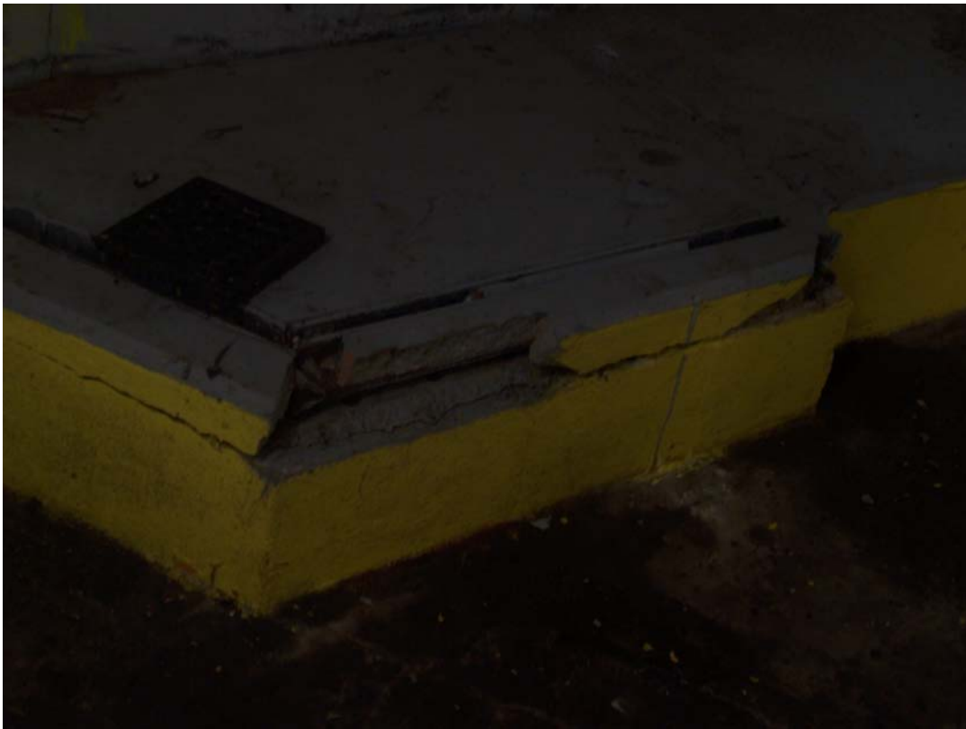
Photo 152 Spalled/delaminated concrete in Room 2. Has increased since last inspection.
