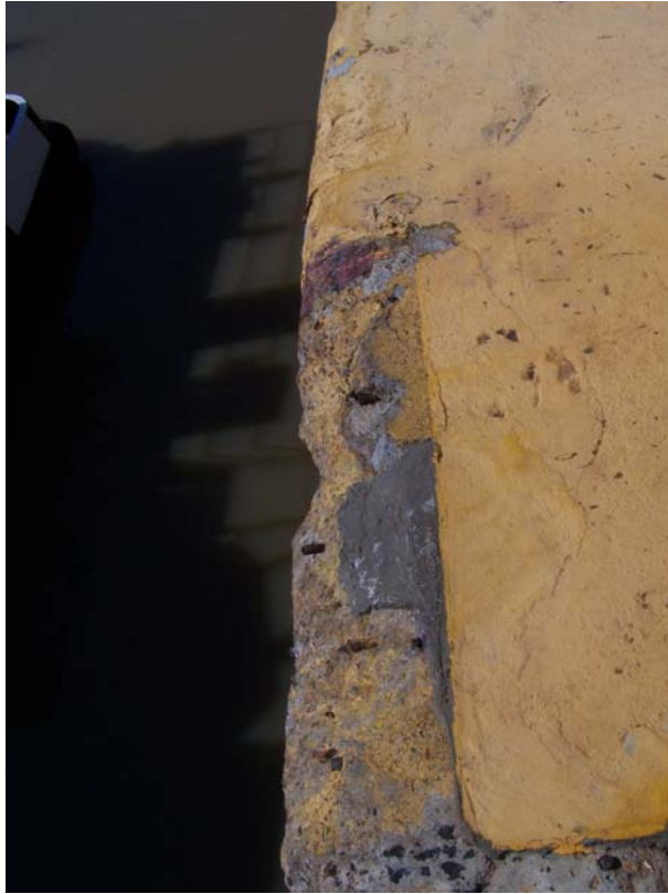
Photo 11 Spalls in top of the west chamber wall near control house.
