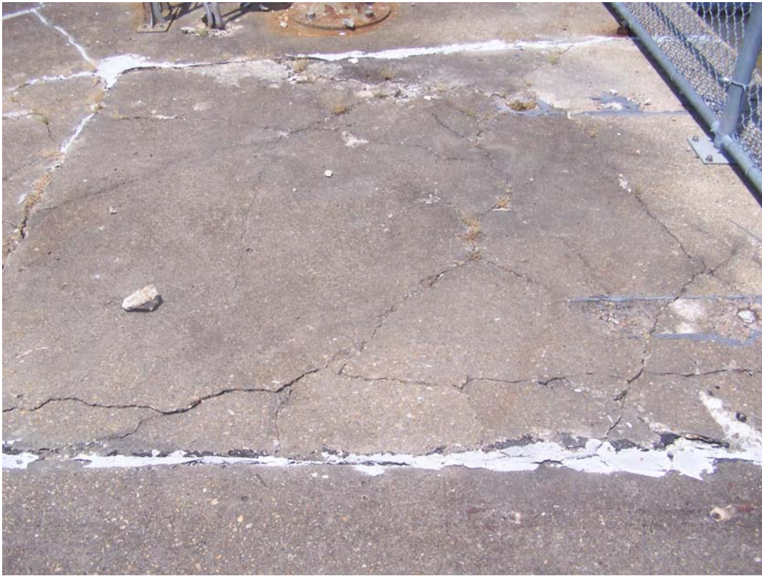
Photo 143 Large area of cracked and spalling concrete behind northeast retaining wall. The whole area sounded hollow underneath.
