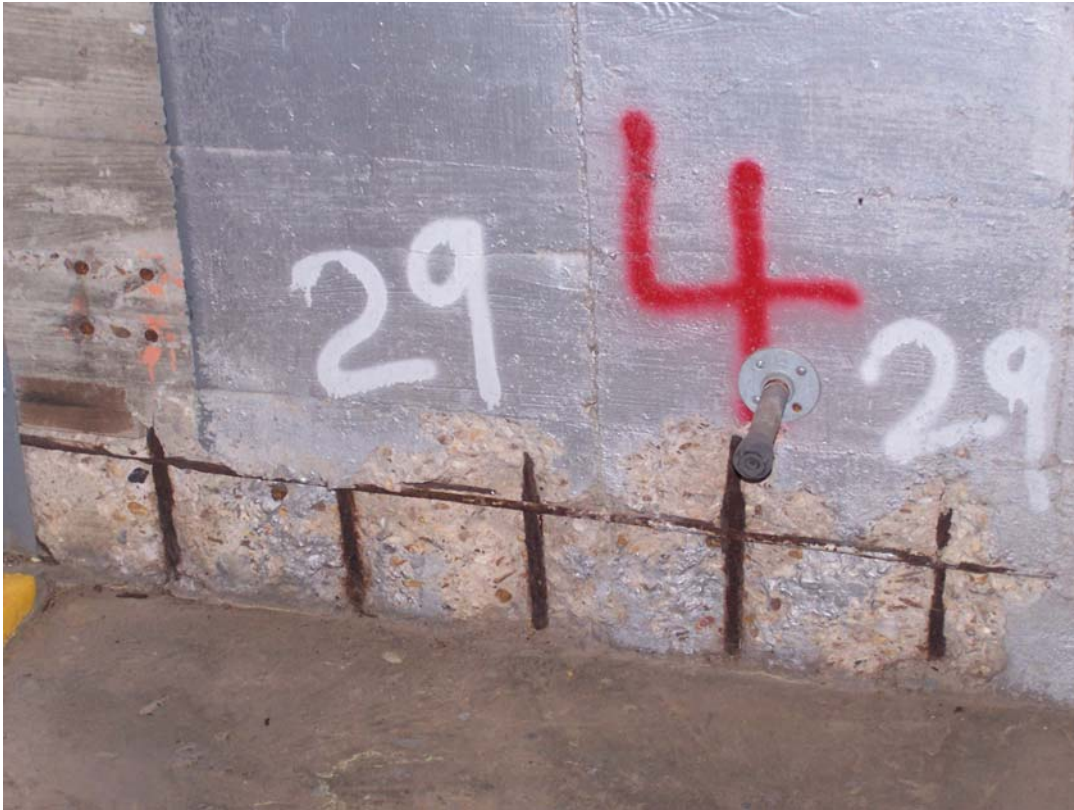
Photo 115 Popouts/spalling along the bottom of the wall near valves 15 and 16.
