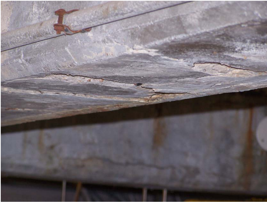
Photo 127 Spalls in beam over Gate 5 machinery. About mid span of beam.
