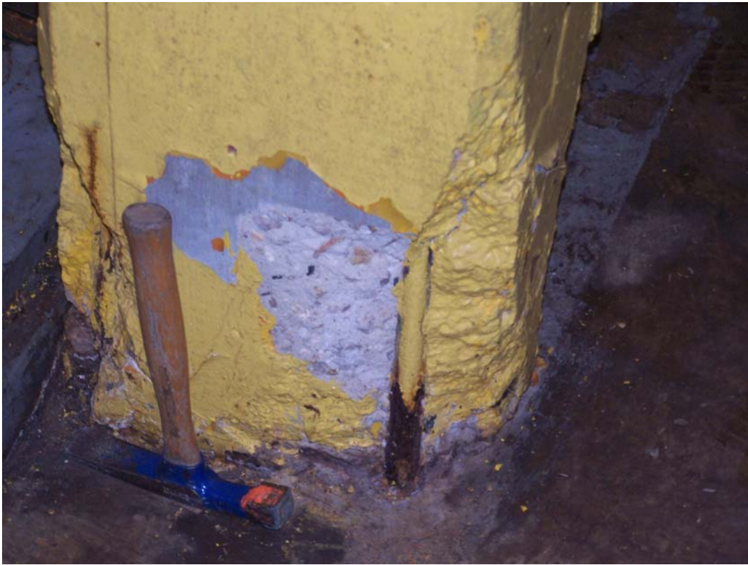
Photo 111 Spalling and corroded steel at the bottom of the column near the louvers by the hinge of gate 5. Damage to about 20" up from floor.
