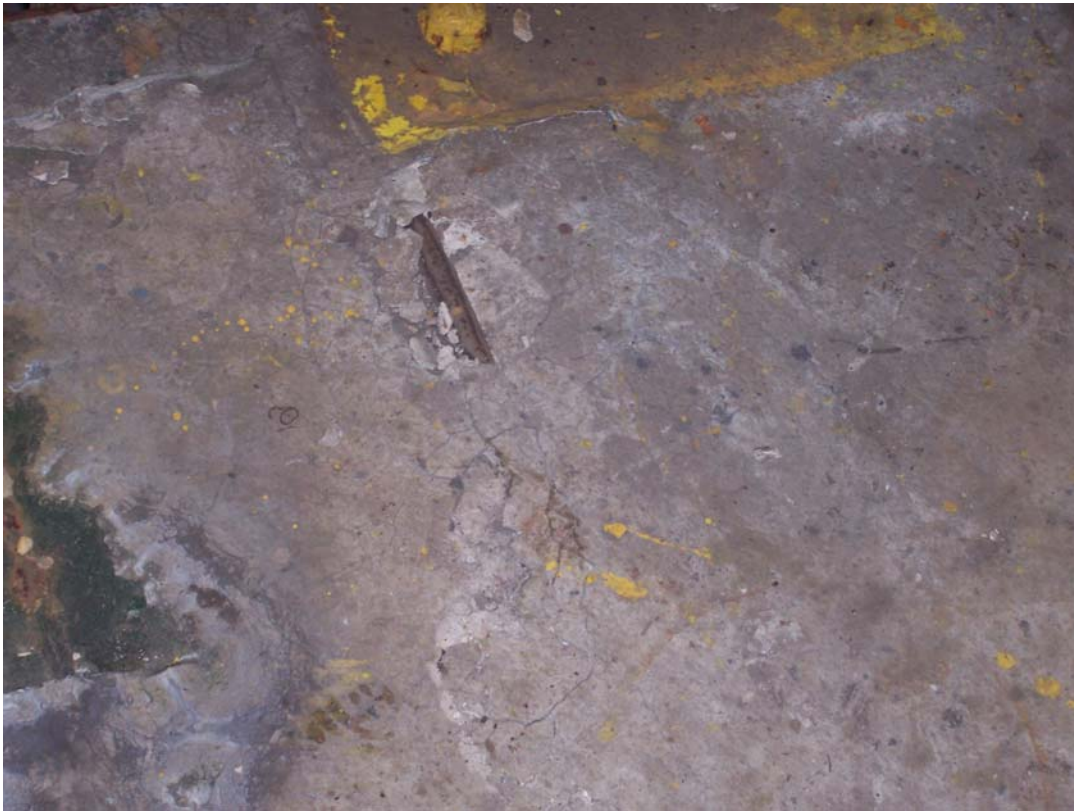
Photo 179 1' x 1' delamination in floor near valve between Rooms 6 and 8.
