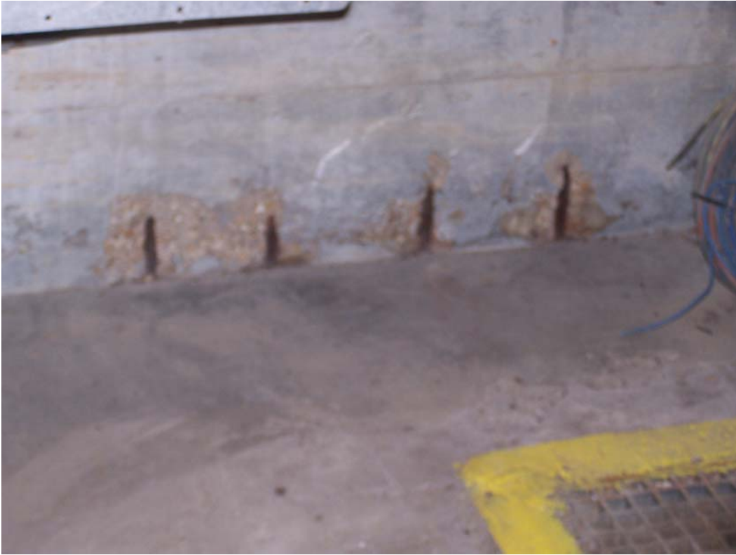
Photo 57 Spalls caused by corrosion of steel at the bottom of the wall in room 3.
