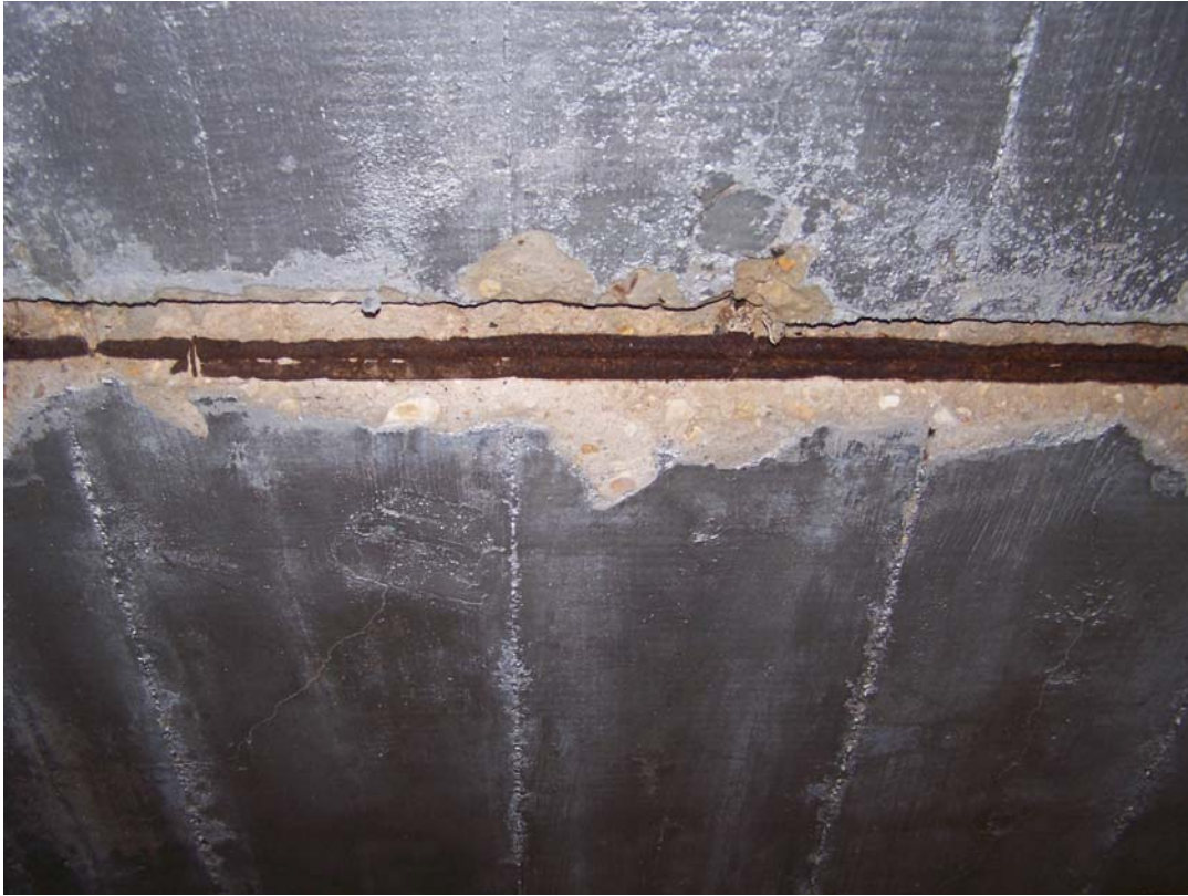
Photo 119 Spalls in ceiling near gate 5.
