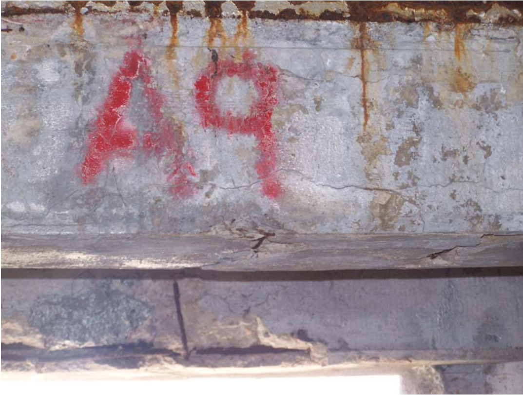
Photo 125 Cracks and spalls in beam over Gate 5 machinery.
