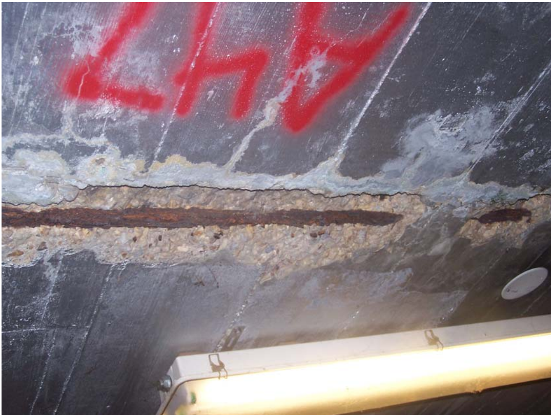
Photo 180 Spalls with corroded steel in ceiling between Rooms 6 and 8.
