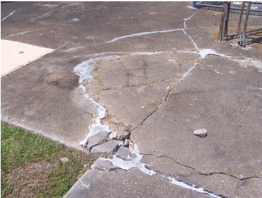
Photo 144 Large area of cracked and spalling concrete. The whole area sounded hollow underneath
