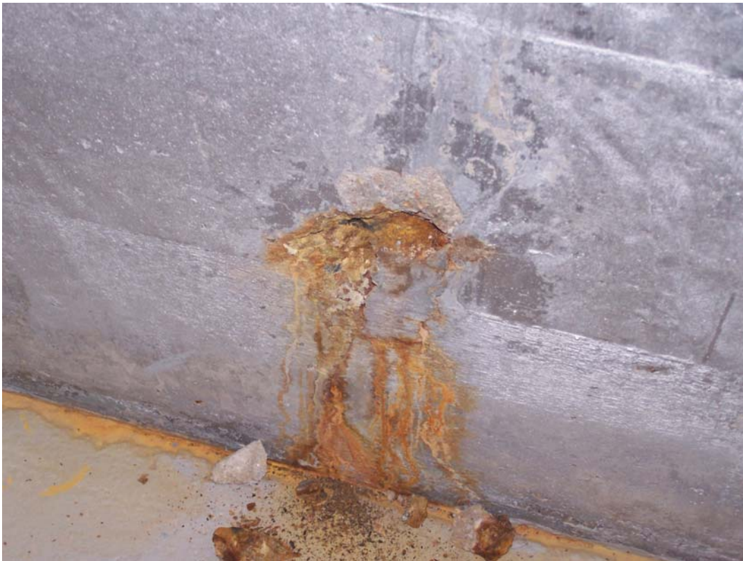
Photo 72 Popout in the bottom of west tunnel wall.
