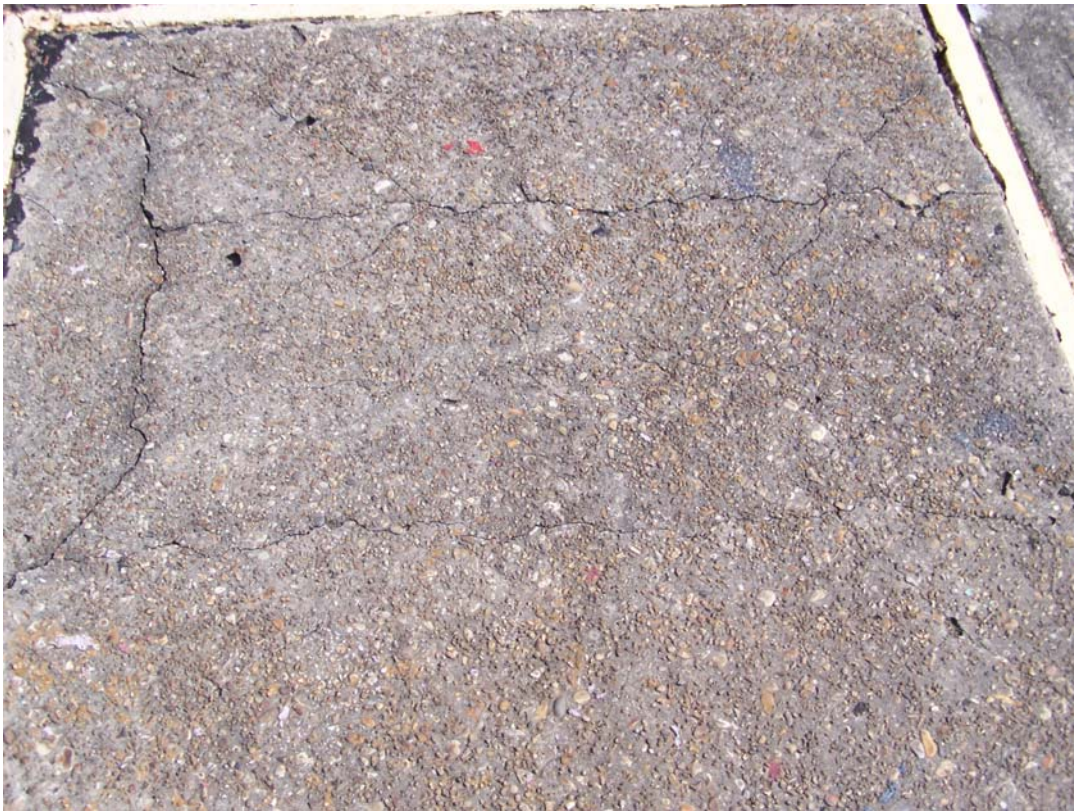
Photo 24 Hatch cover behind the west chamber wall near reference marker 8W.
