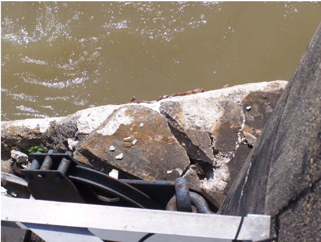
Photo 6 Large spalls and cracked concrete with exposed steel on the northwest side near hinge for gate 9.
