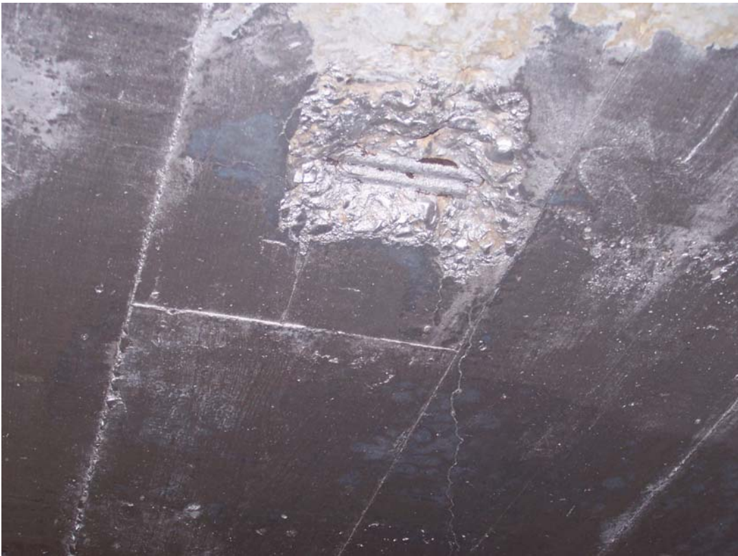
Photo 172 Painted spall in ceiling of room 6.
