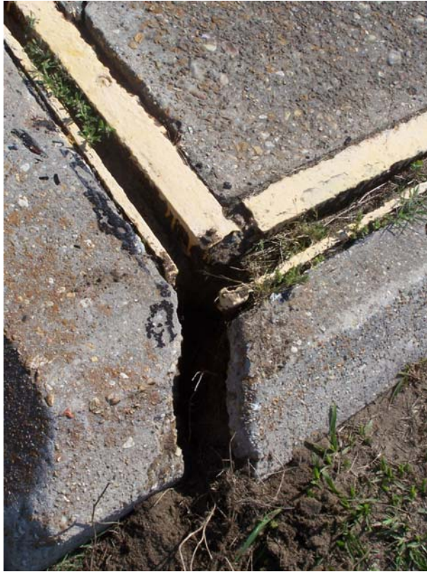
Photo 25 Hatch cover behind the west chamber wall near reference marker 8W.
