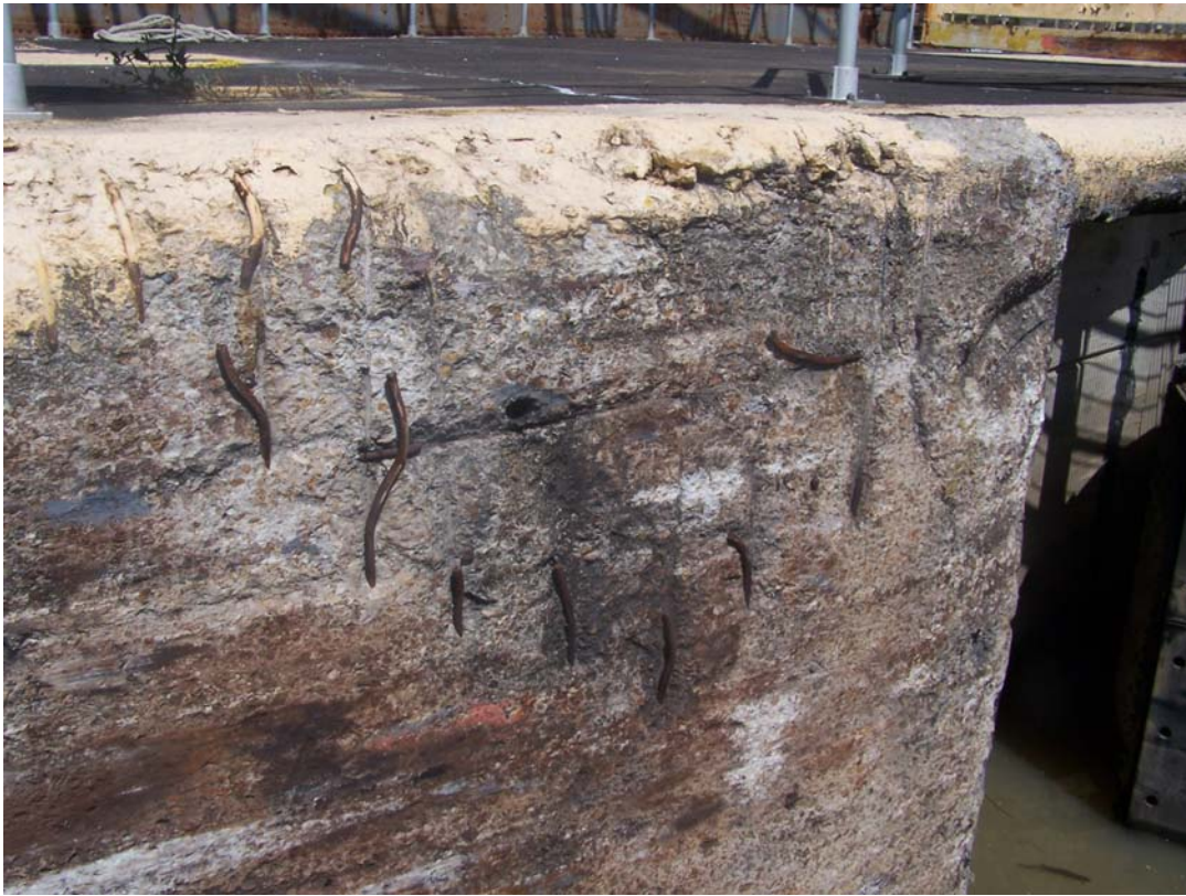
Photo 201 Spalls and exposed steel in chamber walls.
