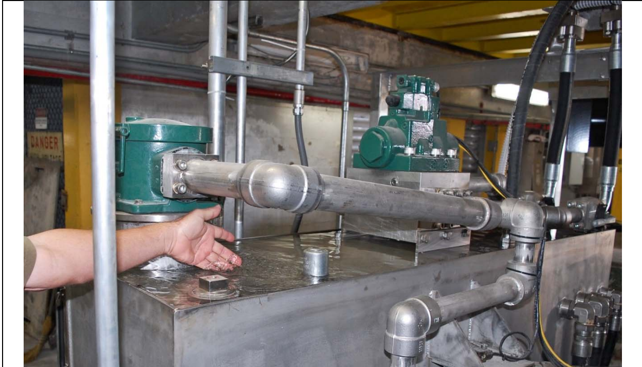
Leaking water collecting in oil retention basin. IHNC 09 Sep 16 Dewater Machinery New Flooded-2-4.jpg
