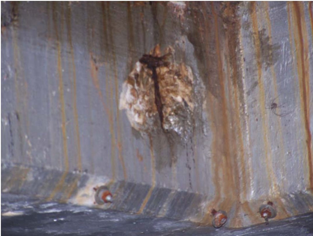
Photo 53 Popout in beam over valve 12 caused by corroding steel.
