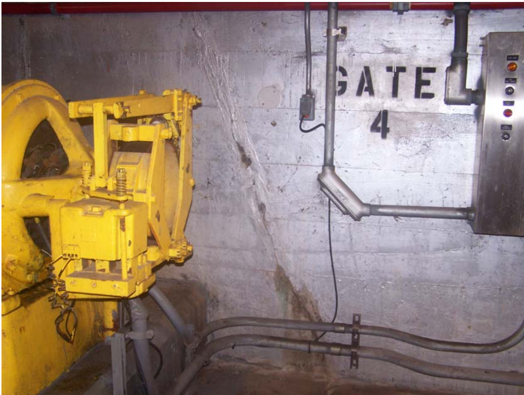
Photo 164 Diagonal crack in wall near Gate 4.
