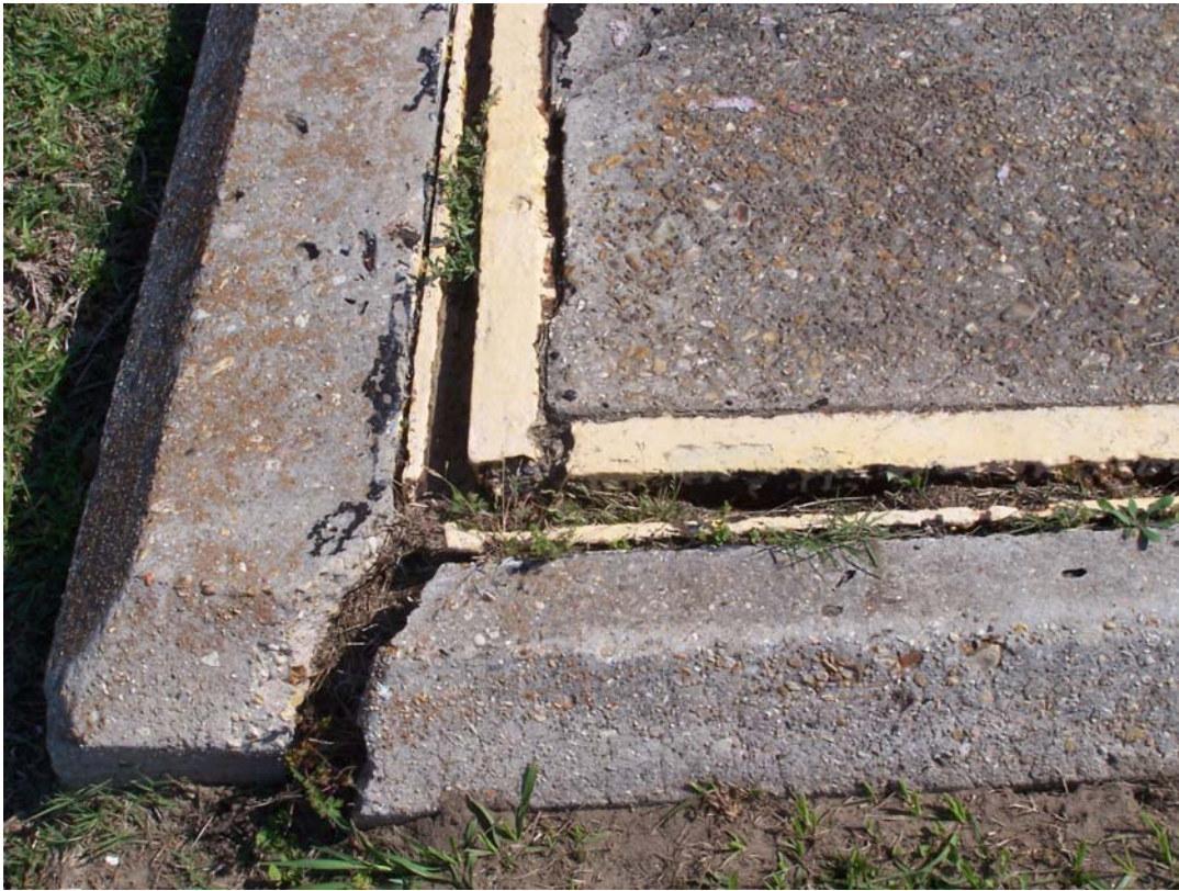
Photo 23 Hatch cover behind the west chamber wall near reference marker 8W.
