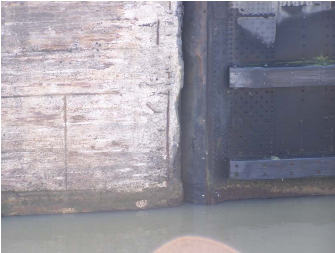
Photo 9 Spalling with exposed steel in the northeast gatebay near the hinge
