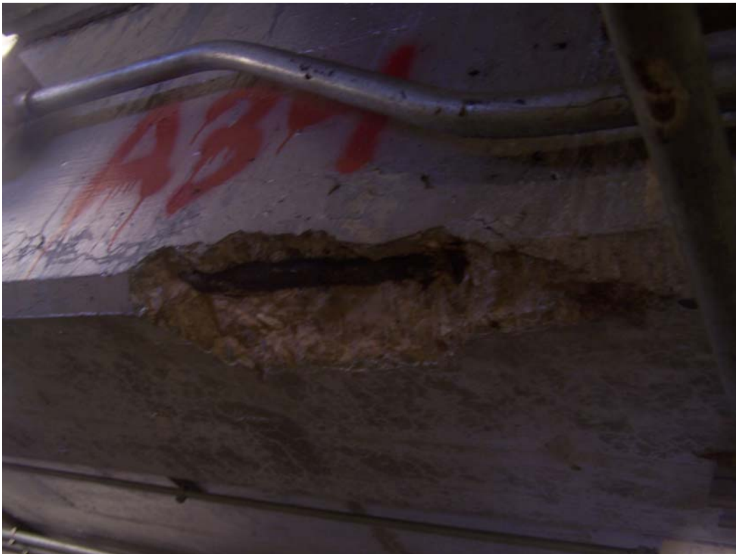
Photo 154 Spall with corroded steel in beam in Room 2.
