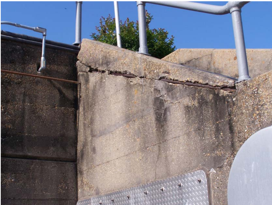
Photo 4 Spalling and exposed steel in the wall below stairs between gates 7 and 9 on northwest side of lock.
