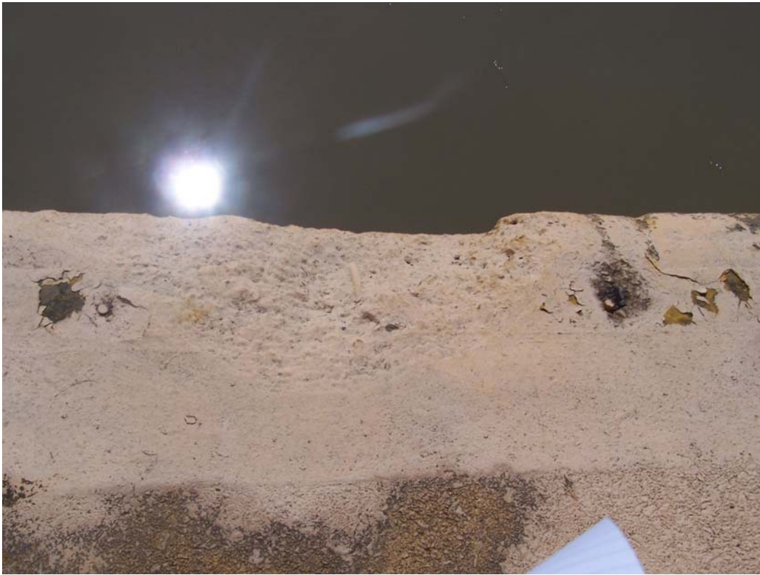
Photo 27 Spall in top of west wall near the hinge for the river side gate.
