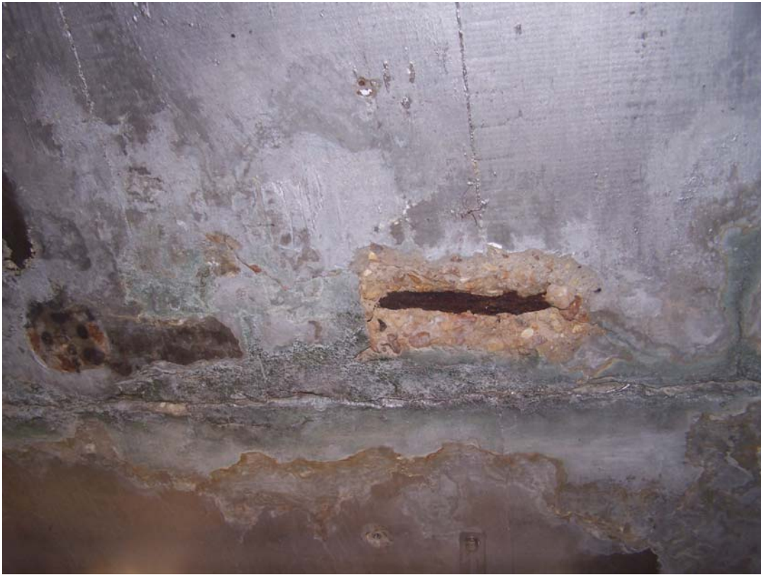
Photo 43 Popout in ceiling near valve 11 caused by corroding steel.
