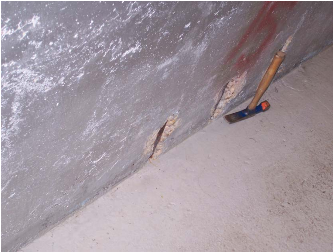
Photo 73 Popout in the bottom of west tunnel wall.
