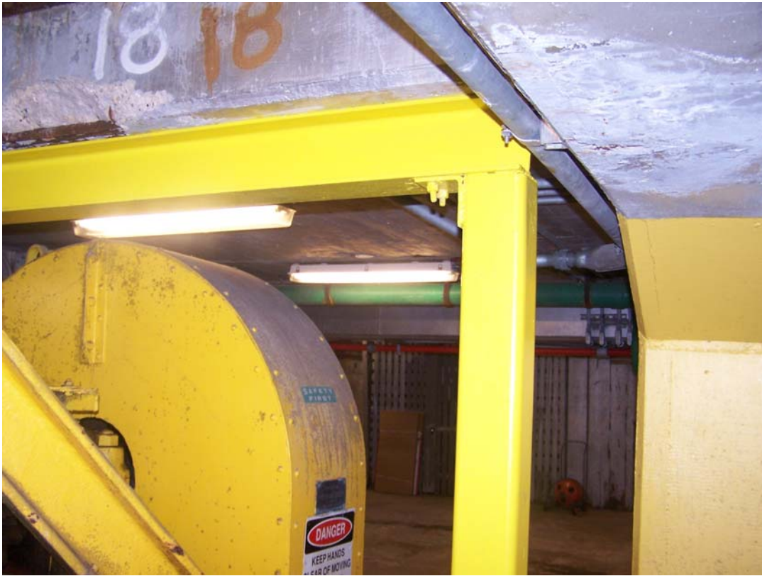
Photo 95 Spalls and corroded steel in beams over machinery in room 5. Note steel beam and columns added to support these beams.
