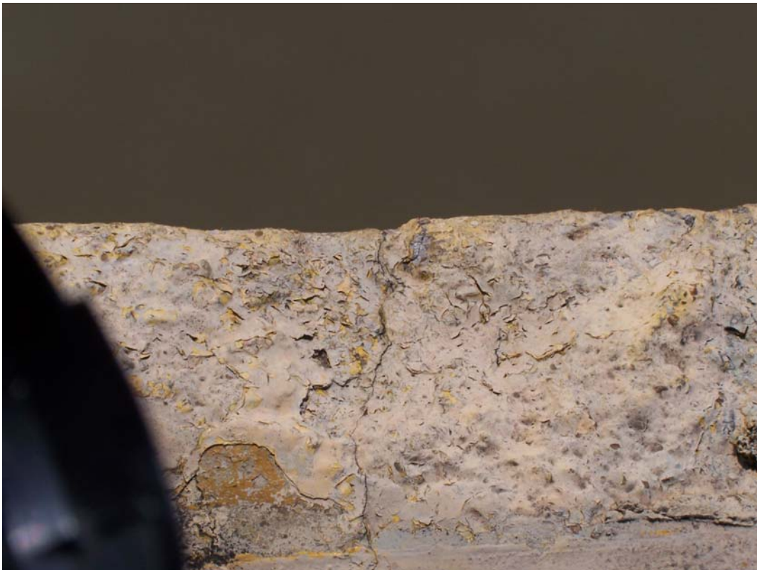
Photo 16 Spall in top of west chamber wall near light pole number 9.
