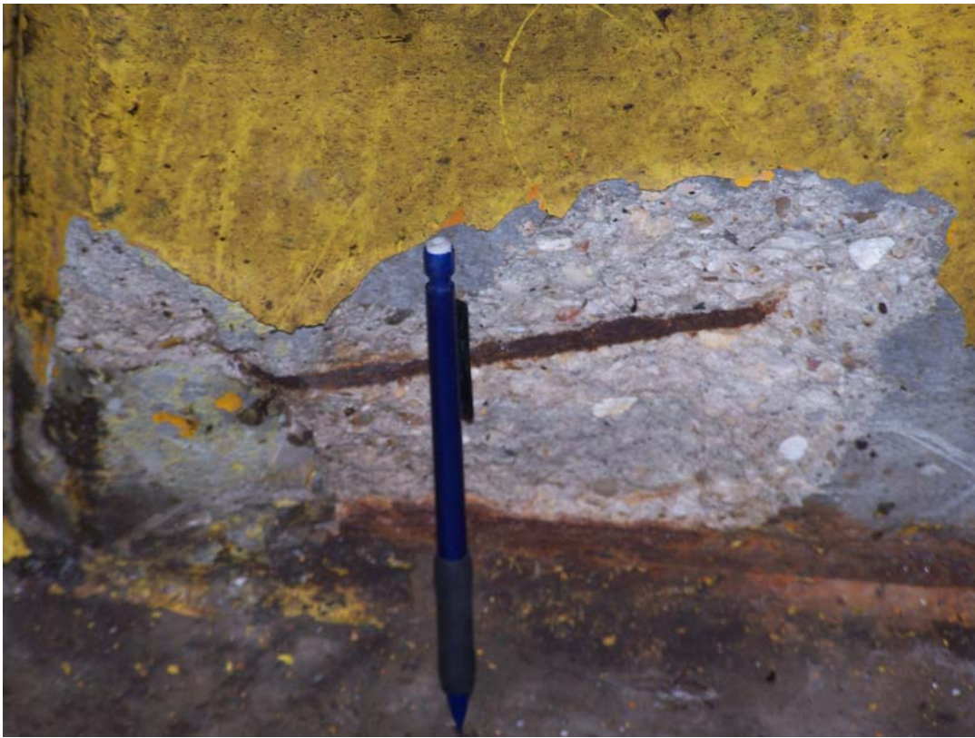
Photo 50 Spalls and delaminations at bottom of columns on both sides of hinge for gate 1.
