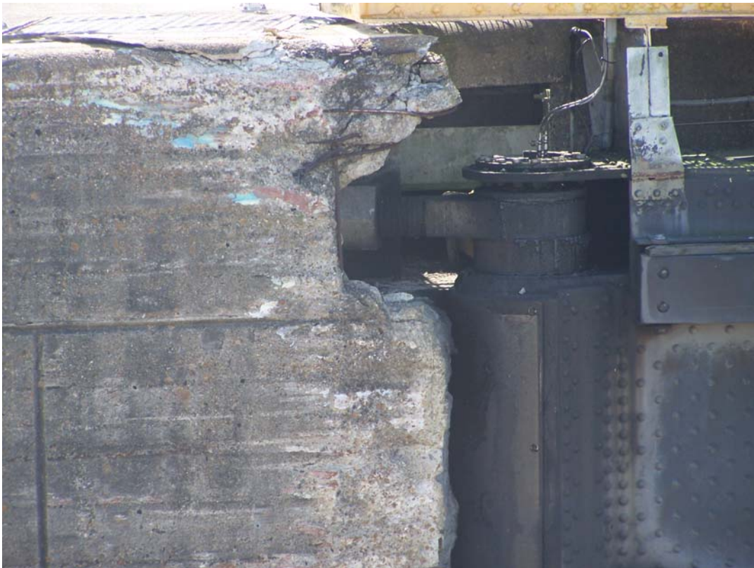
Photo 10 Spalling with exposed steel in the northeast gatebay near the hinge
