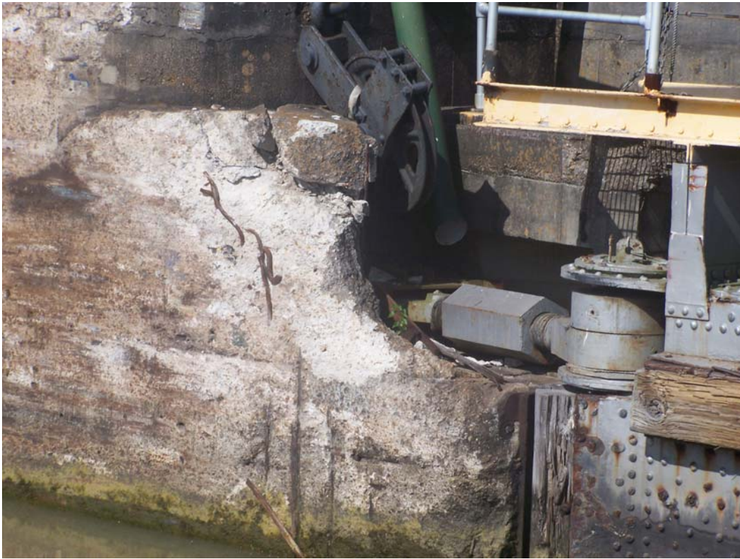
Photo 187 Damaged concrete at the northwest reverse head gate hinge.
