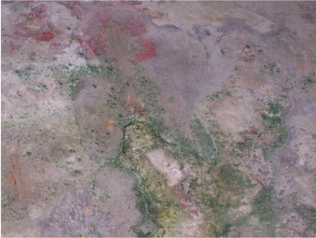
Photo 85 Failed patch in the floor of room 5.
