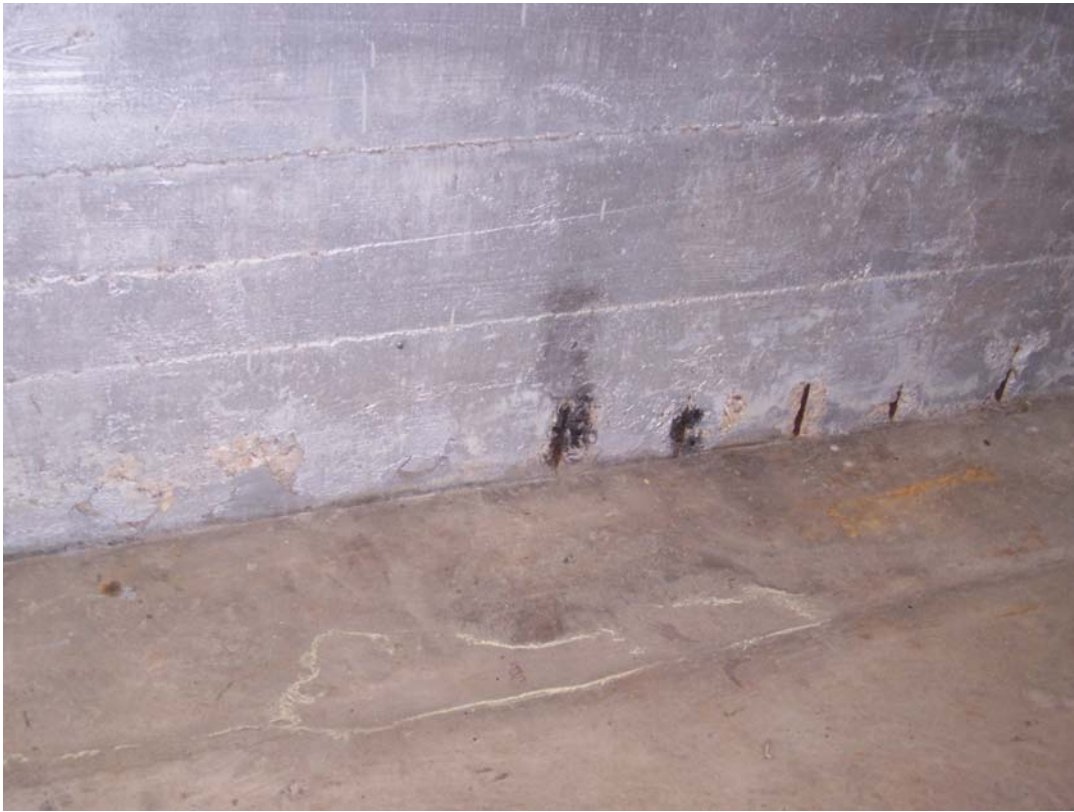
Photo 117 Popouts along the bottom of the wall near valves 15 and 16.
