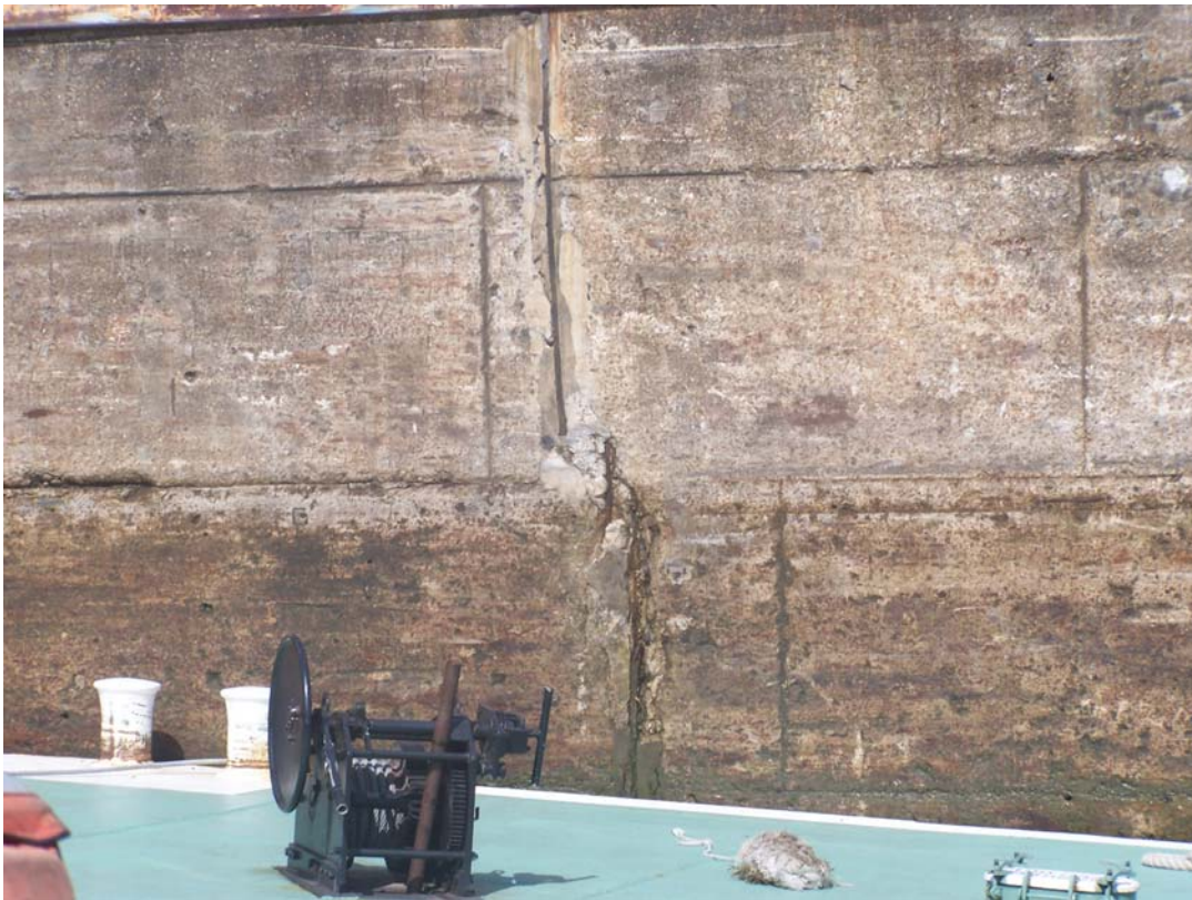
Photo 190 Spalls with exposed steel in the west chamber wall on river side.
