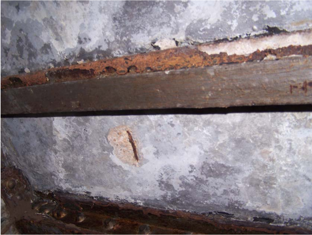
Photo 69 Bottom of hatch cover in west tunnel.
