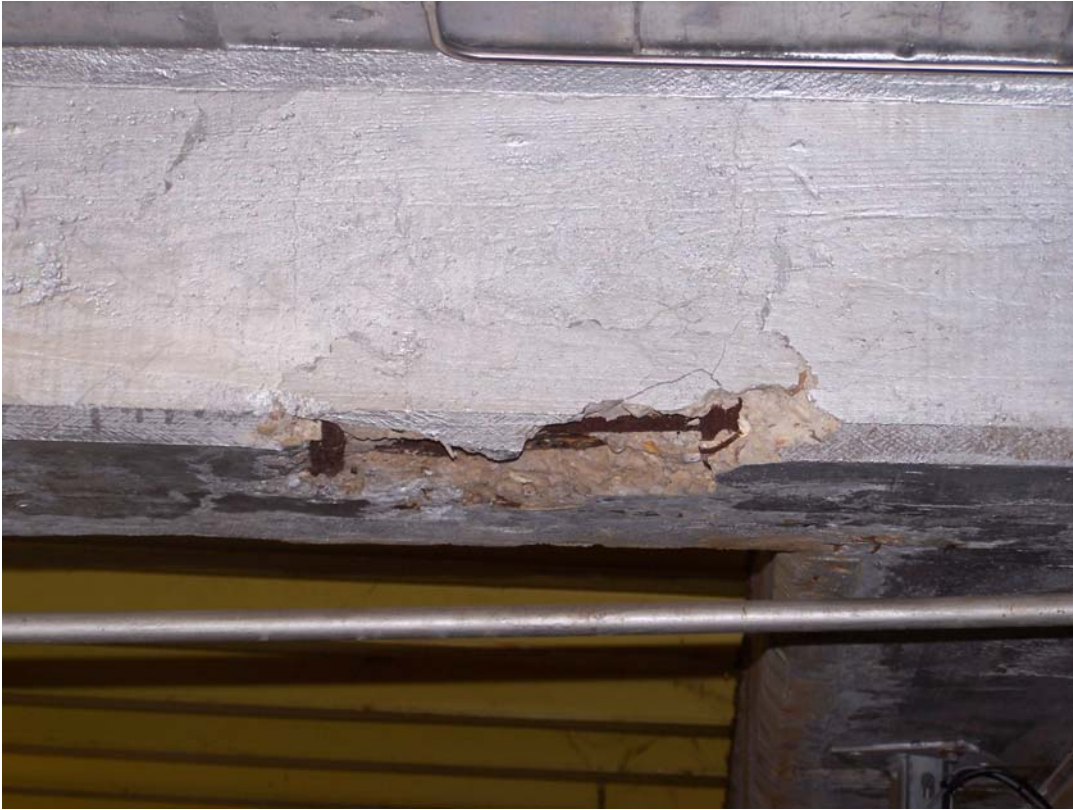
Photo 121 Spall and corroded steel in beam over gate 5 machinery.
