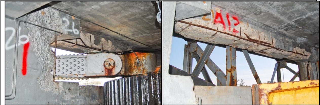
Pictured are main gate and reverse head gate strut arm openings on NW side of chamber that support the edge of the lock wall deck. These two pictures are typical for all eight machinery room/strut arm openings and show severe spalling exposing the rebar support system.
