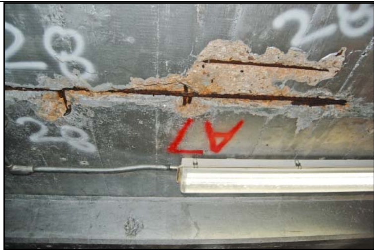
Underside of concrete deck in a machinery room in the west wall.
