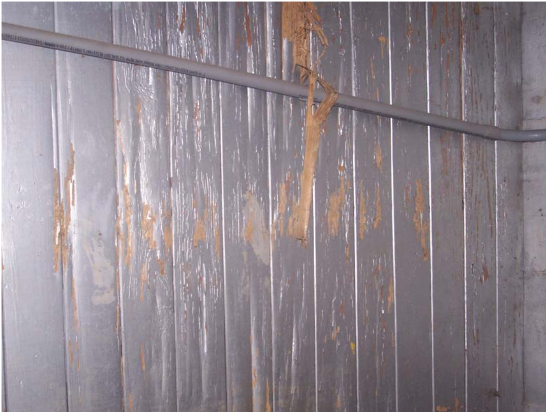
Photo 165 Termite damage in walls of storage area in Room 2.
