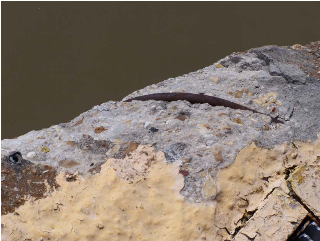
Photo 8 Spalls in the northeast corner of the northwest gatebay. Appears to be new.
