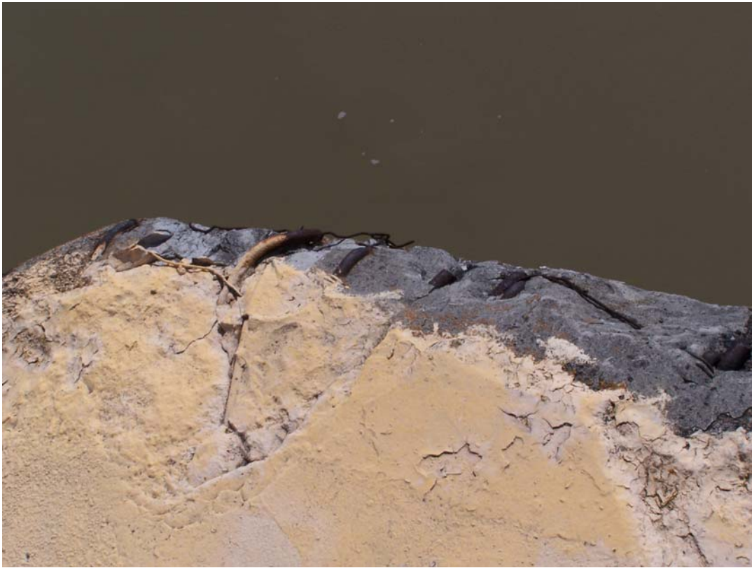
Photo 7 Spalls in the northeast corner of the northwest gatebay
