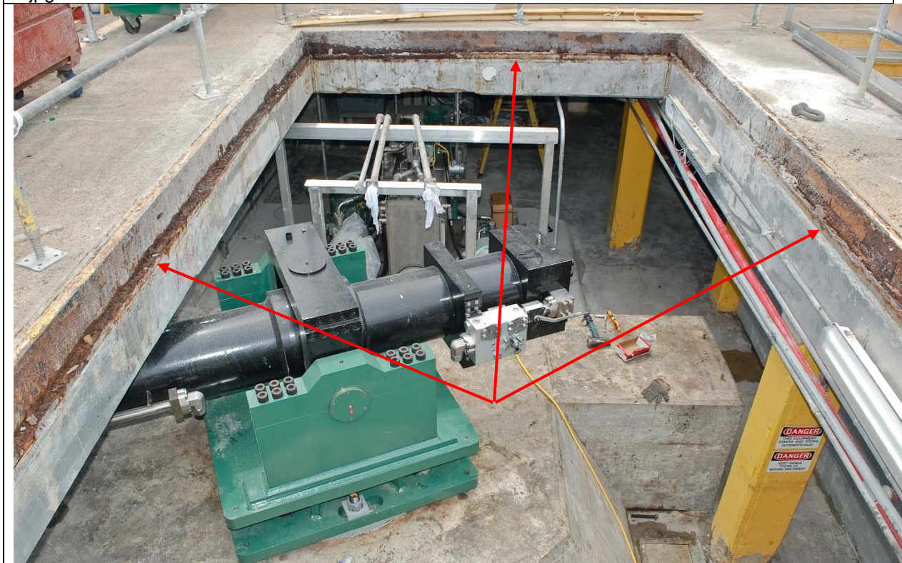
Machinery opening showing steel frame with rusted out water diverting lip gone from the opening recess. IHNC 24 Aug 16 Dewater Gate 7 Cylinder New-7-7.jpg
