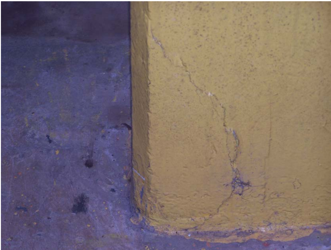
Photo 90 Corner of column in Room 5.
