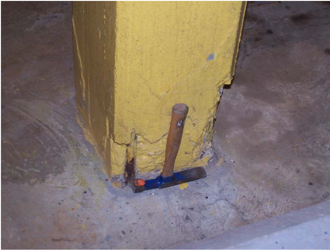
Photo 89 Spall at the bottom of column in Room 5. Delamination continues about 19” up.
