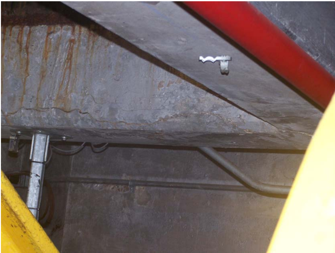
Photo 162 Crack in beam over Gate 4.
