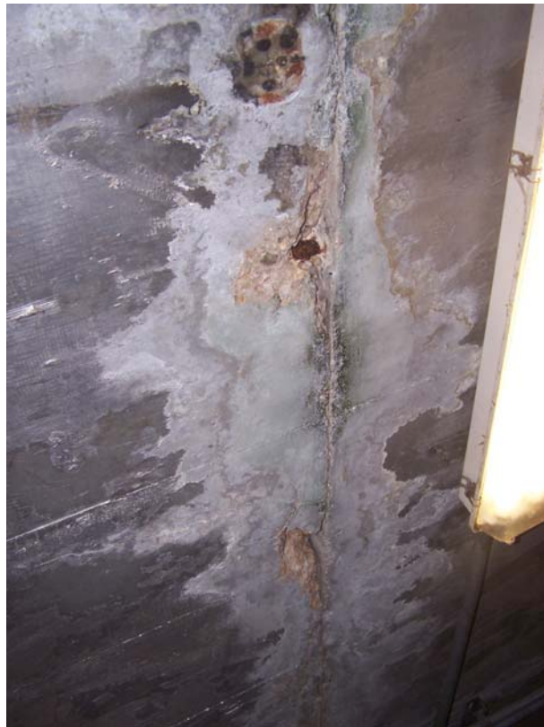
Photo 44 Spalls in ceiling near valve 11 caused by corroding steel
