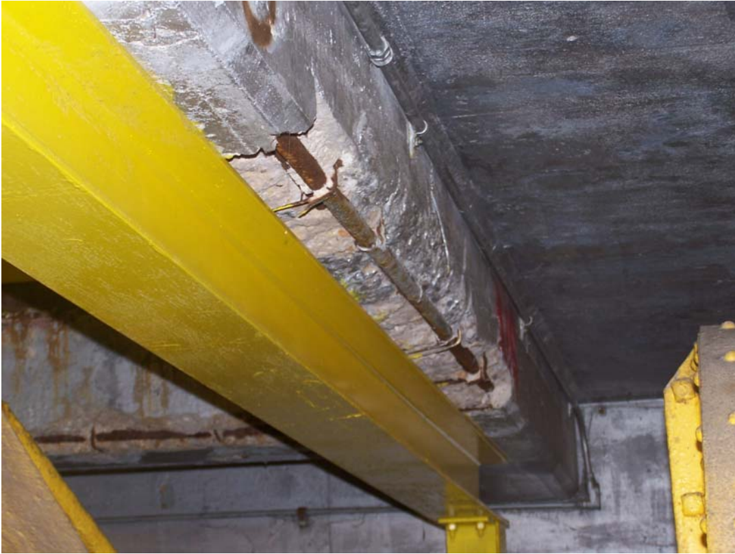
Photo 93 Spalls and corroded steel in beams over machinery in room 5. Note steel beam and columns added to support these beams.
