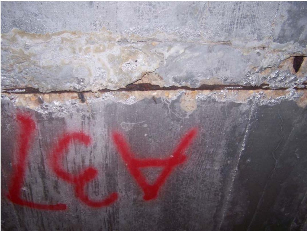
Photo 156 Spalls and popouts with corroded steel in ceiling of Room 2.
