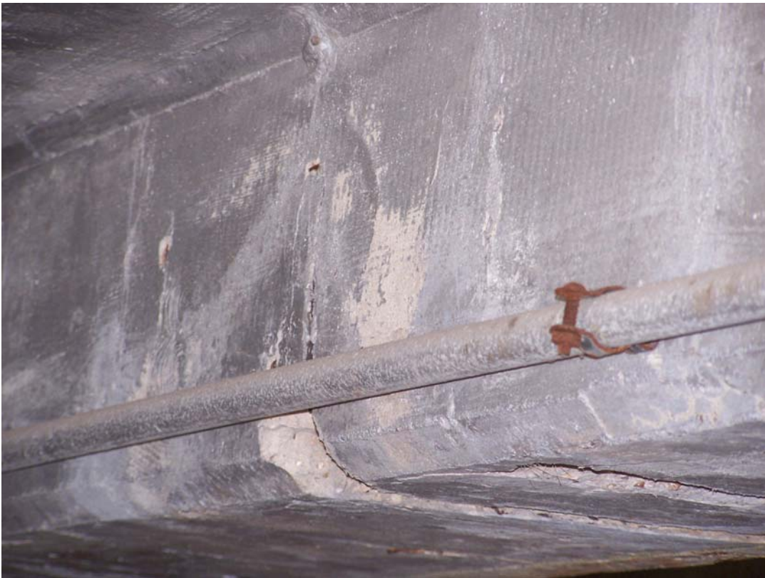
Photo 126 Spalls in beam over Gate 5 machinery. About mid span of beam.
