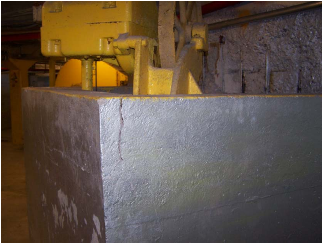
Photo 83 Cracks in top of wall around sump pump in room 5.
