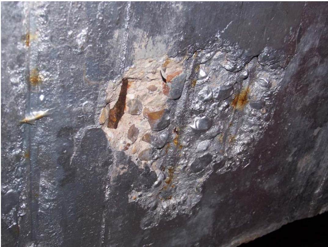
Photo 42 Popout in beam near valve 11 caused by corroding steel.
