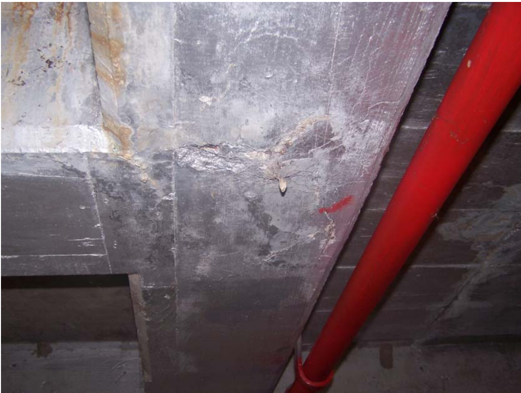
Photo 176 Cracks in beams by hinge in Room 6.
