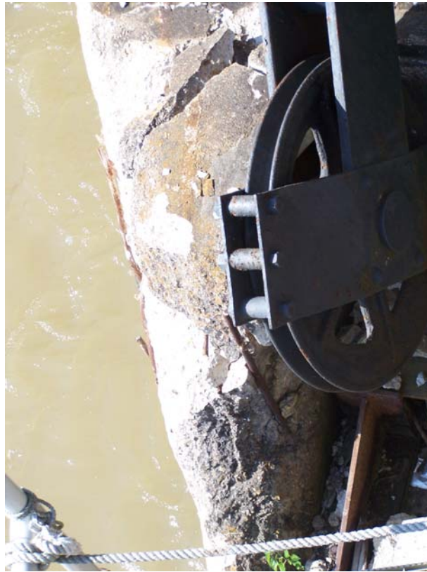
Photo 5 Large spalls and cracked concrete with exposed steel on the northwest side near hinge for gate 9.
