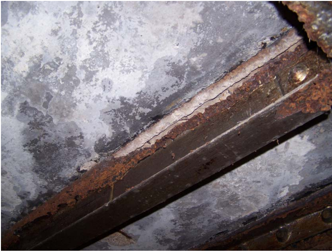
Photo 71 Bottom of hatch cover in west tunnel.
