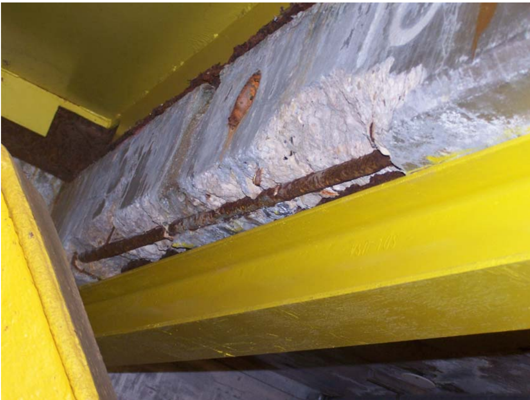
Photo 94 Spalls and corroded steel in beams over machinery in room 5. Note steel beam and columns added to support these beams.
