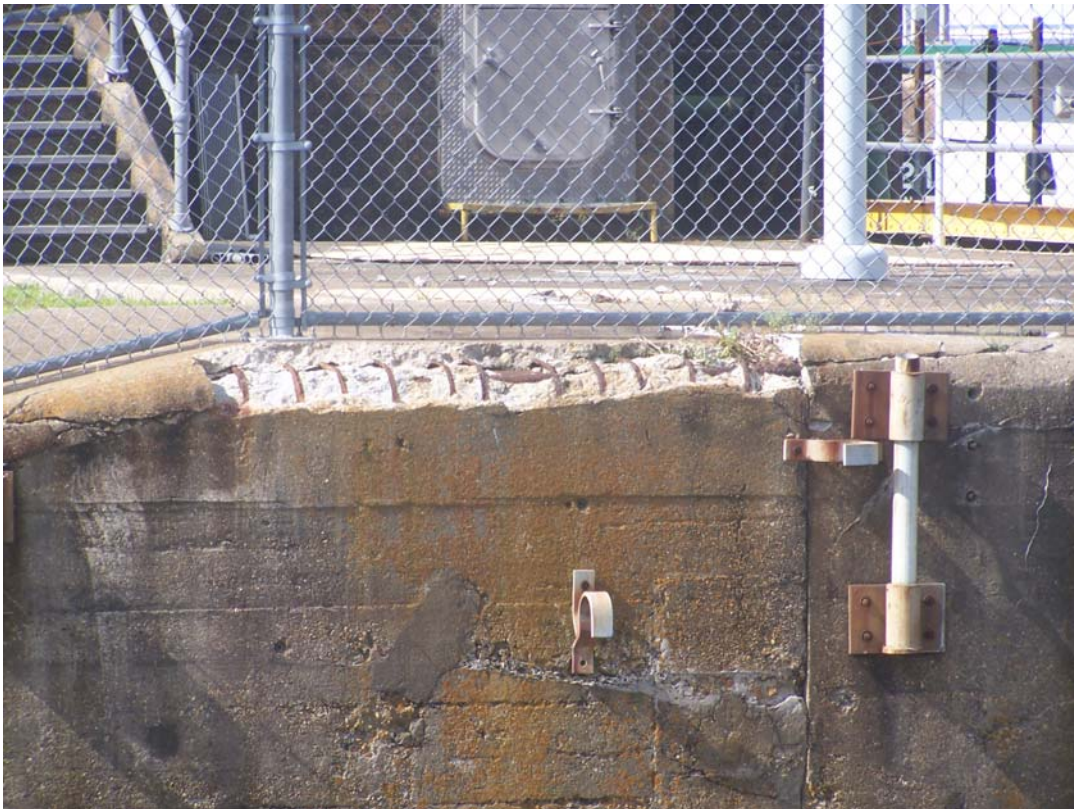
Photo 184 Cracks and spalling in the retaining wall on the northeast side.
