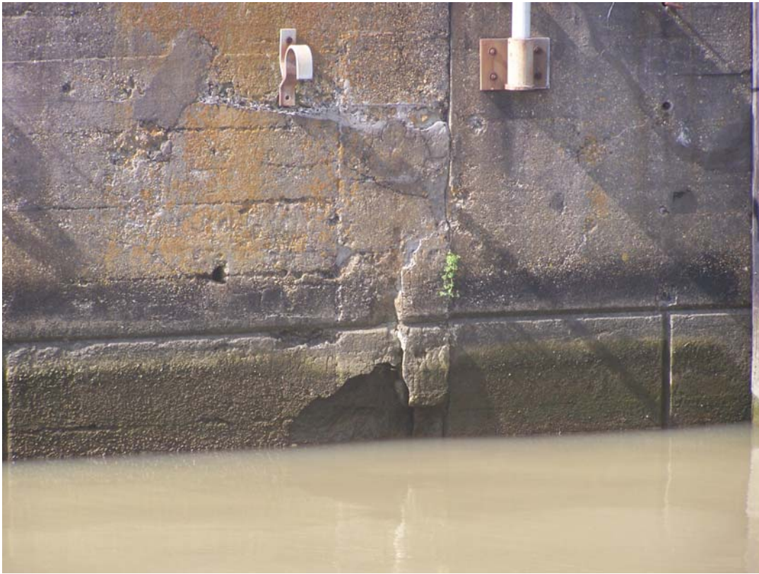
Photo 183 Cracks and spalling in the retaining wall on the northeast side.
