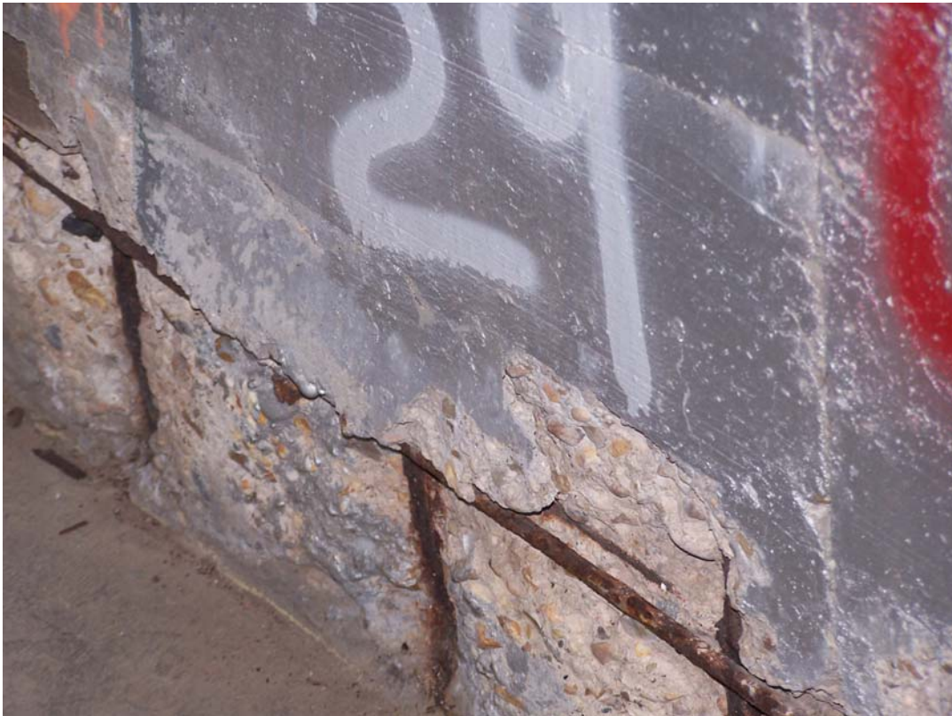
Photo 116 Popouts/spalling along the bottom of the wall near valves 15 and 16.
