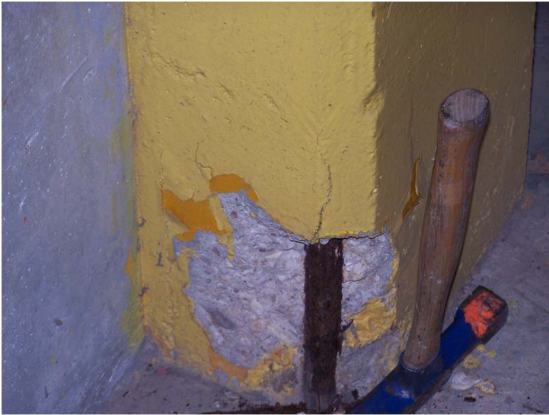
Photo 105 Bottom of column in the wall in room 5. Delamination continues up the column.
