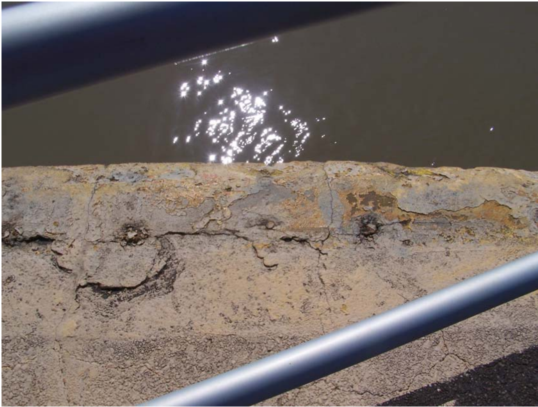
Photo 21 Delamination (2'x1') along edge of west chamber wall.
