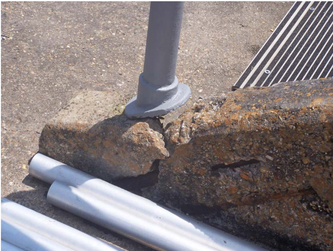
Photo 142 Spall where handrail post embeds in stairway wall. Handrail is loose
