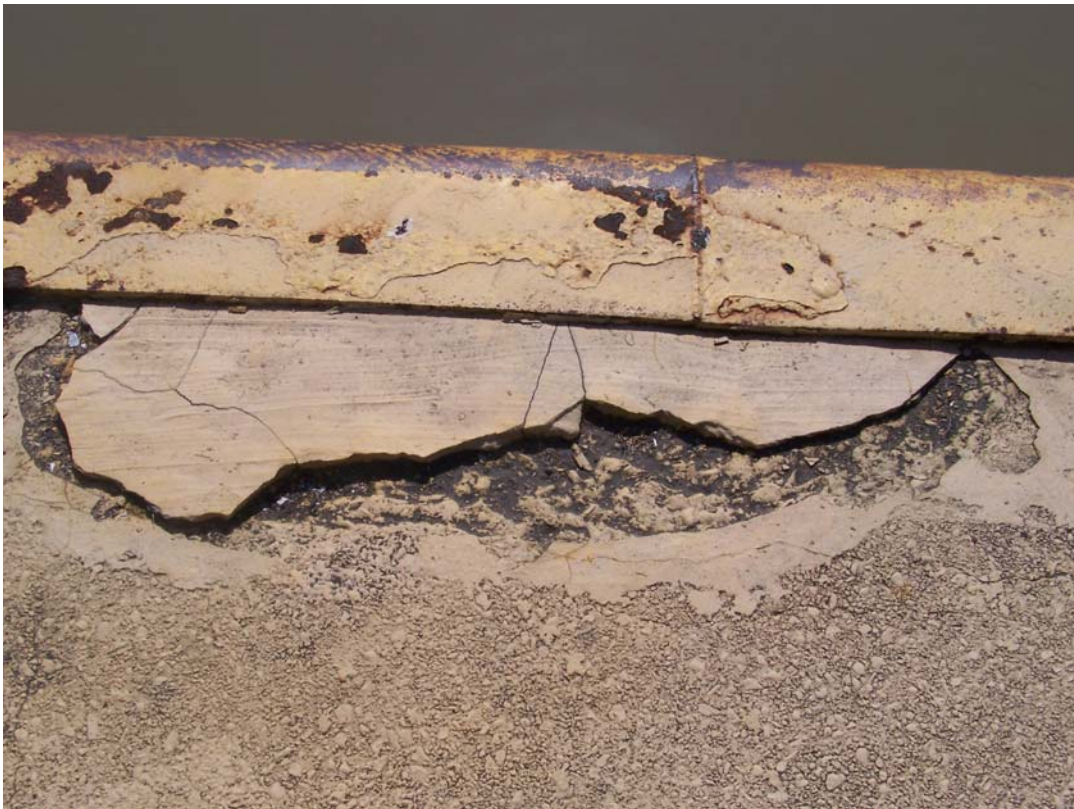
Photo 26 Large shallow spall with a failing patch in top of west chamber wall.
