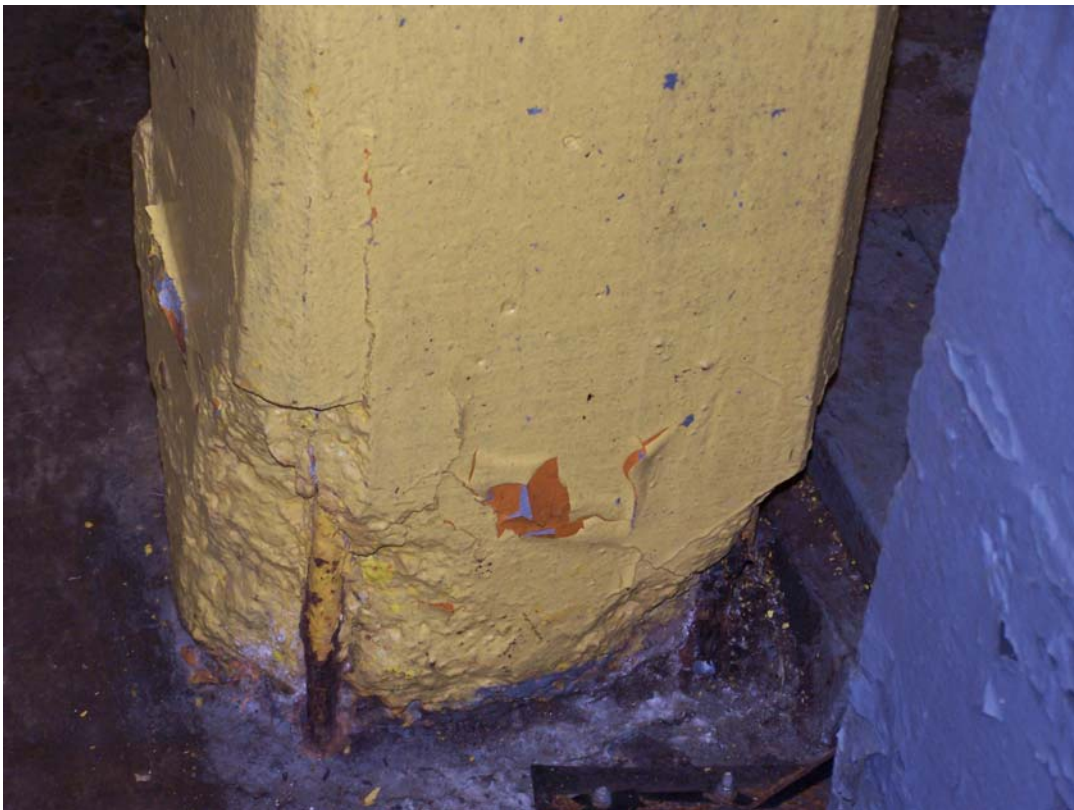
Photo 112 Spalling and corroded steel at the bottom of the column near the louvers by the hinge of gate 5. Damage to about 20" up from floor.
